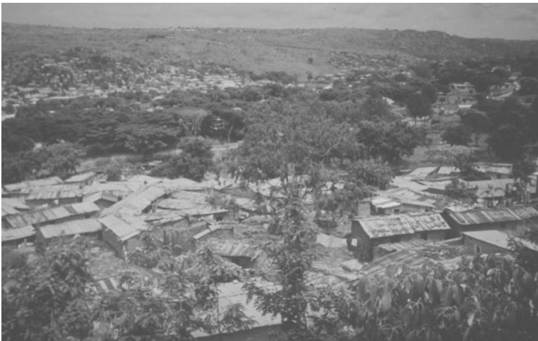
Figure 4.4 Low-income and squatter housing on the hills just above Mwanza's city center. Many of these homes are constructed with mud bricks that disintegrate easily in heavy rains and makeshift corrugated iron roofs weighed down with bricks and rocks. Pieces of corrugated iron posed an occasional but lethal threat during wind storms in Mwanza when they blew off these types of houses.
