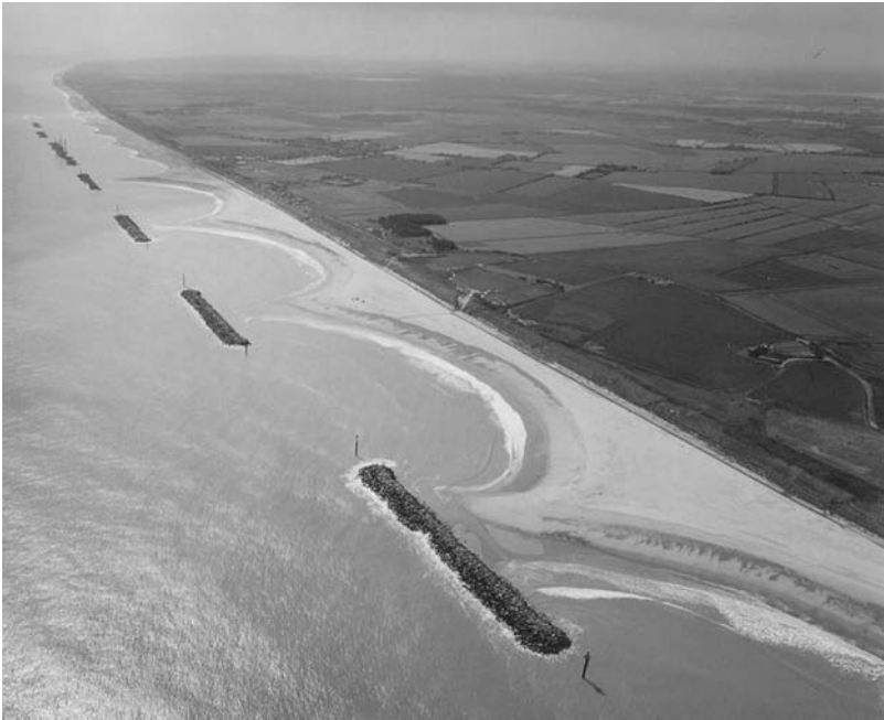
Figure 6.48 Oblique aerial photo of the Happisburgh to Winterton scheme, viewing south-eastwards (with courtesy of Mike Page).
