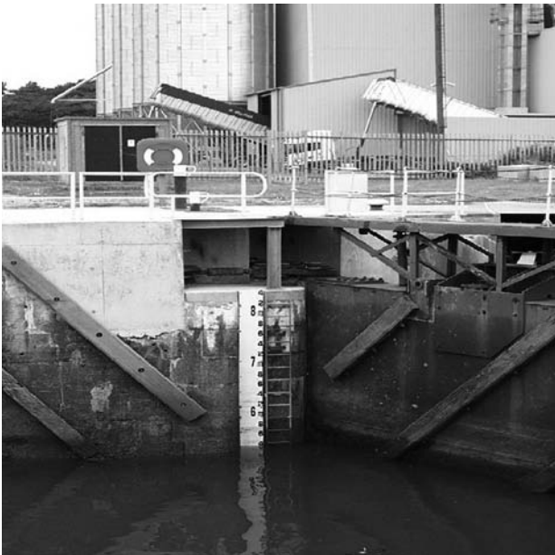
Figure 2.7 Tide boards either side of lock gates at Silloth, UK, used for recording water levels. This board, plus another on the other side of the lock gate, were the first metric boards to be installed in the UK. (Photograph courtesy of Dr Dominic Hames.)
