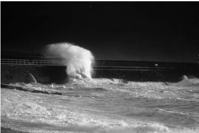
Figure 6.14 Wave overtopping of a stone/concrete near-vertical seawall at Aberystwyth, Wales. Note also the return flow of the overtopped water through the pipe outflow in the wall towards the left-hand end of the picture (photograph courtesy of Dr Adrián Pedrozo-Acuña).
