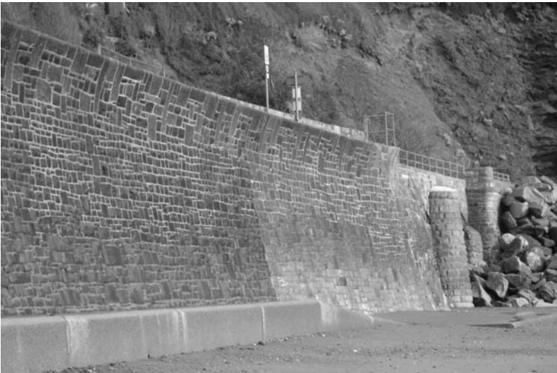
Figure 7.8 Completed repairs of the Teignmouth–Dawlish seawall (courtesy of Network Rail).
