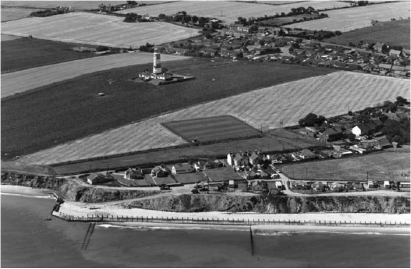
Figure 6.35 Rapidly eroding cliffs at Happisburgh, North Norfolk, UK. In the foreground the remains of a timber coast protection can be seen. The centre of Happisburgh village can be seen at the top of the photograph and the Happisburgh lighthouse towards the top left. The photograph was taken in summer 1998. The row of houses at the top of the cliffs and the three houses lying closest to the sea along the road running diagonally from bottom left to middle right have all now been lost to erosion (Photograph courtesy of Mike Page).
