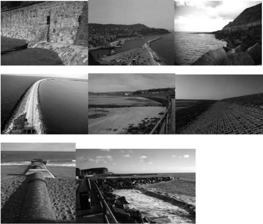
Figure 4.1 Examples of flood defence structures (left to right and from top to bottom): (a) Storm water outflow from seawall at Teignmouth, UK. (b) Harbour breakwater at Nice, France. (c) Concrete sea wall with rock scour protection at Sheringham, Norfolk, UK. (d) Harbour breakwater at Sohar, Oman (courtesy of Halcrow Group Ltd). (e) Low-lying rock groyne on a sandy beach backed by vertical blockwork wall in Colwyn Bay, Wales. (f) Concrete mattress revetment on earth embankment at Freiston, Lincolnshire, UK. (g) Short piped sea outfall at Teignmouth, UK. (h) Sea wall with rock toe protection and short groyne at West Bay, UK (courtesy of Dr David Simmonds).
