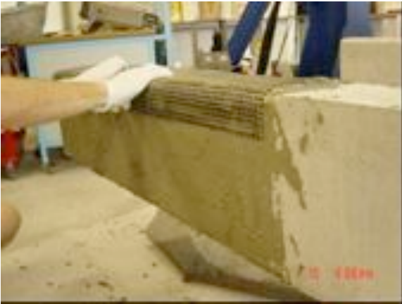
Fig. 14: Textile-reinforced mortar (TRM) jacketing.
