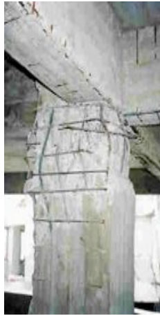
Fig. 14: Failure of a column in Adapazari due to inadequate detailing of transverse bars
