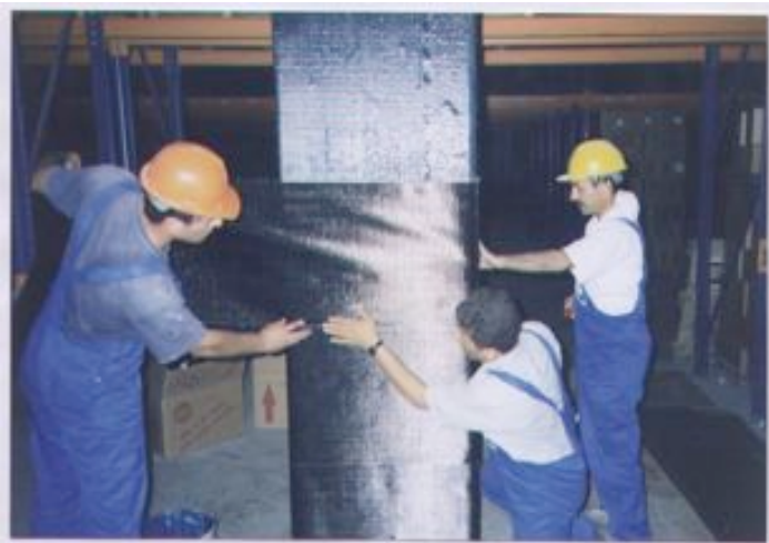
Fig. 2: FRP wrapping of a column for shear strength enhancement
