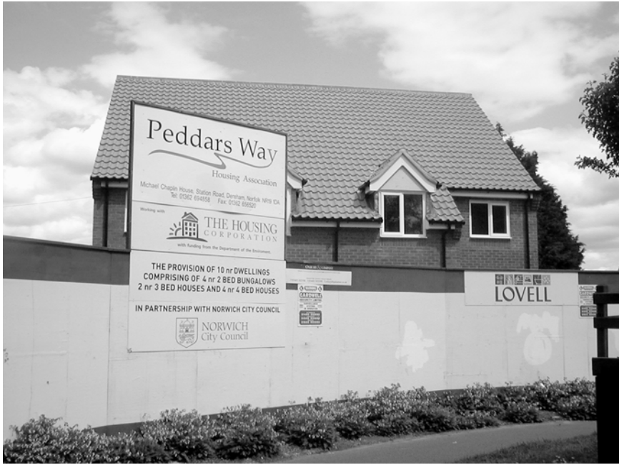
Plate 5.4 New social housing in Regeneration area, Norwich.
