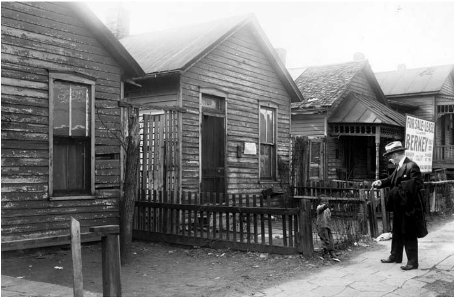
Many African Americans in Kansas City lived in subpar housing. These homes sat in the 1700 block of Troost Avenue. Courtesy of Kansas City Public Library, Missouri Valley Room.
