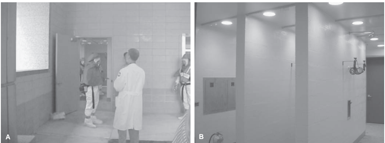
FIGURE 7.6 A fixed, indoor decontamination facility, contiguous with, but structurally separate from the main ED. A: The external entrance to the ambulance bay. B: Three parallel lanes to provide capacity for both ambulatory and nonambulatory victims. (Courtesy of Tony Van Dyke and Michael Goldberg, Department of Environmental Health and Safety, Children’s Hospital of Philadelphia, Philadelphia, PA.)
