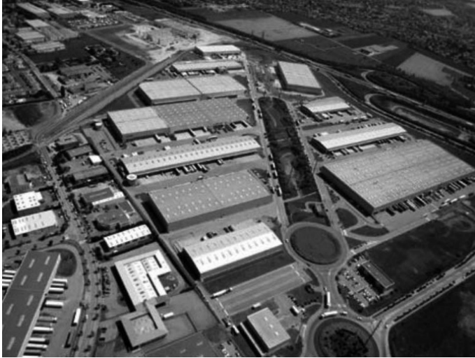
Figure 4.19. Example of a logistics area [RUL 10]
