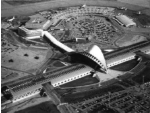
Figure 4.13. We can improve into : Intermodal road/rail/air hub for long-distance travel : airport and TGV station at Lyon-Saint Exupéry, France (Ref. CCI Lyon)
