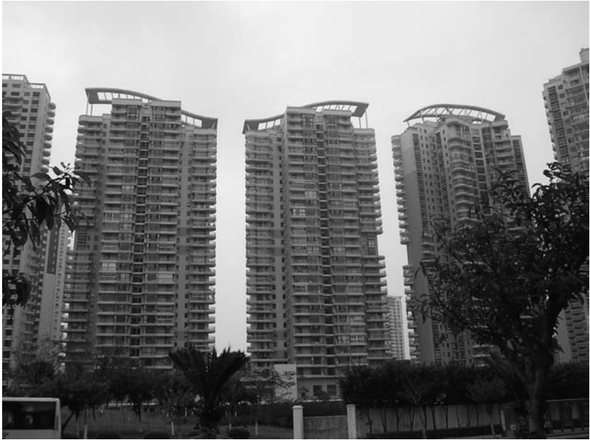
Fig 6.3 Feng shui-inspired, waving rooftop design on new apartment buildings in Xiamen, China. Photograph by Ole Bruun.
