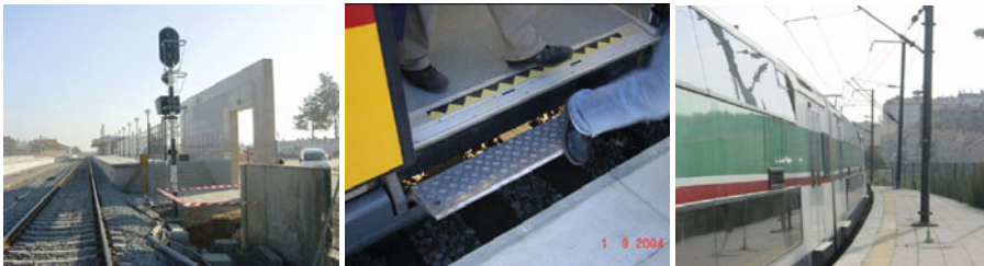
Figure 3: Gaps between the vehicle exit and the station platforms
