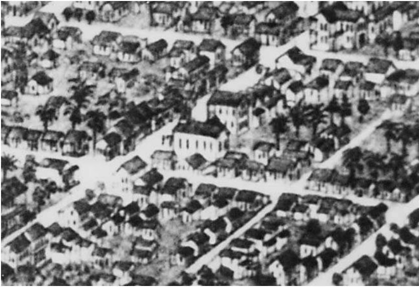
41. This view illustrates the appearance of Key West's Bethel AME Church during the 1880s. Courtesy Photographic Collection, Florida State Archives, Neg. No. 421.
