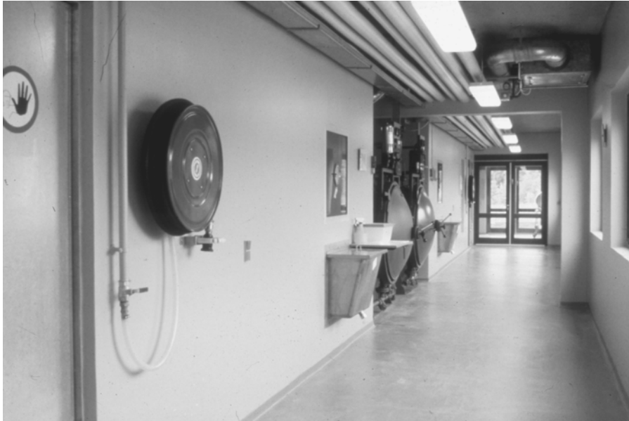
Figure 11.6 The outside of two separated barrier units. The shower entrance of barrier 1 is closest followed by a diptank for chemical disinfection into barrier 1, autoclave for barrier 1, autoclave for barrier 2, diptank for barrier 1, shower entrance and chemical disinfection lock for barrier 2 (M&B Ltd, Denmark).
