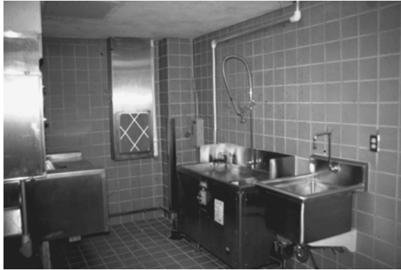
Figure 8.5 From the view of the soiled side of a cage sanitation facility, shown is a bedding dump and disposal station that disposes of bedding directly to the sanitary sewer system. To the left of the picture is the load end of a tunnel washer. To the near side of the disposal unit is a wall-mounted stainless steel sink typical of a type often recommended for use in animal rooms. The wall and floor finish is ceramic tile with epoxy grout.
