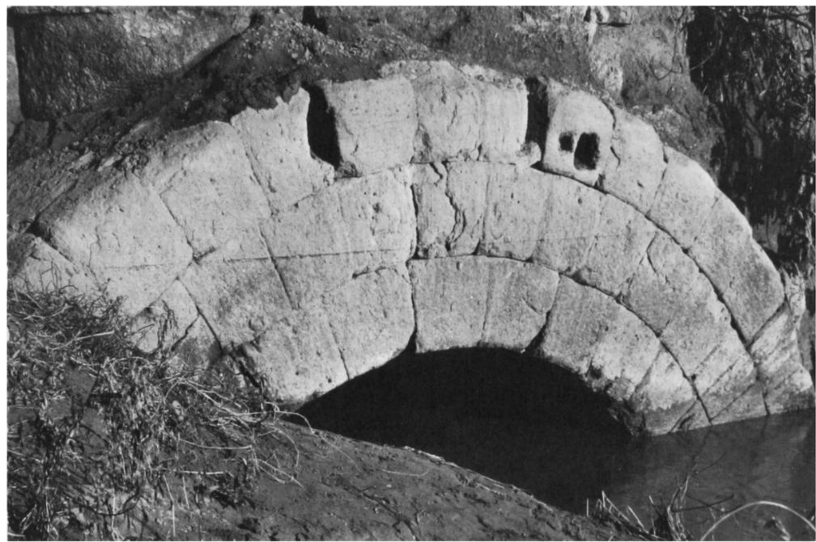
100. Cloaca Maxima : its issue into the Tiber. The masonry, once considered part of the original construction, is now dated to the second century B.C. though of course the drainage channel is much earlier
