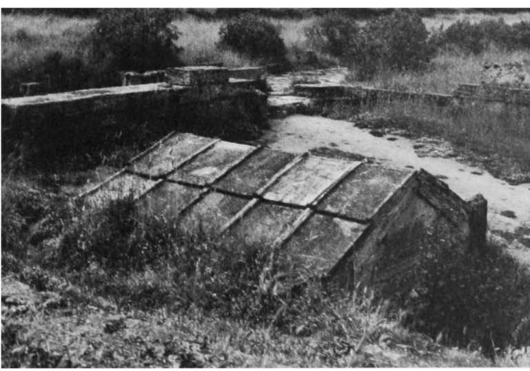
141. The 'buried' shrine at Paestum from S.-E. showing the blocked 'entrance'
