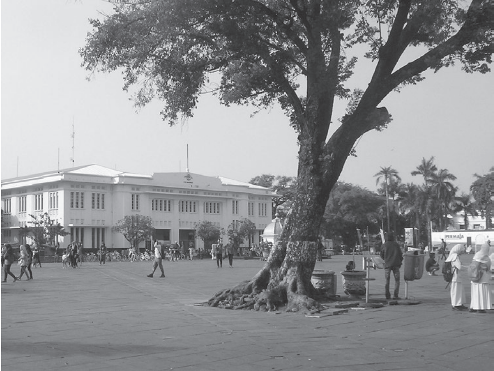
Figure 2.3 An example of Dutch colonial modernism in Indonesia (photograph by Freek Colombijn)
