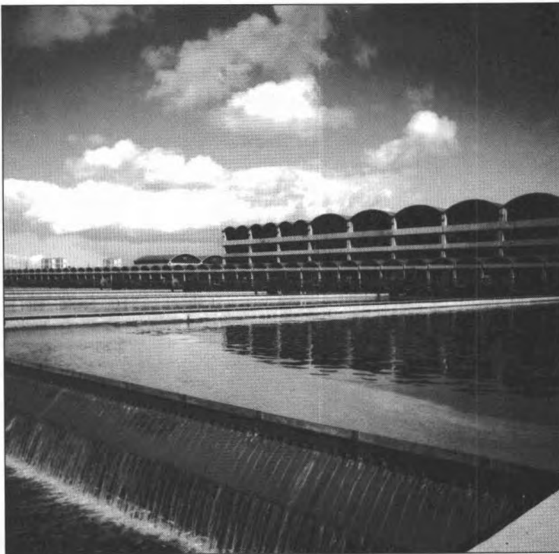
Sheildhall sewage works, Glasgow, Scotland for Strathclyde Regional Council.
