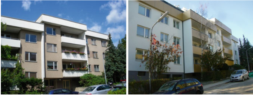
Fig. 9 V_RES_BOKU2 before renovation ( left ), and after renovation ( right ) (Heidenreich 2014, 2015)
