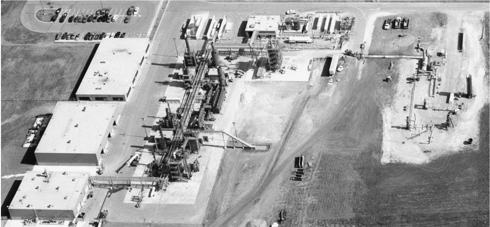
FIGURE 9.1 John Zink Co. LLC. R&D Test Center, Tulsa, Oklahoma. (Courtesy of John Zink Co., LLC. 21 )
