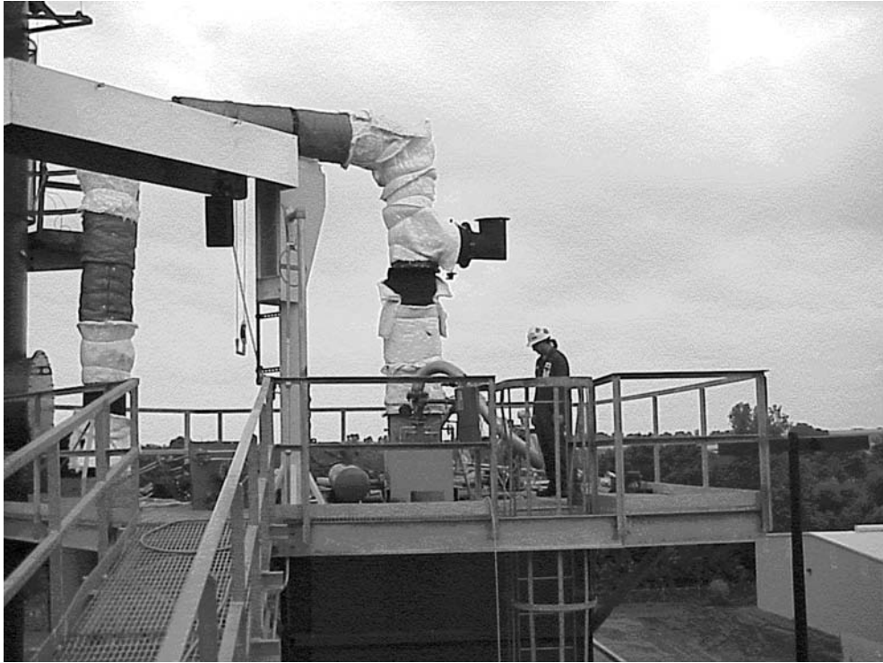
FIGURE 6.37 Example of a down-fired, forced-draft, preheated air burner. (Courtesy of John Zink Co., LLC. 3 )
