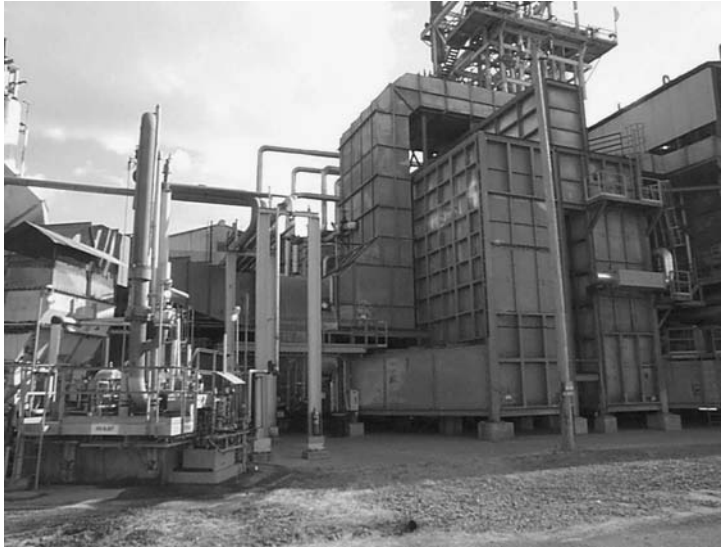
FIGURE 16.15 Cabin heater. (Courtesy of John Zink Co., LLC. 3 )
