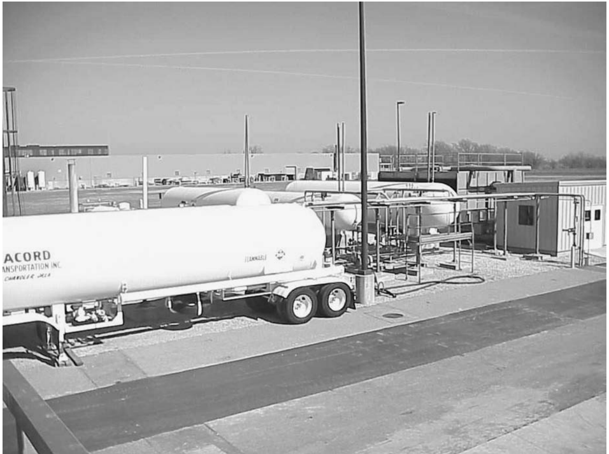
FIGURE 9.6 Test fuel storage tanks. (Courtesy of John Zink Co., LLC. 21 )
