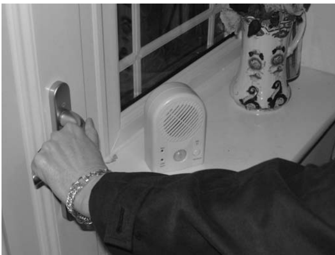
Figure 8 A wander reminder fitted near an exit door
