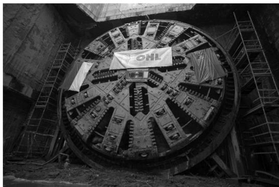
Figure 8. Breakthrough of S-745 Słowacki Tunnel Gdansk.
