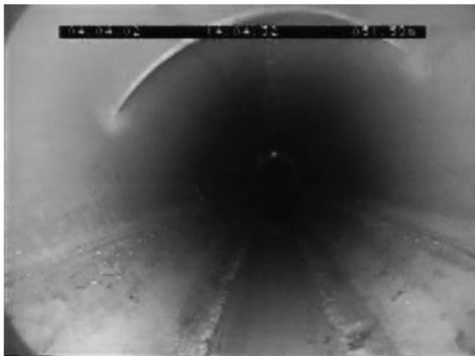
Figure 5. Linear dent in the PVC-U pipe (photograph by the author).
