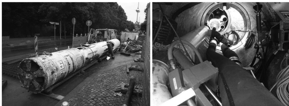
Figure 9. Assembly of the AVN slurry machine and jet pump in machine can 3.
