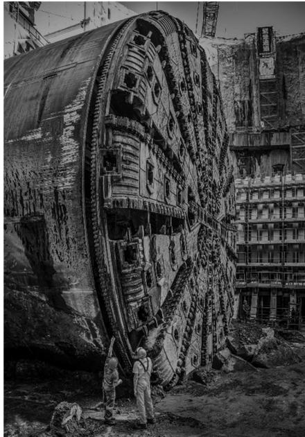
Figure 6. Breakthrough of the 17.6 m diameter Mixshield.
