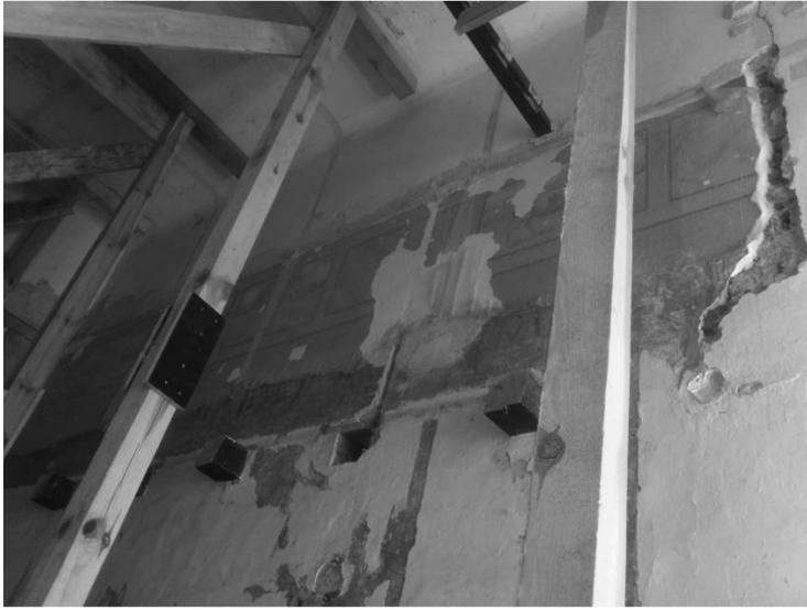
Figure 2. Historic wall paintings in the building of the former House of Prayers. Visible temporary protection of the ceiling with a wooden structure.
