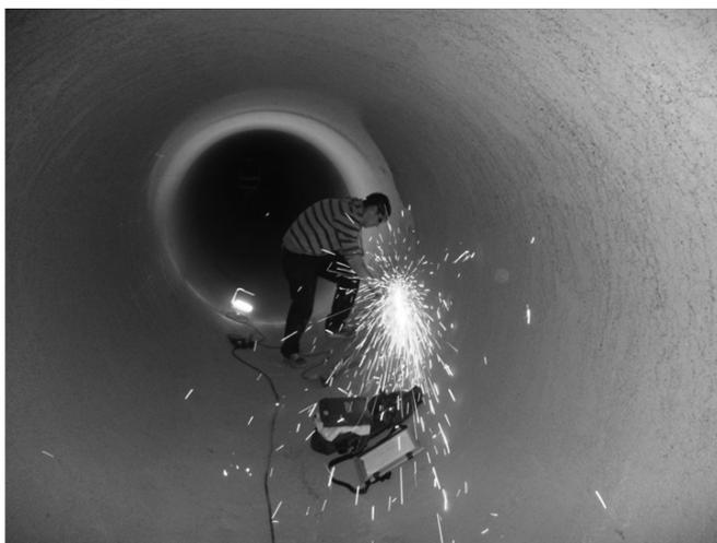
Figure 4. Preparation of a surface for measurements [Abel, 2016].
