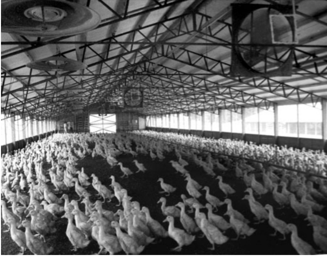
Fig. 3.15. Naturally ventilated intensive rearing accommodation provided with large-diameter fans used to distribute a microsol of water and reduce environmental temperature.
