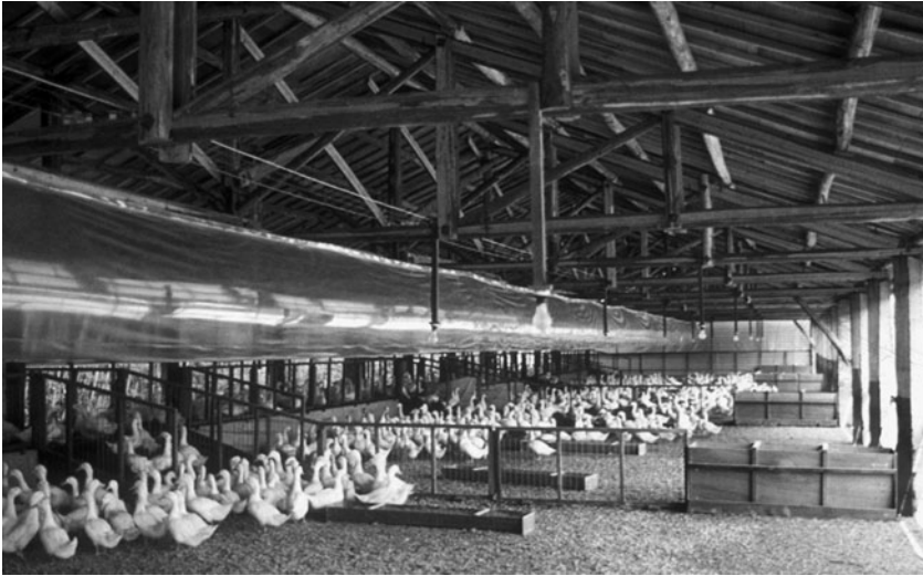
Fig. 3.16. Naturally ventilated intensive breeding accommodation provided with pressure jets to distribute a microsol of water to reduce environmental temperature.
