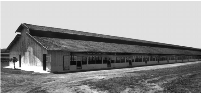
Fig. 3.14. Naturally ventilated intensive duck-rearing accommodation.
