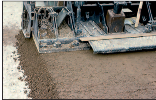
Figure 23 Paver-laying of mix-in-plant produced HBM.
