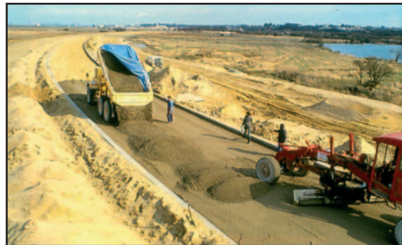
Figure 19 Sheeted-lorry delivering mix-in-plant produced HBM for grader-laying. Note how discharge is carried out 'on-the-run' to minimise segregation and aid spreading.
