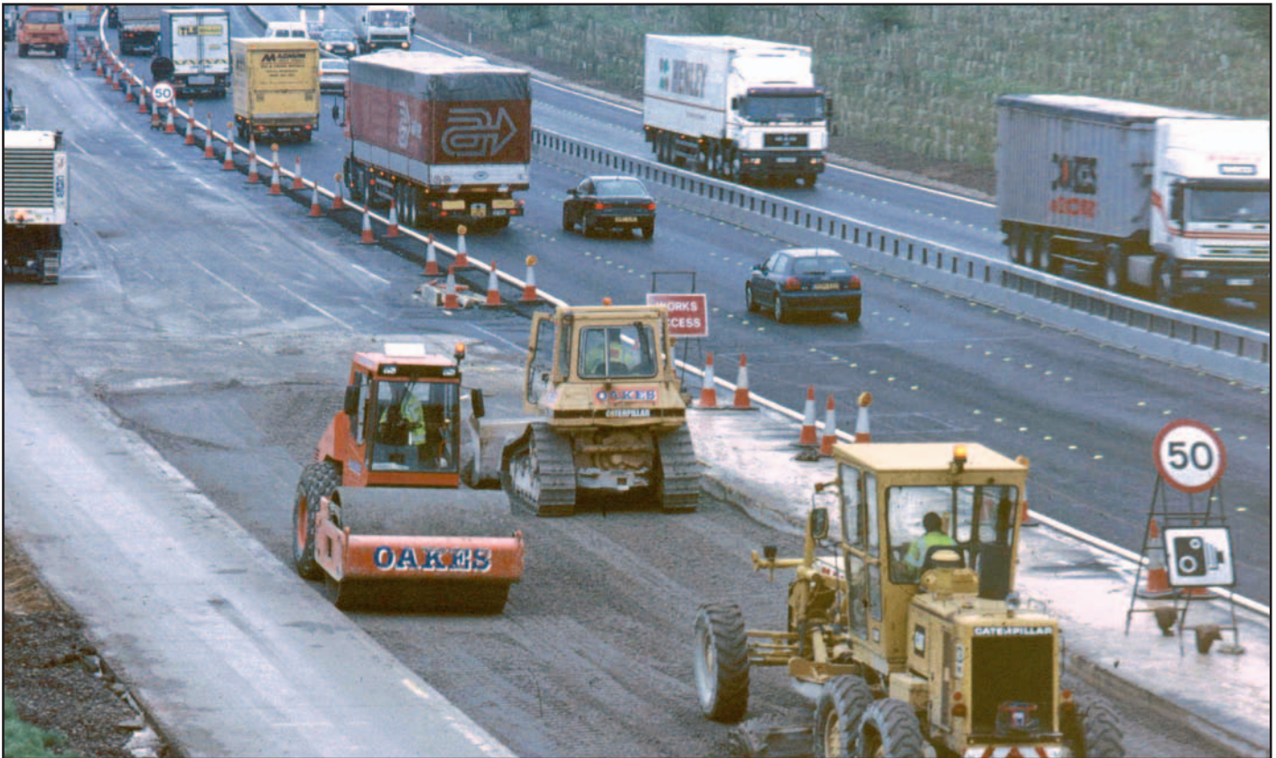
Figure 3 Grader laying and compaction of mix-in-plant produced HBM.
