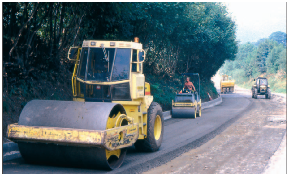
Figure 26 Compaction plant – vibrating roller.
