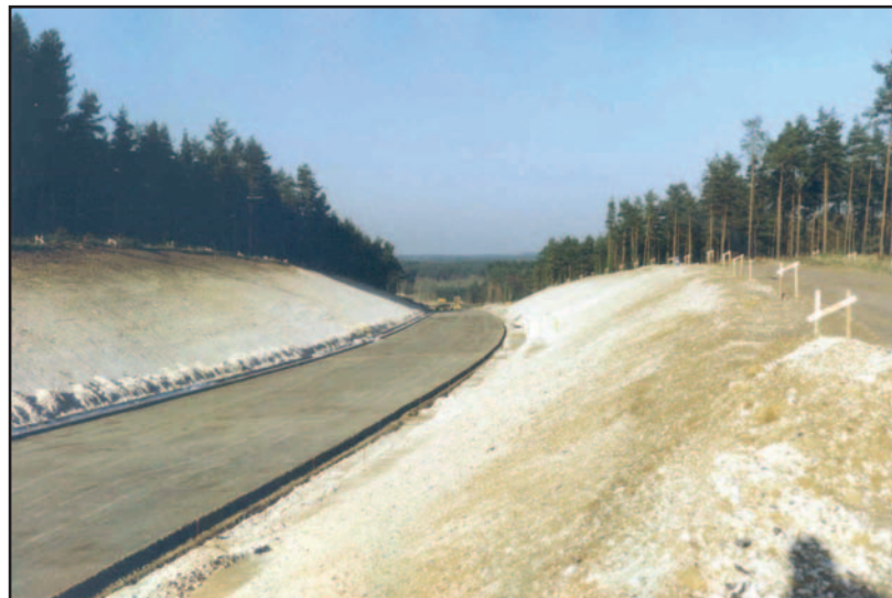
Figure 4 Completed HBM layer with an aluminised resin-based seal coat.
