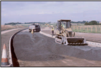
Above: Figure 20 Dozer-spreading of mix-in-plant produced HBM.
