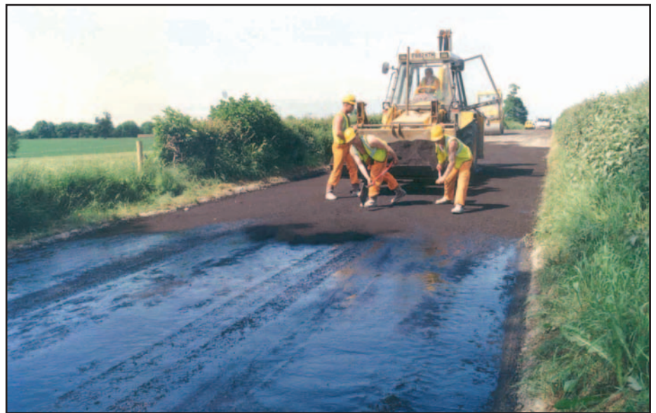
Figure 30 Application of grit to prevent removal of bitumen-emulsion seal coat under traffic.
