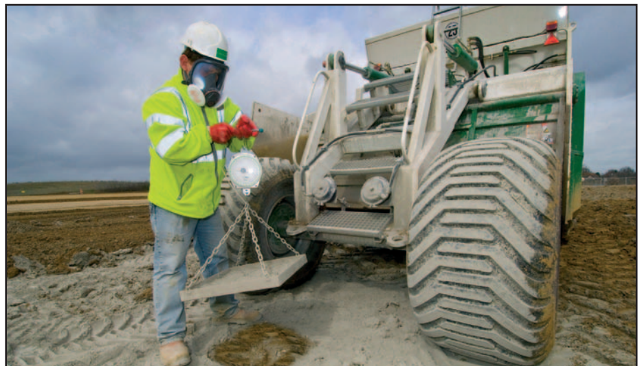
Figure 31 Checking 'rate-of-spread' of powder with mix-in-place work. The powder-spreader has passed over a tray of known area and weight
