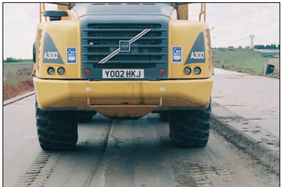
Figure 5 Fresh HBM under site traffic.
