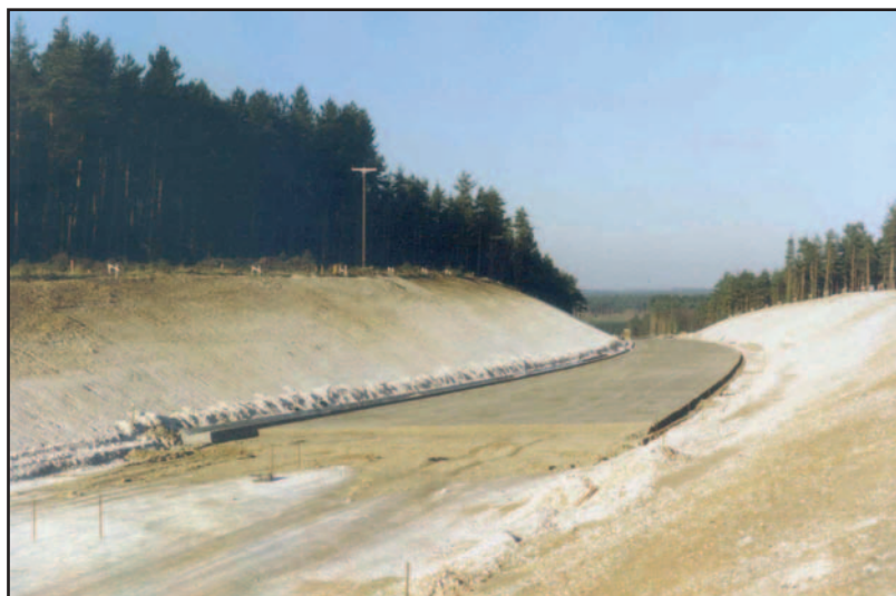
Figure 24 End-of-day shot of paver-laid material, cut-back to a vertical-face of fully-compacted material in preparation for next day's laying. Previously the end of the layer had been 'ramped-down' by the rollers during compaction.
