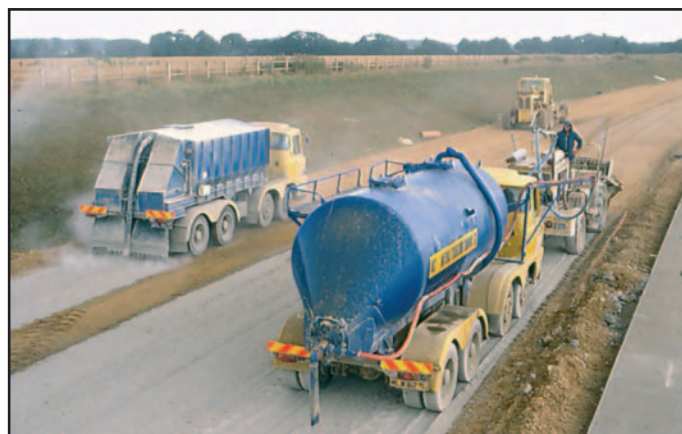
Figure 14 Mix-in-place method of construction showing powder spreading and water-bowser in tandem with rotovator for water addition through spray-bar in hood of rotovator.
