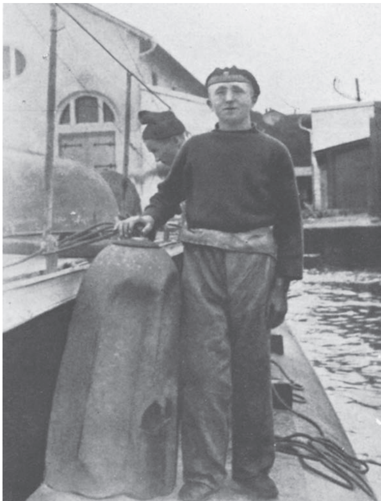
Fig. 13. A torpedo head crushed by depth charges
