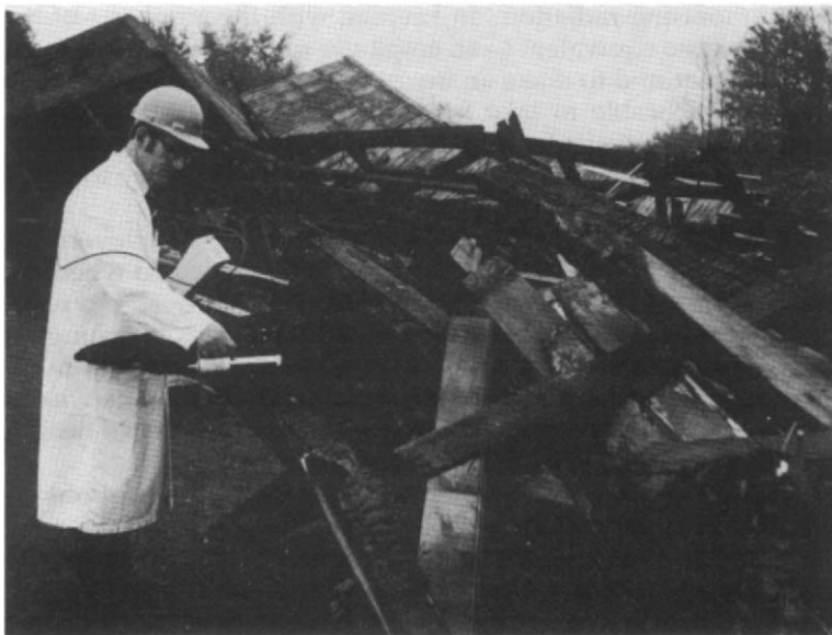
Figure 4.3 Checking contamination levels after a fire
