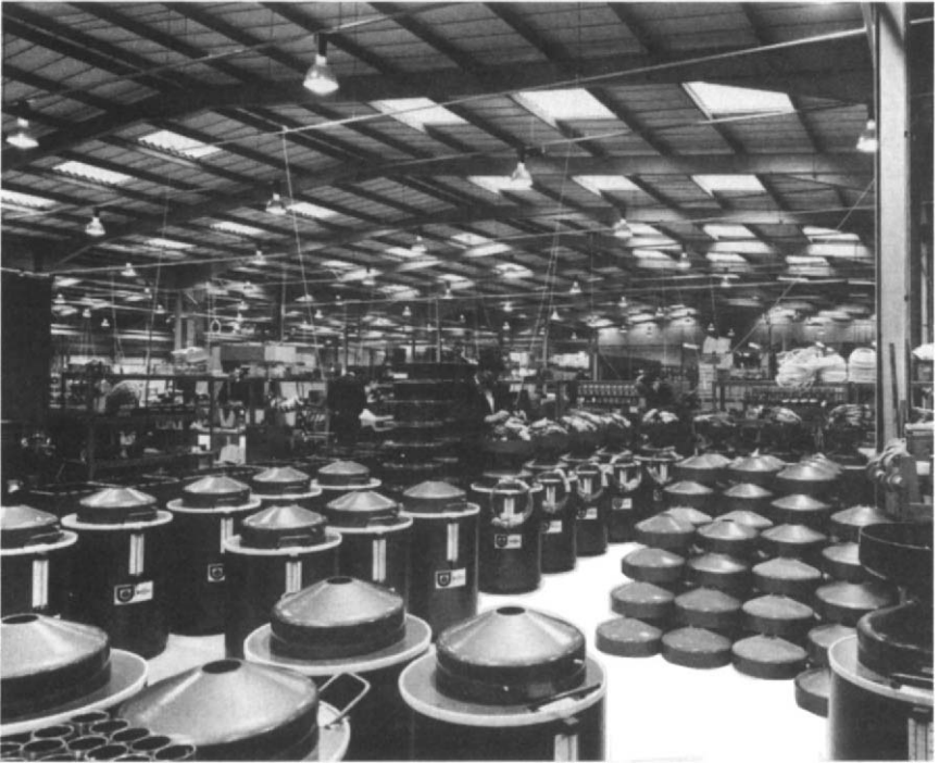
Figure 7.2 Factory lighting of correct illuminance, free from shadow and glare, making use of high pressure discharge lamps. (Courtesy Thorn Lighting Ltd)
