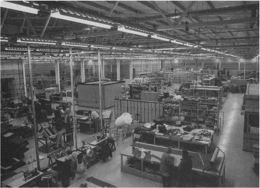
Figure 7.1 Factory lighting where fine work is carried out and colour rendering is important, making use of reflector luminaires with tubular fluorescent lamps. (Courtesy Lighting Industry Federation)
