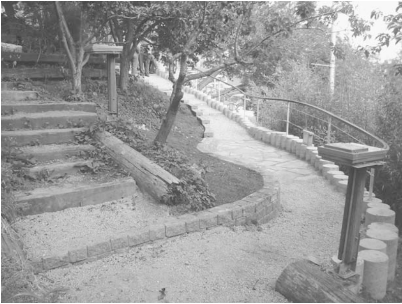
Figure 9.8 As a community-university partnership, the NDBS obtains funding from multiple sources—the university’s Howard S. Wright Endowment, local businesses, foundations, and the Seattle Department of Neighborhoods. Because students supply design and construction services as part of their professional education, these funds are devoted solely to materials. Shown here is a newly installed path from the street that provides a legally accessible route into the garden. Photographs courtesy of the UW’s Neighborhood Design/Build Studio.
