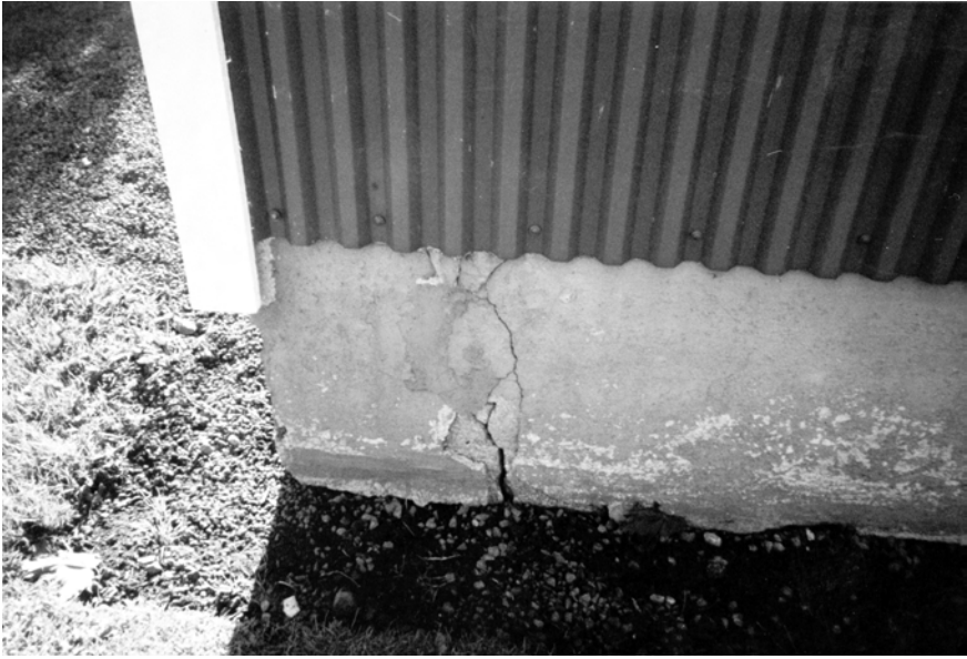
Figure 7.9 Crack in a foundation
