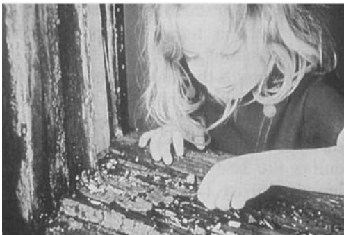
FIGURE 1-6 • Lead-based paint in many older homes still represents a serious health hazard to many young children. A. Potential child exposure to peeling lead-based paint on a windowsill, a common site for such exposure. Although the most important pathway of exposure to lead-based paint is through house dust and hand-to-mouth activity by young children, paint chips may be directly ingested, and toddlers often stand at a windowsill while chewing or sucking on the paint. B. Lead-abatement worker, with personal protective equipment, performs postabatement cleanup. Workers performing lead abatement must be trained and certified, and they must carefully adhere to safe practice standards. (Photographs by the California Department of Health Services.)
