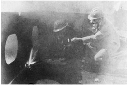
FIGURE 30-2 ● The worker at left is exposed to lead as he cuts apart a ship. The man at right is obtaining an air sample for lead determination. (Photograph courtesy of NIOSH.)
