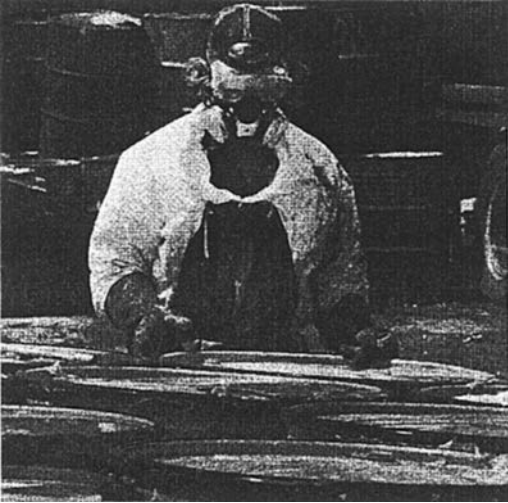
FIGURE 2-2 ● Hazardous waste worker sealing abandoned drums of waste chemicals.
