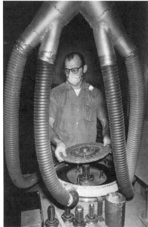
FIGURE 7-3 • Local exhaust ventilation used to protect a worker from asbestos dust generated in working with clutch plates. (Photograph by Earl Dotter.)
