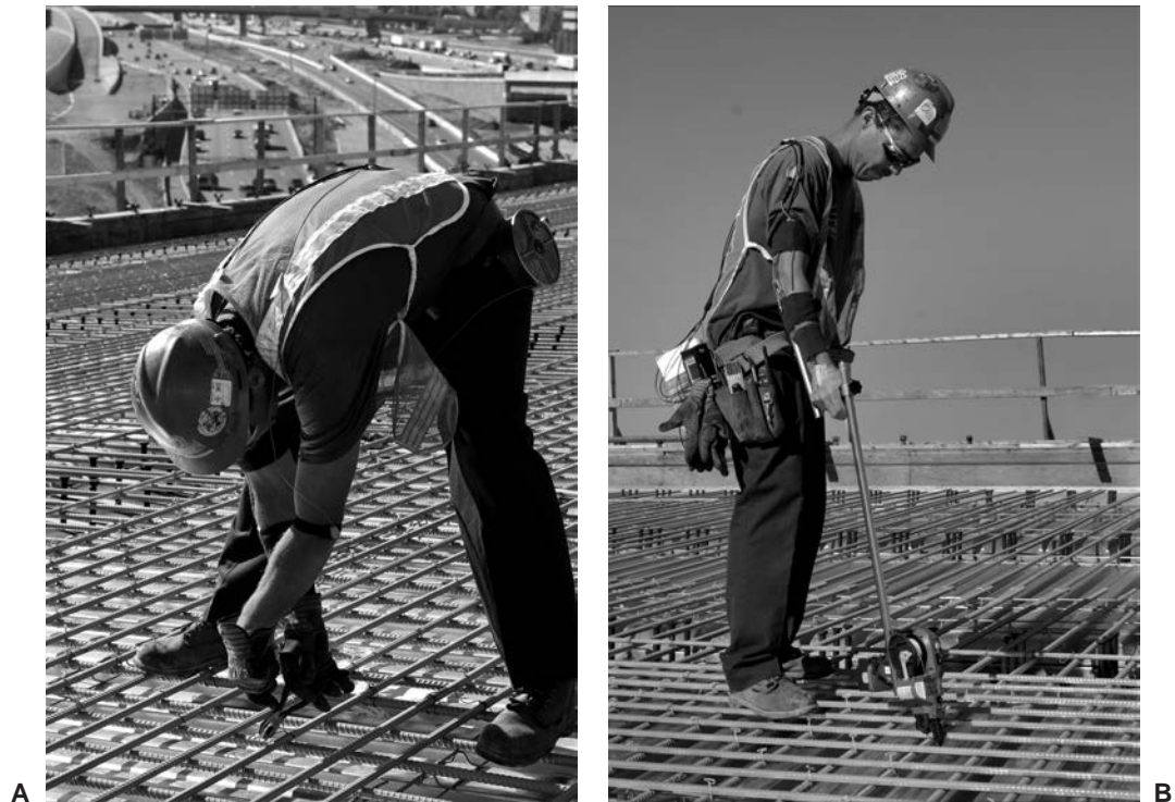
FIGURE 32-4 • (A) Construction workers are at increased risk of upper extremity and back strain. (B) An ergonomically designed device decreases the upper extremity and back strain on construction workers who are tying rebar. (Photographs by Earl Dotter.)
