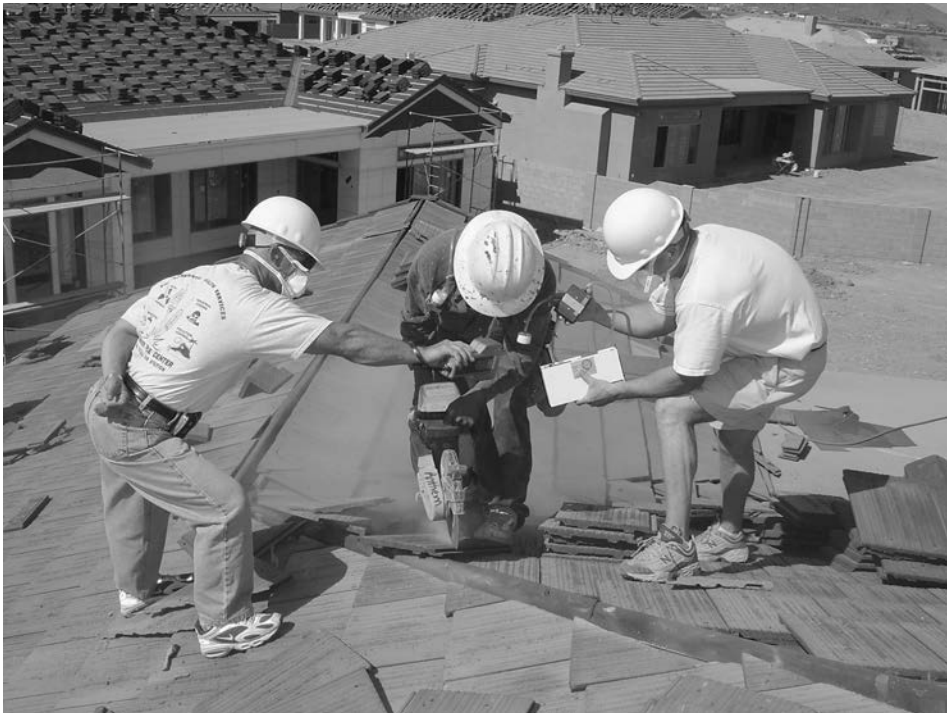
FIGURE 33-2 • Industrial hygienists collecting follow-up samples for silica exposure among roofers. (Courtesy of the National Institute for Occupational Safety and Health.)
