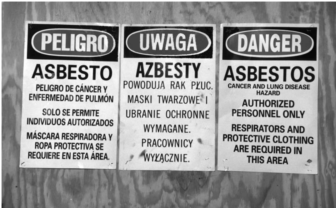
FIGURE 7-4 • Warning signs, as illustrated in this photograph, should be in multiple languages, if appropriate. (Photograph by Earl Dotter.)
