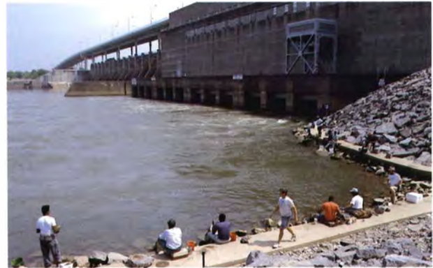
One of the numerous dams on the Tennessee River, Chickamauga Dam, Hamilton Co., TN.
