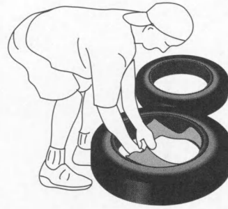
Wall framing using automobile tires.
