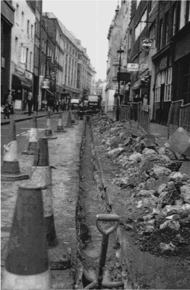
Plate 16 The SohoNet under construction in the Soho district of London, a centre of media activity. Source: SohoNet Web page www.sohonet.co.uk
