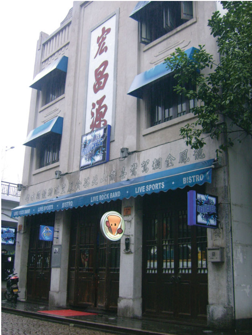
Fig. 4.1 The Hongchangyuan building after renovation (photographed by the author in March 2009).
