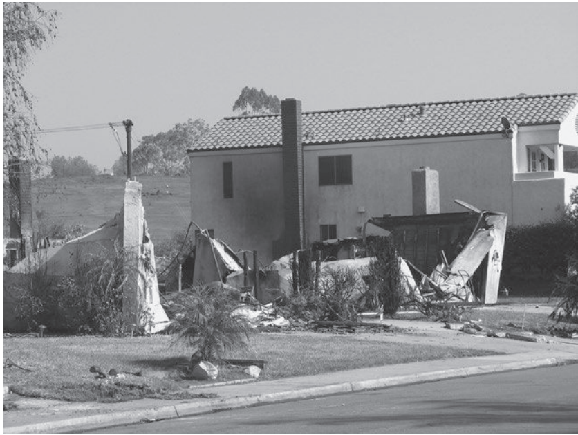
Figure 3.2 Lack of Planning for Wildfires: Home Burned in the Rancho Bernardo Community of San Diego
