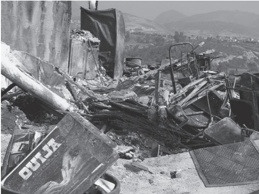
Figure 6.1 Home Damaged by 2007 Wildfire, Rancho Sante Fe Suburb of San Diego
