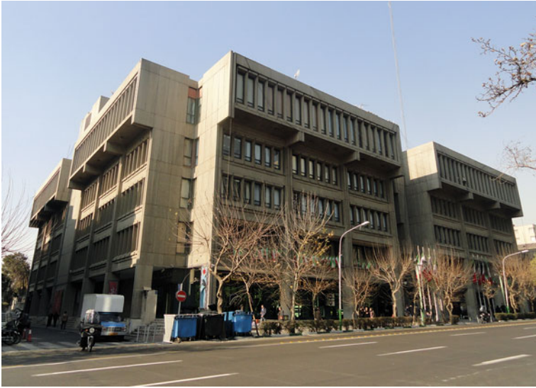
Fig. 3.15 Behshahr Headquarter, general view (Author)
