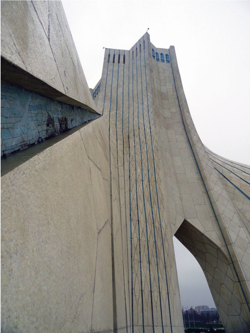
Fig. 3.9 Azadi Tower, façade (Author)
