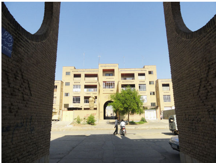
Fig. 4.4 Shushtar-No, view to apartment housing (Author)
