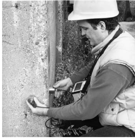
FIGURE 8.6 Application of pulse velocity technique on a concrete structure. (Courtesy of James Instruments, Inc.)
