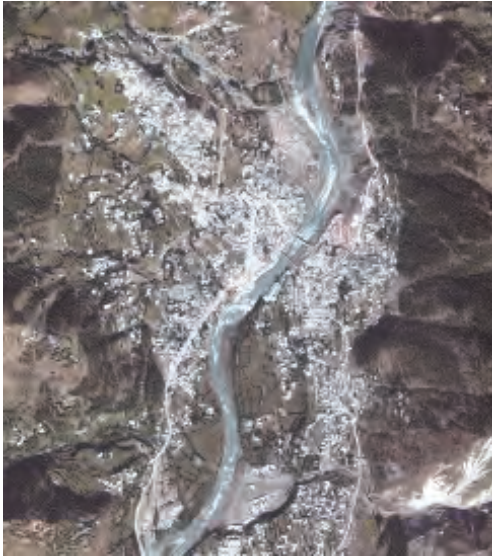
Figure 29.2 Satellite image showing destruction of a bridge as a result of flooding.
