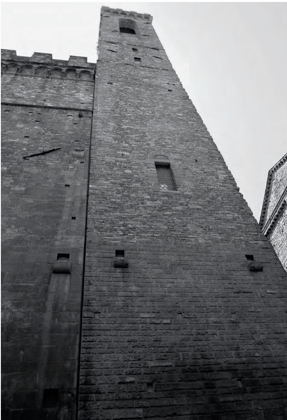
FIG. 86 The bell tower of the Podestà (Bargello), where the separate structures of tower and palace can easily be distinguished by both the color of the stones and the ways in which they have been dressed by the stonecutters. Photo by author.
