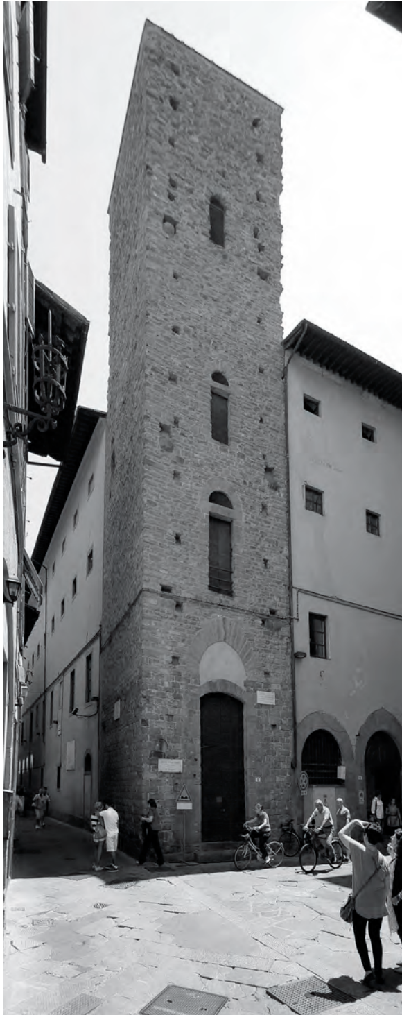
FIG. 79 Torre della Castagna: the mute façade of the old defensive towers that protected the tower societies of medieval Florence and that fell under strict regulation with the establishment of the Florentine Republic and its Ordinances of Justice. Councils of the secondo popolo met here before the completion of the Palazzo Vecchio. Photo by author.
