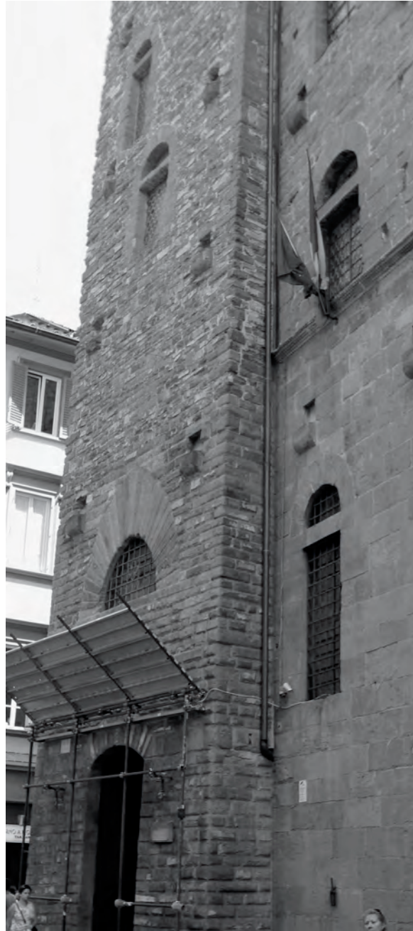
FIG. 88 The Bargello, showing the distinct axes and masonry techniques for the twelfth-century bell tower ( left ) and the thirteenth-century palace ( right ). Photo by author.
