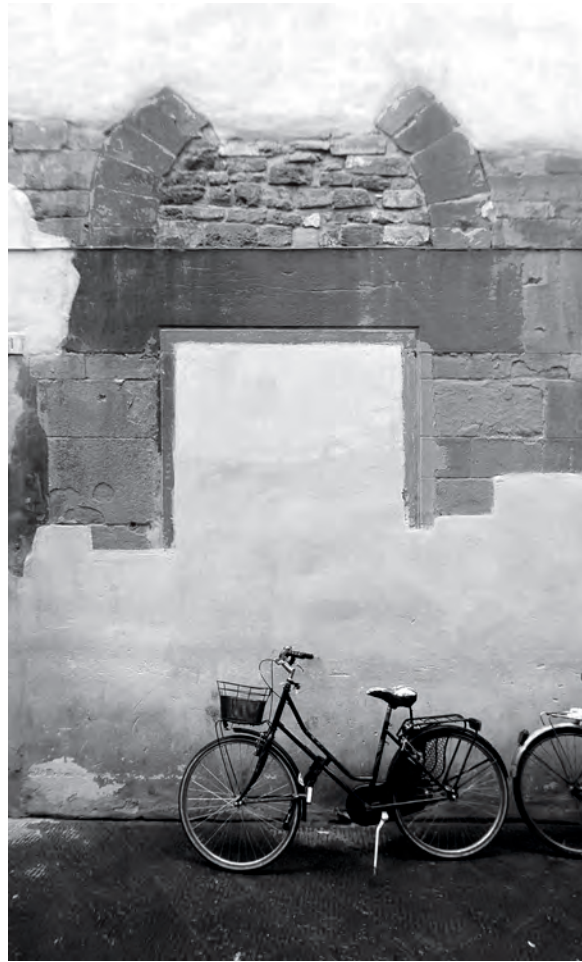
FIG. 122 The remains of the old portal of San Martino before the church was reoriented. Photo by author.
