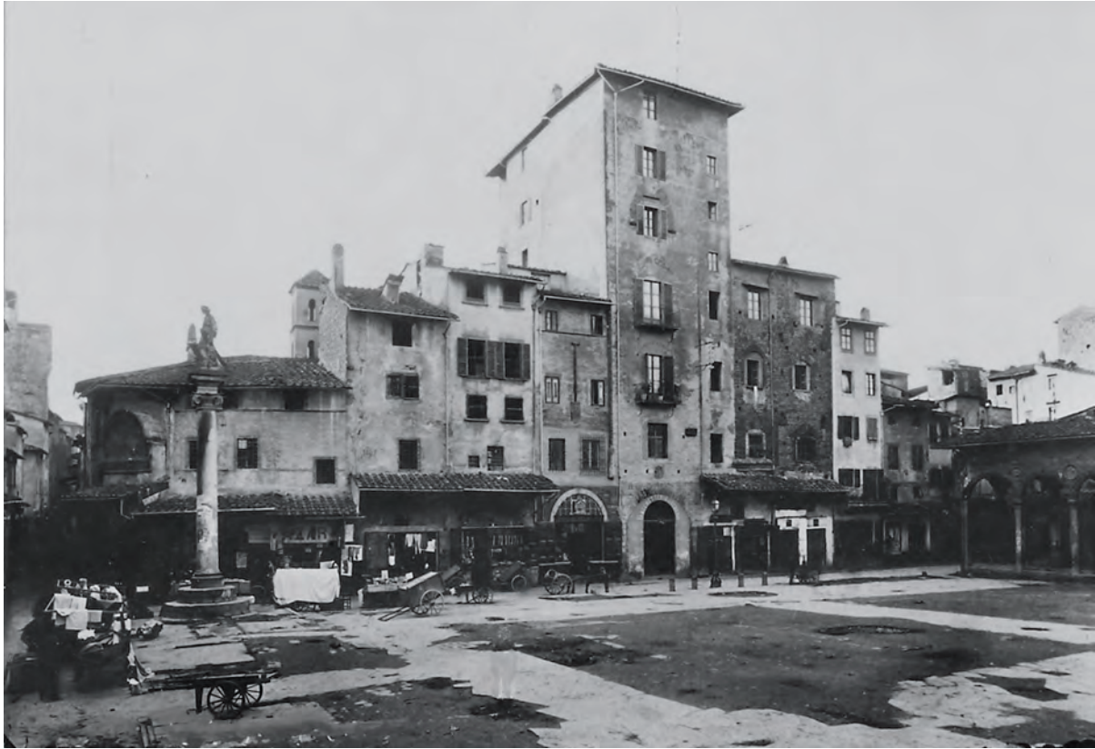
FIG. 22 Piazza del Mercato Vecchio, c. 1890, during the demolitions that would transform it into the present Piazza della Repubblica. The exposed structures still give a sense of the densely packed living arrangements persisting well into the nineteenth century. Photo: Kunsthistorisches Institut in Florenz—Max-Planck-Institut.
