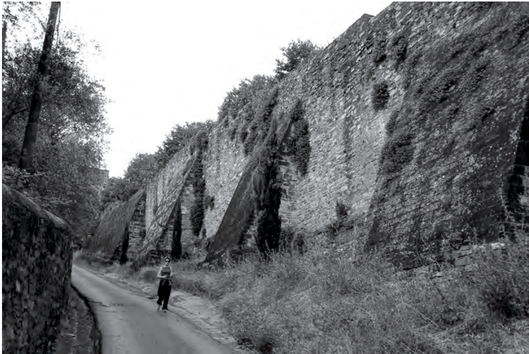
FIG. 71 View of the remaining section of the fourteenth-century walls in the Oltrarno, ascending from Porta San Miniato to the Porta San Giorgio. Photo by author.
