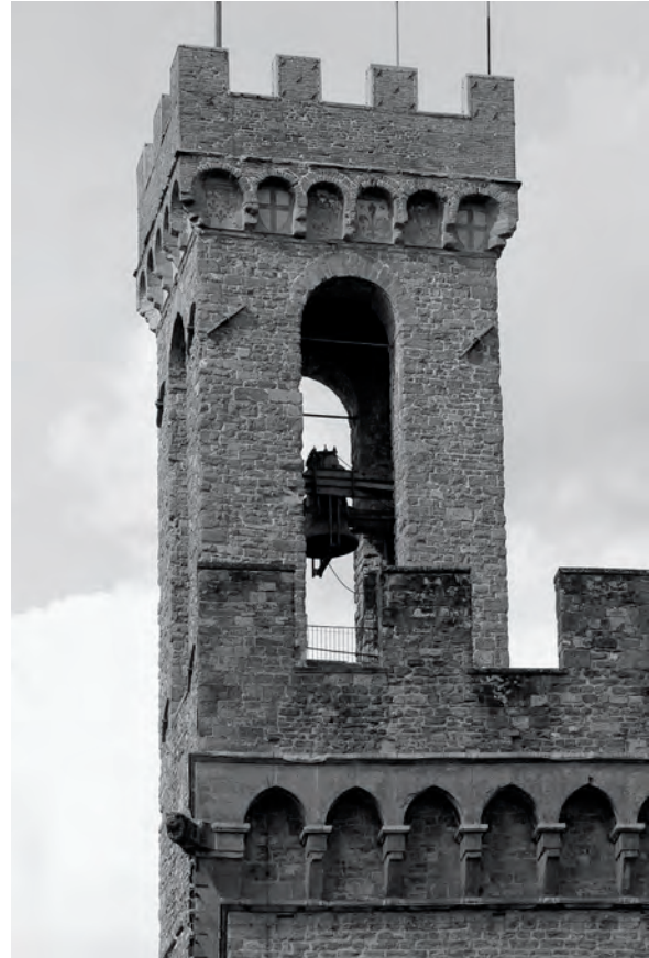
FIG. 89 View of the belfry of the Palace of the Podestà (Bargello). The corner pilasters of the crenellated summit are structural and may have allowed for the construction of a more elaborate and ornamented bell housing. Photo by author.
