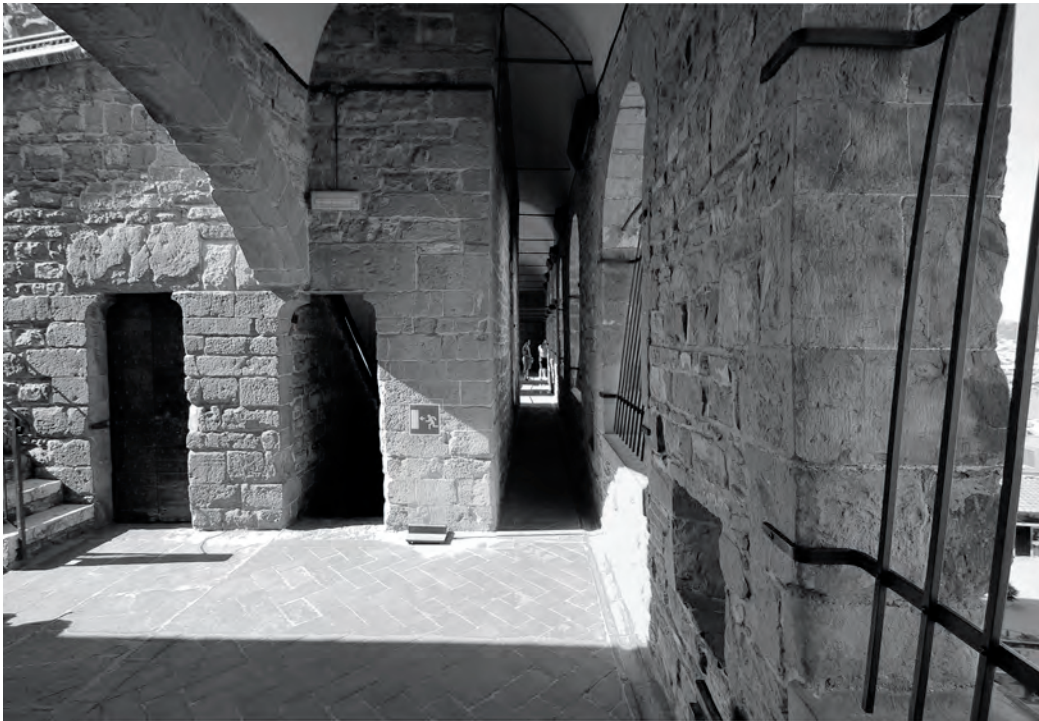
FIG. 94 View of the substructure of the bell tower of the Palazzo Vecchio (on the left with two doors) seen from the arcaded gallery. Trachtenberg has pointed out that the narrow passage on the right between the arcades and the tower makes it appear from the square that the tower is floating, when in fact the palace has been built around the preexisting tower, filling it in to support the massive belfry built above. Photo by author.
