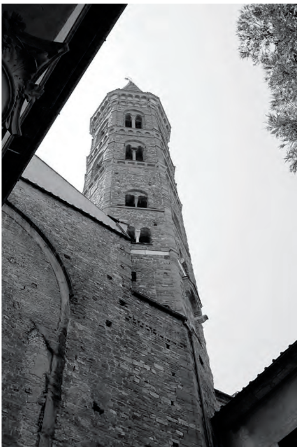
FIG. 31 New hexagonal bell tower of the Badia rising from its old foundations, reconstructed after 1330. Photo by author.
