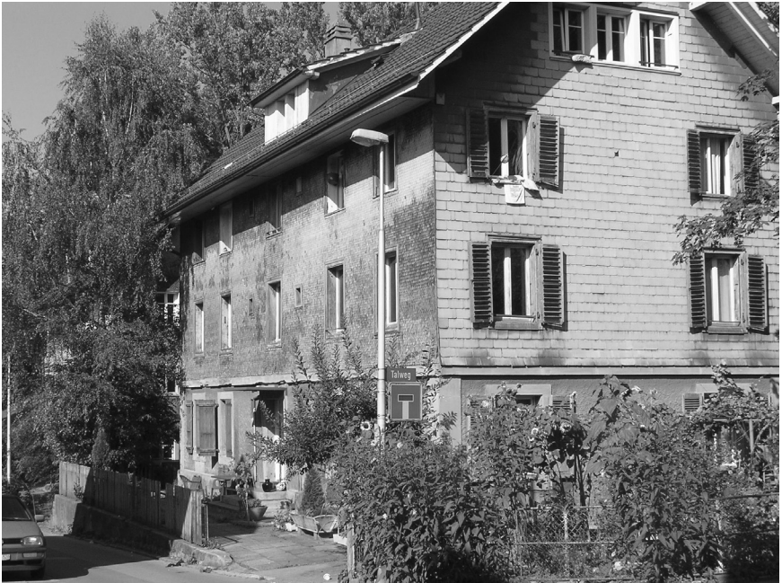
Figure 21.1 Communal housing and urban regeneration in Lorraine, Berne. Once a typical state-owned house to be demolished, this dwelling was occupied in the early 1980s, renovated step-by-step, and is today one of Lorraine's listed buildings.
