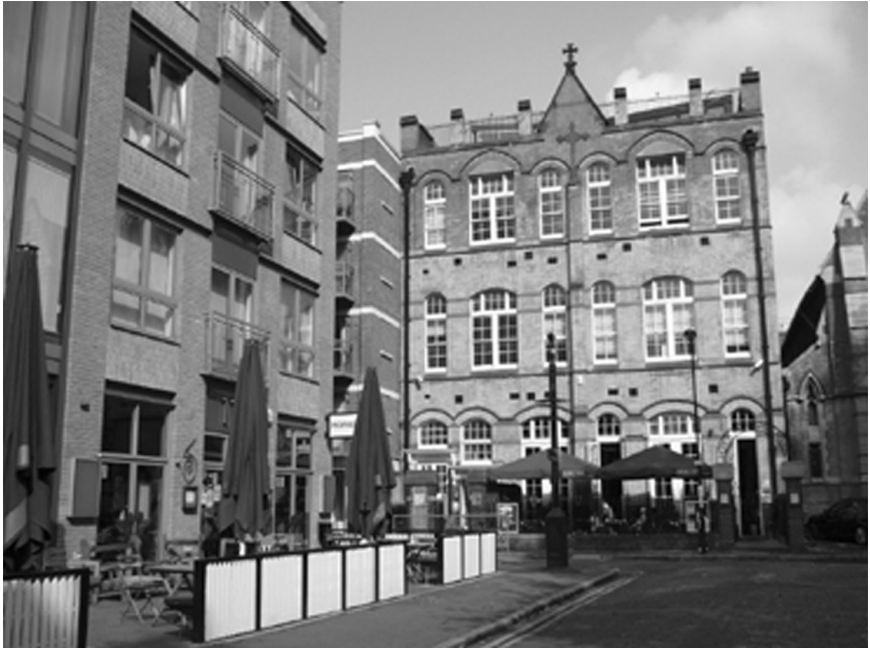
Figure 16.2 16 Hoxton Square community centre, London. Retaining spaces for local communities amidst upmarket bars and art galleries.
