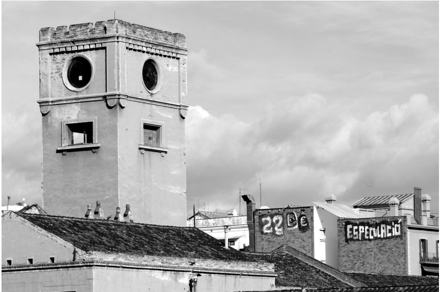
Figure 12.2 Can Ricart tower, Barcelona.
