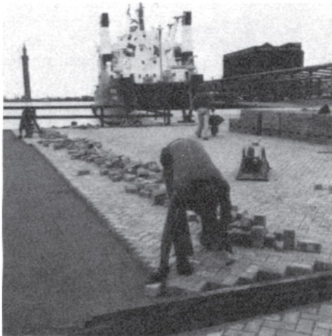
Fig. 6.20. Interlocking blocks being laid on site.
