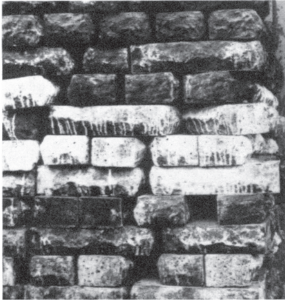
Fig. 3.1. Lime bloom masking black pigmented wet-cast blocks.
