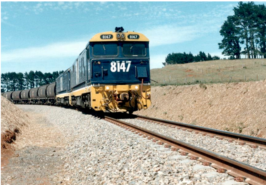
Figure 7-3: Track in Australia with Pandrol rail fastenings
