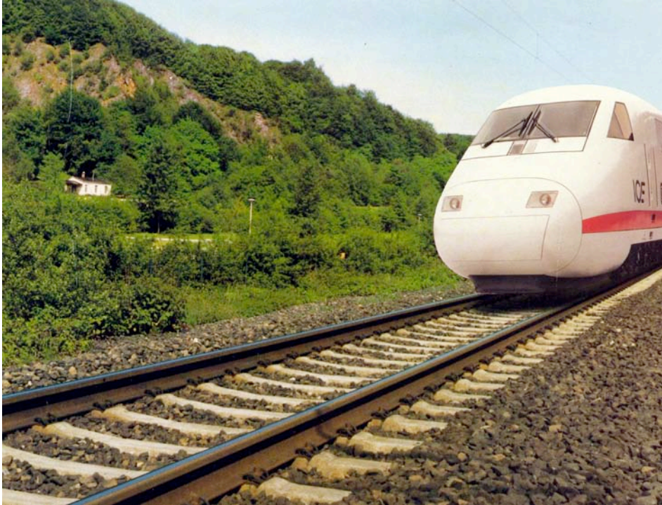
Figure 7-2: Track in Germany with Vossloh rail fastenings (2002)
