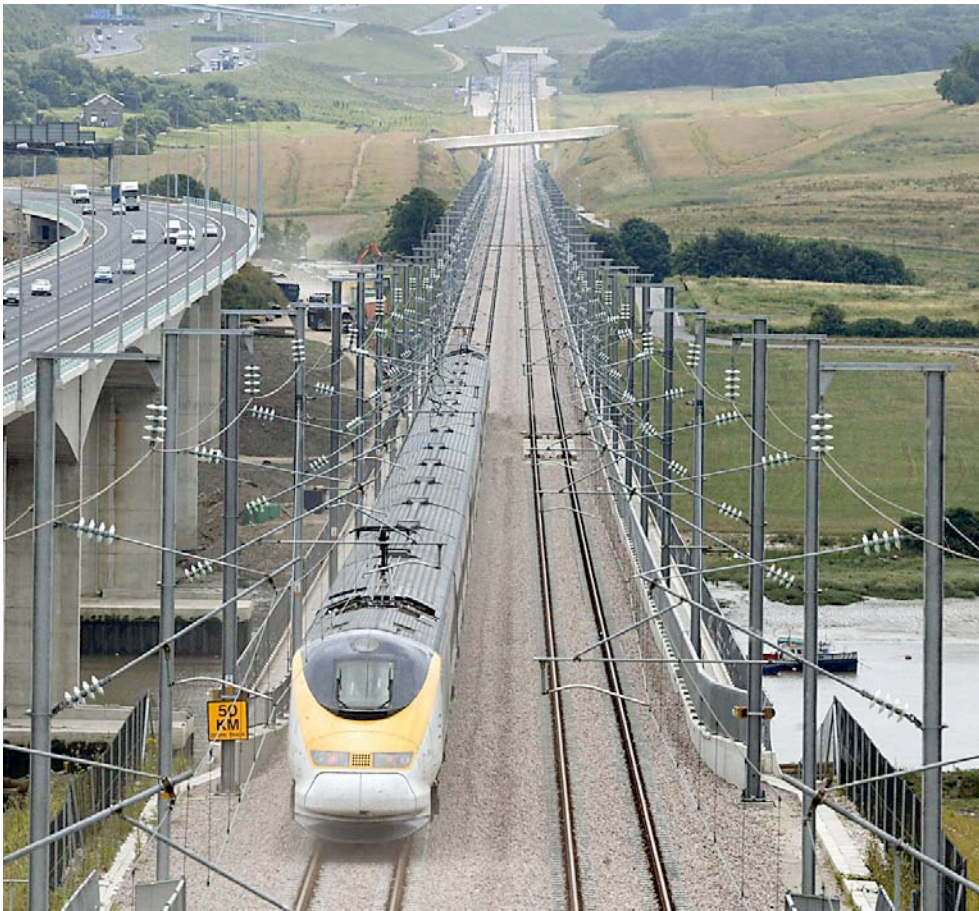
Figure 2-2: Twin block sleepers, Channel Tunnel Rail Link, UK (2005)
