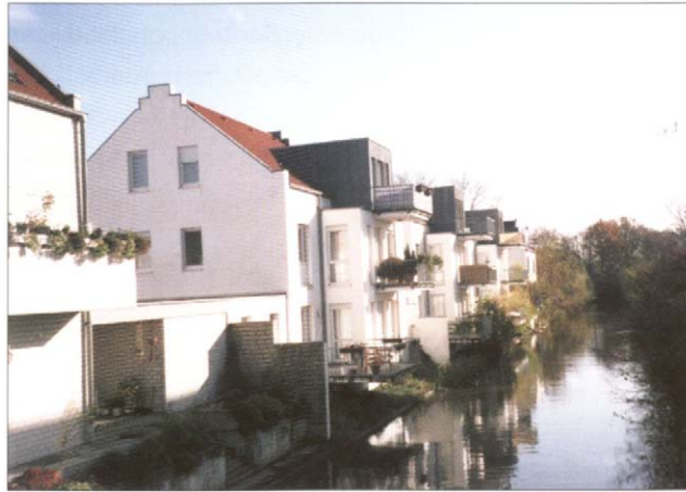
German design and construction skills in evidence in Nordhorn
