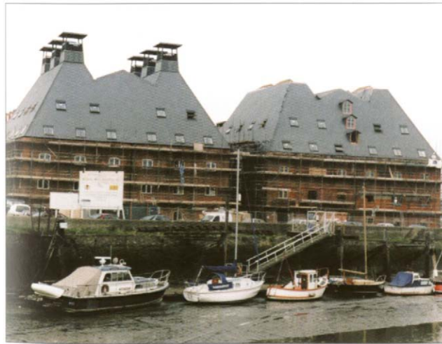
Restoring the Felaw Malting, Ipswich Wet Dock (Ipswich Council)
