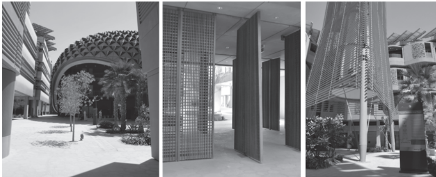
Figure 16.4 Masdar's architectural design directs desert sun and winds to enhance urban living. (Left to right): school class in front of the library, wind breakers and Masdar Cooling Wind Tower. (Source: authors.)
