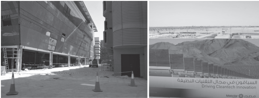
Figure 16.5 Construction works at Masdar City in 2013 (source: authors).
