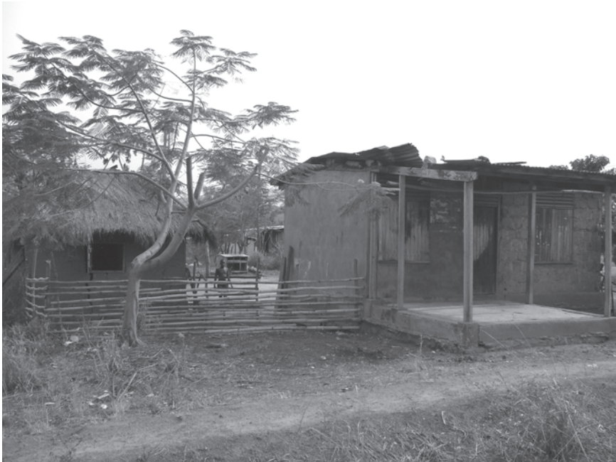
Figure 15.1 A ‘core-house’, typical of those provided to resettlers throughout the 54 resettlement townships. Note the front porch, intended for infill as an additional room. A separate kitchen has been added to the side. (Source: author.)
