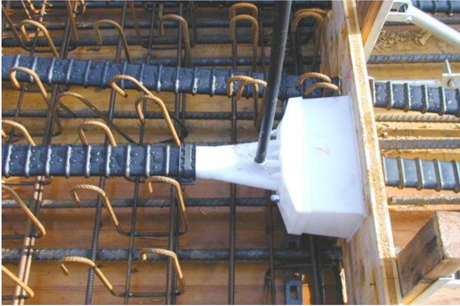
Figure 2.34: Stressing anchorage of group 1
