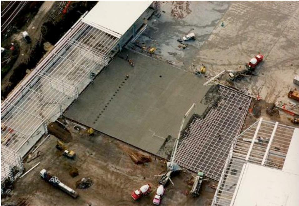
Figure 4.15: 100 t container stacking area under construction
