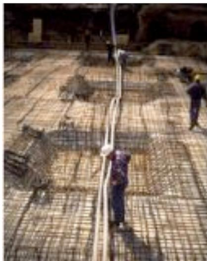
Figure 4.9: Placing the prestressing cables within the column strips
