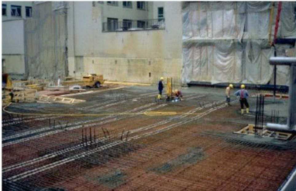
Figure 3.36: Floor slab reinforcement: prestressing cable and top reinforcement
