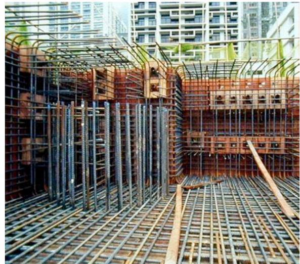
Figure 5.5: a) Wall and support lay-out and typical tendon arrangement
