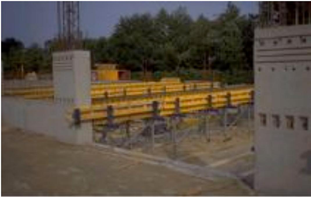
*Figure 3.18: Downstand beams in the formwork*
