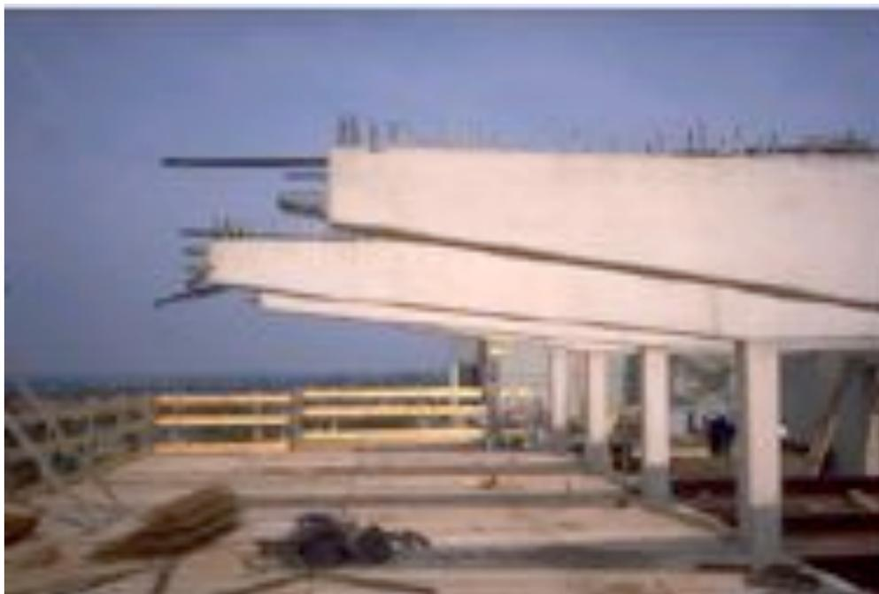
*Figure 6.11: Cantilevering prefabricated beams during construction*
