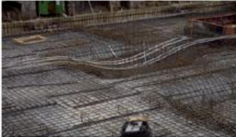
*Figure 4.10: Relieving the stresses by means of prestressing cables in the thickened parts of the raft foundation*
