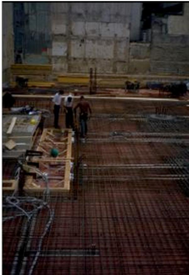
*Figure 3.38: Installation openings also serve as anchoring points for the prestressing cables*
