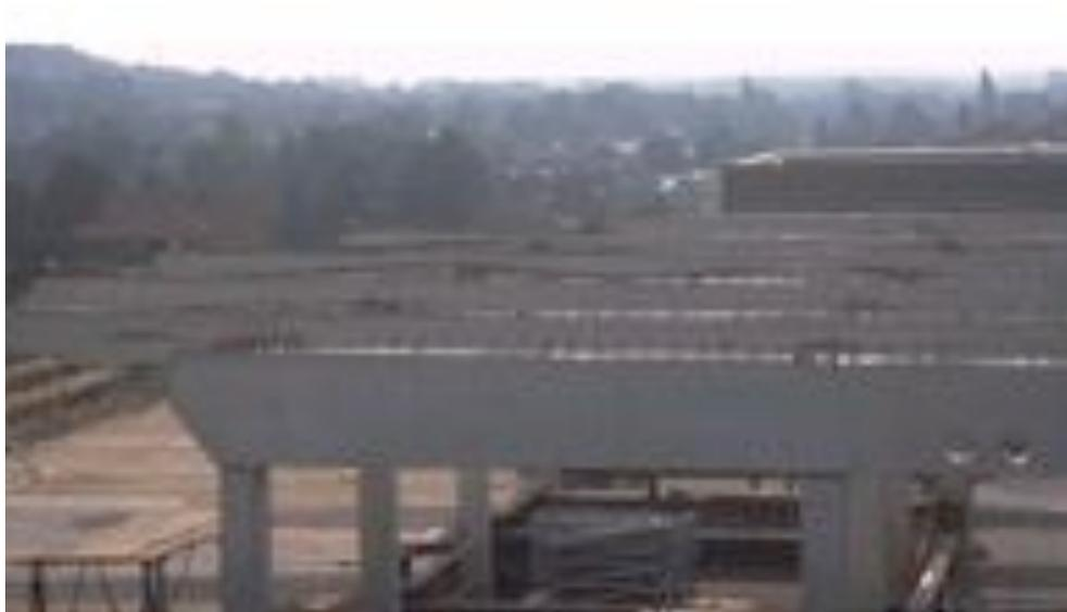
*Figure 6.10: Construction stage prefabricated beams placed and fixed*
