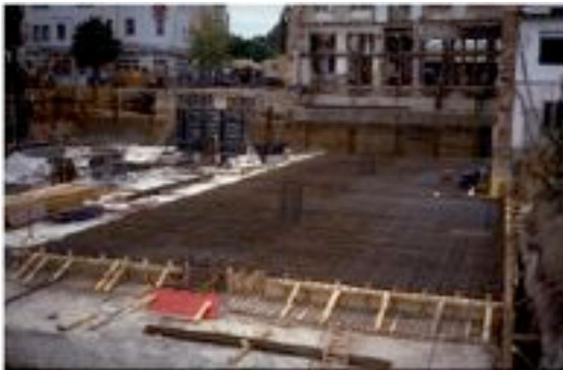
*Figure 4.11: Reinforced raft foundation construction stage*
