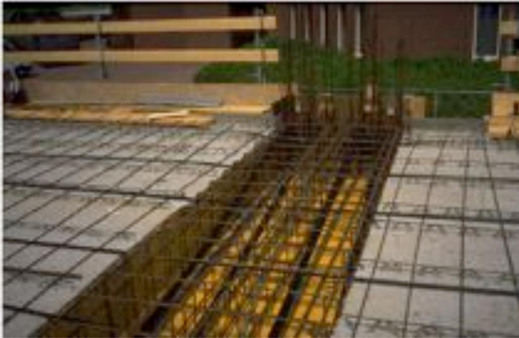
Figure 3.20: Reinforcement arrangement (prestressing and untensioned reinforcement) for the downstand beam and deck
