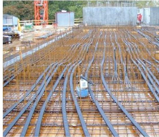
Bonded slab post-tensioning system
