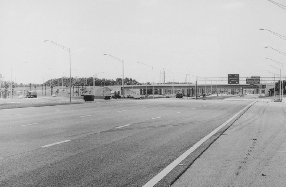
Plate 8.10 Medium severity rutting.
