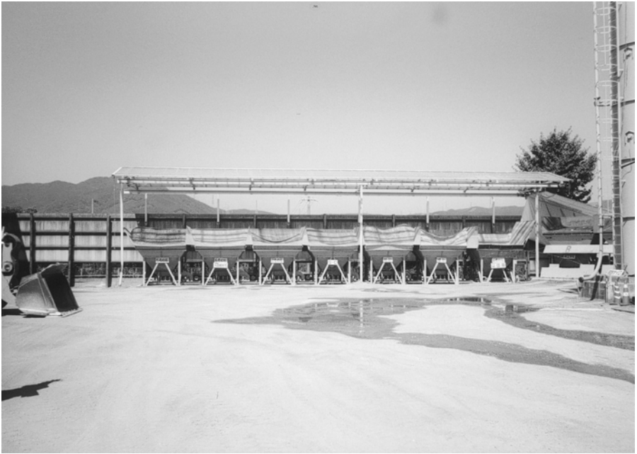
Plate 6.4 Multiple bin cold feed system.
