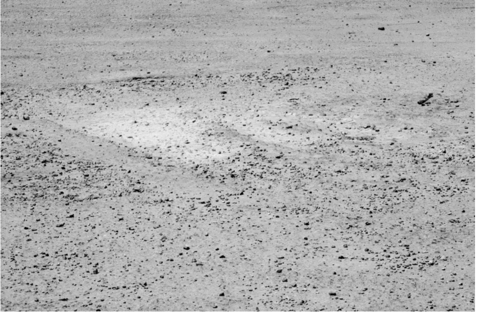
Plate 8.5 High severity raveling.
