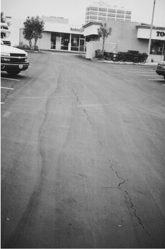
Plate 9.24 Sealcoat on top of a crack.
