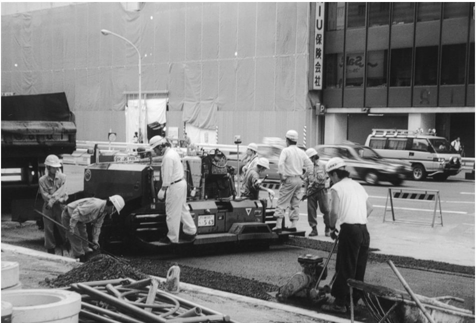
Plate 6.31 Paving process.
