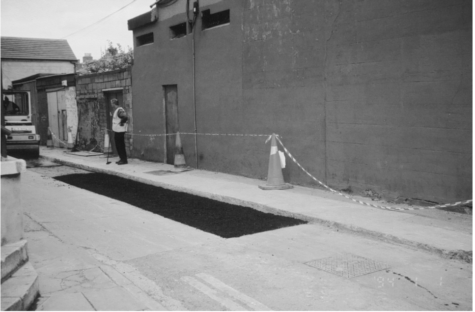
Plate 9.5 Utility cut patching.
