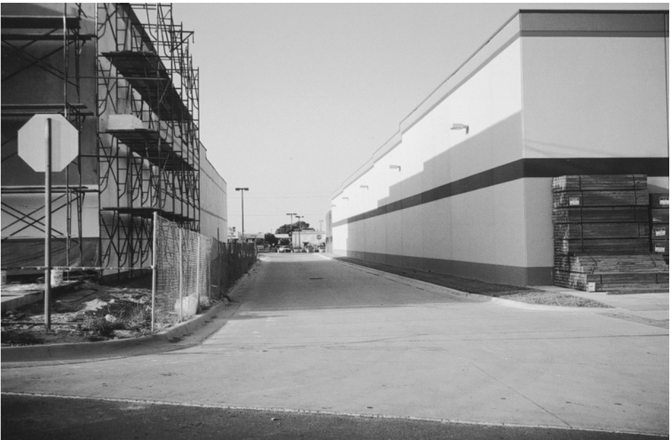
Plate 4.5 Portland cement concrete service alley with an asphalt pavement parking lot.
