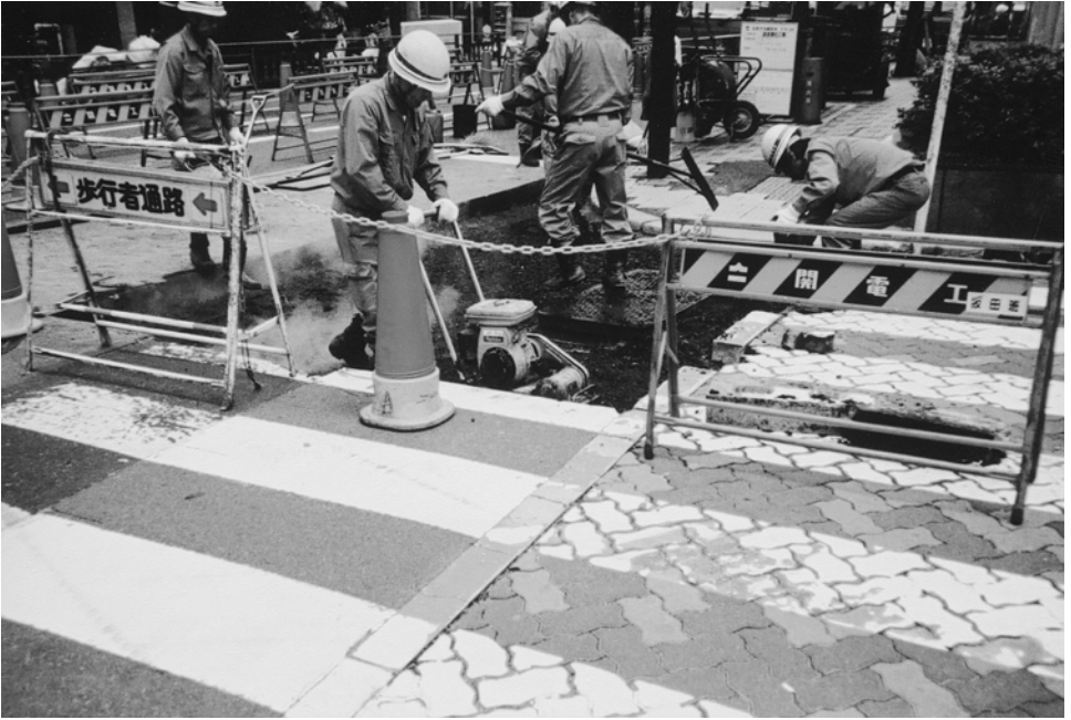
Plate 9.10 Vibrating plate compactor.
