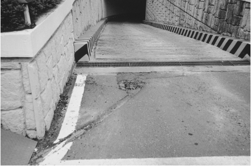
Plate 9.4 Pothole hazard.
