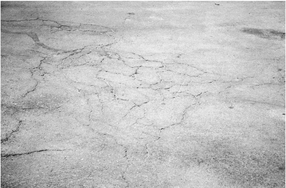
Plate 8.24 Subgrade failure.
