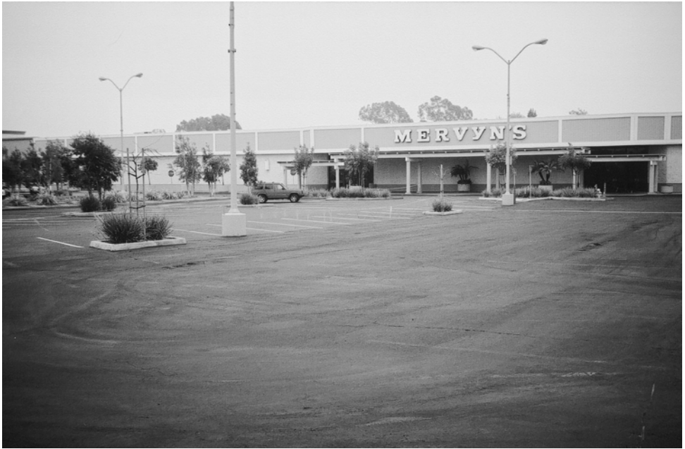
Plate 9.22 Sealcoat blocked off.
