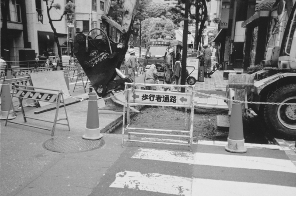
Plate 9.6 Patch excavation.
