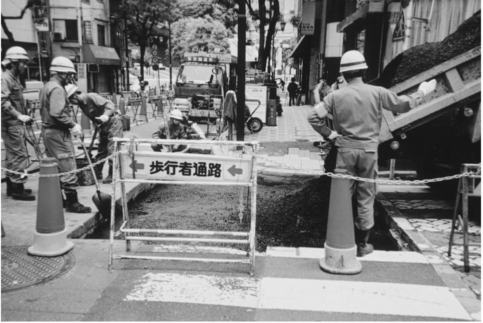
Plate 9.8 Dumping the mixture.
