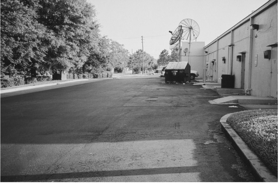
Plate 4.6 Asphalt pavement used for a service alley.
