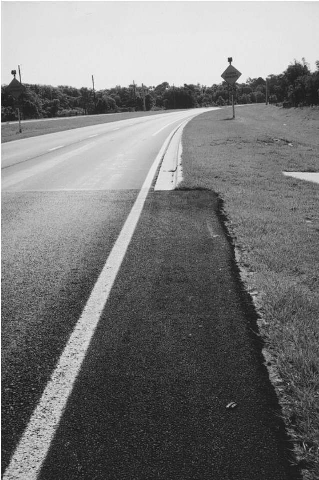
Plate 7.5 Porous asphalt next to curb.
