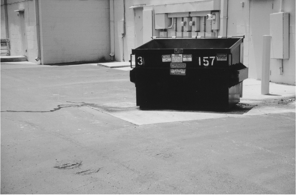
Plate 8.12 Distortion caused by a refuse truck.
