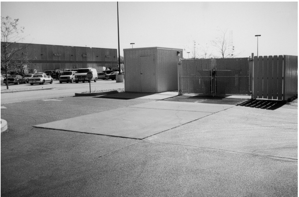
Plate 4.4 Portland cement concrete refuse container pad.
