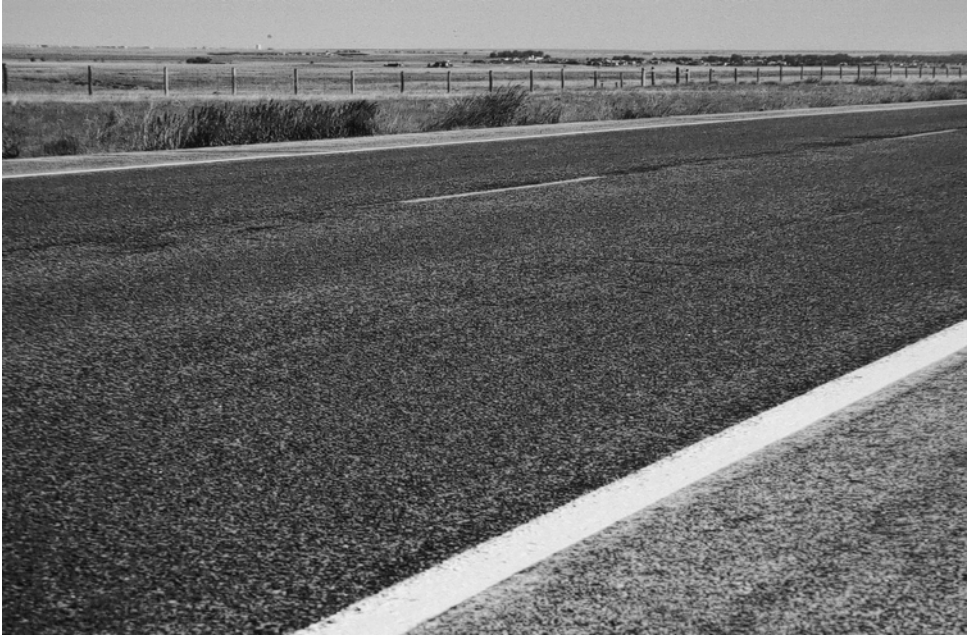
Plate 9.26 Chip seal texture.
