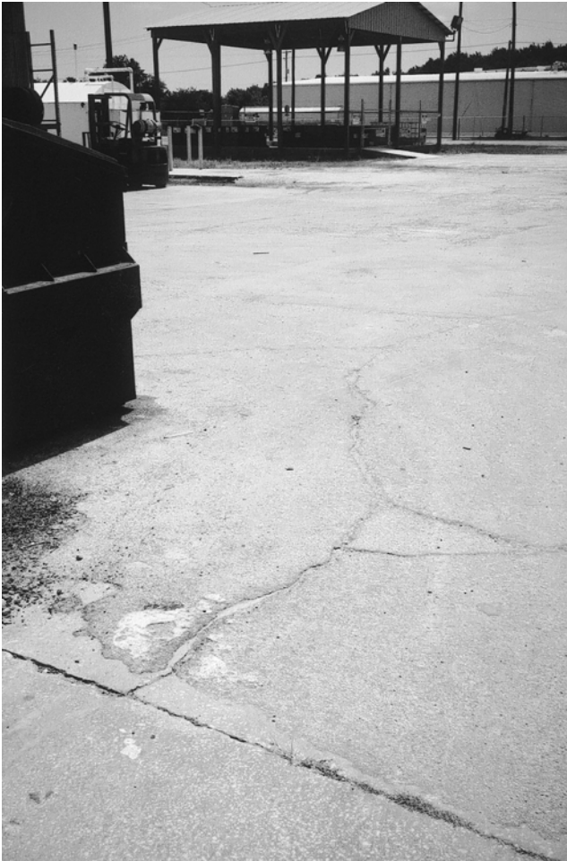
Plate 8.20 Reflective crack.
