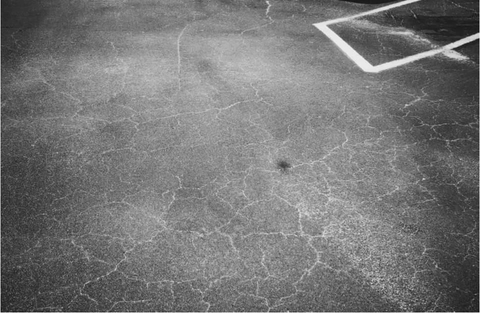
Plate 8.23 Alligator cracking.
