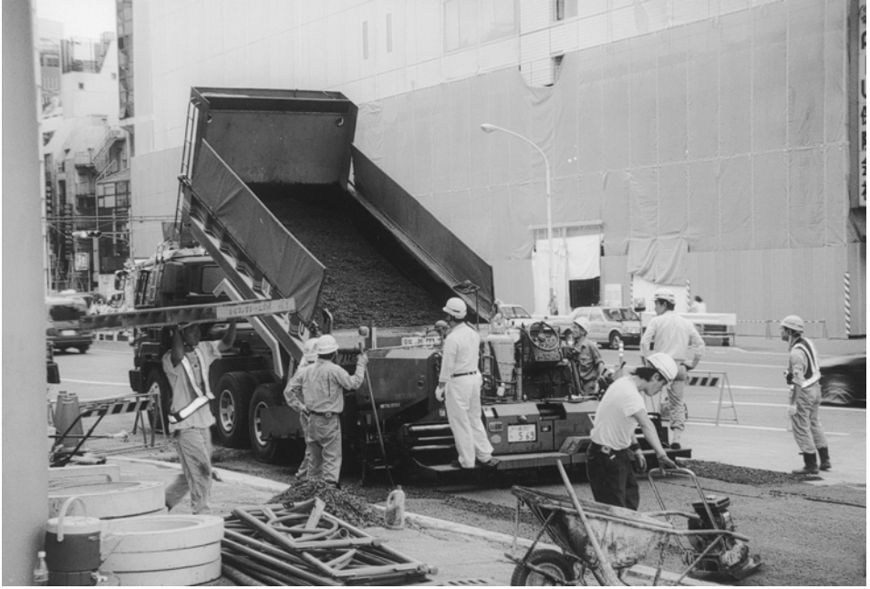
Plate 6.15 Discharging into paver.
