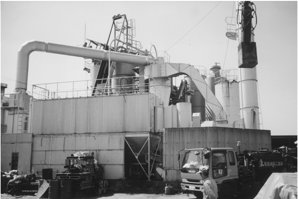
Plate 6.2 Small stationary batch plant.
