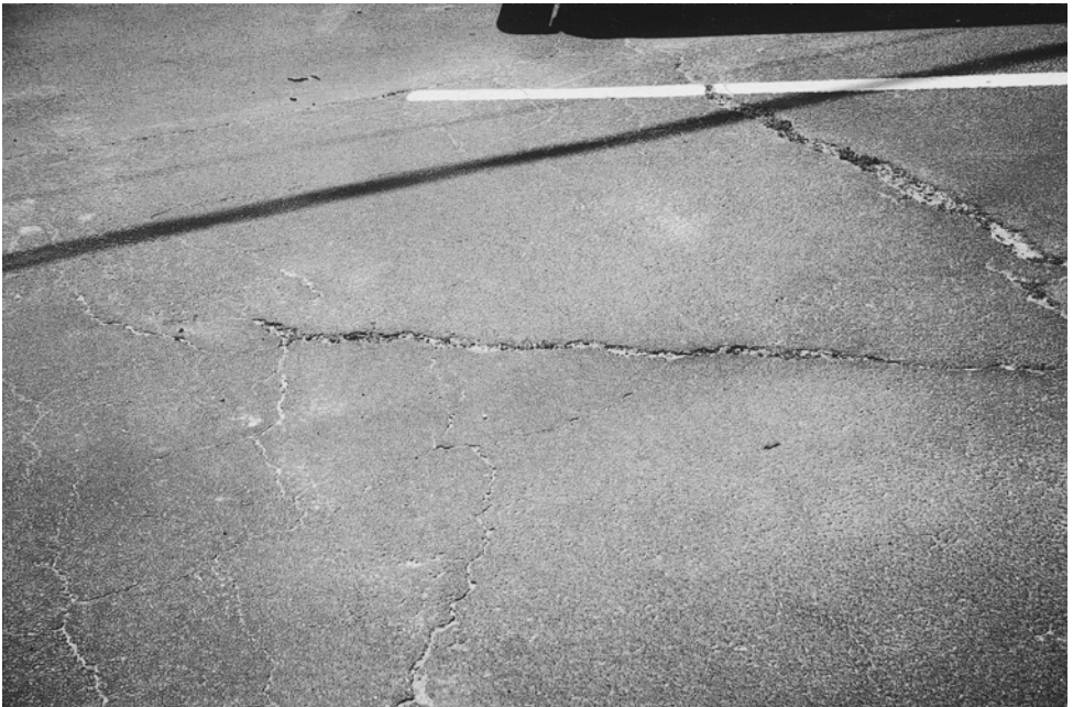
Plate 8.22 Block crack.
