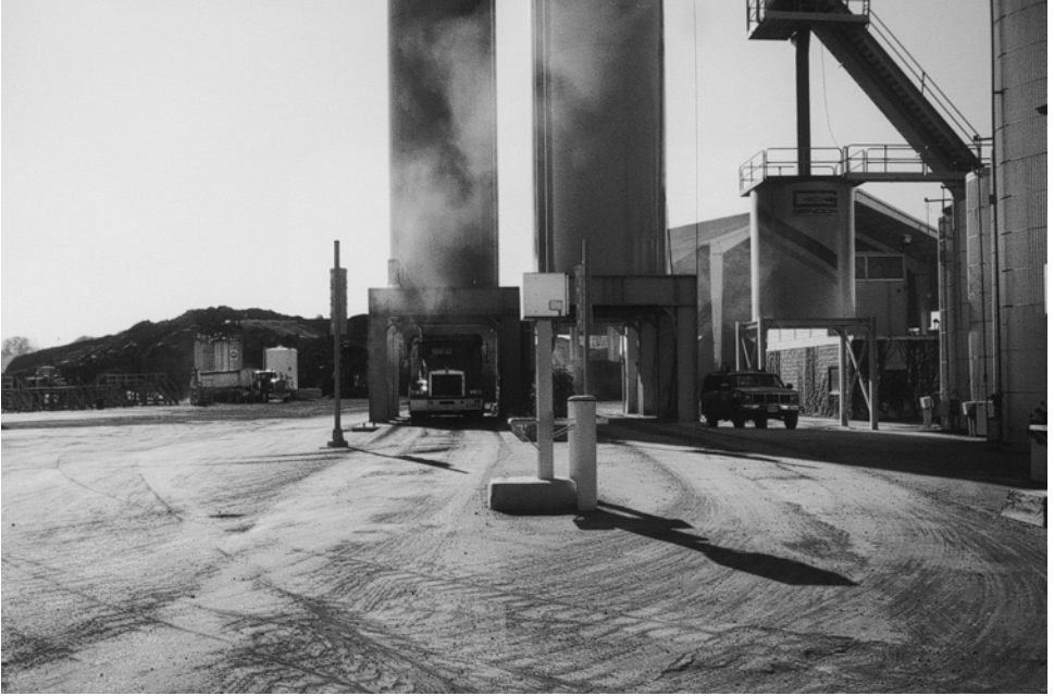
Plate 6.6 Multiple storage silos at a drum mix plant.
