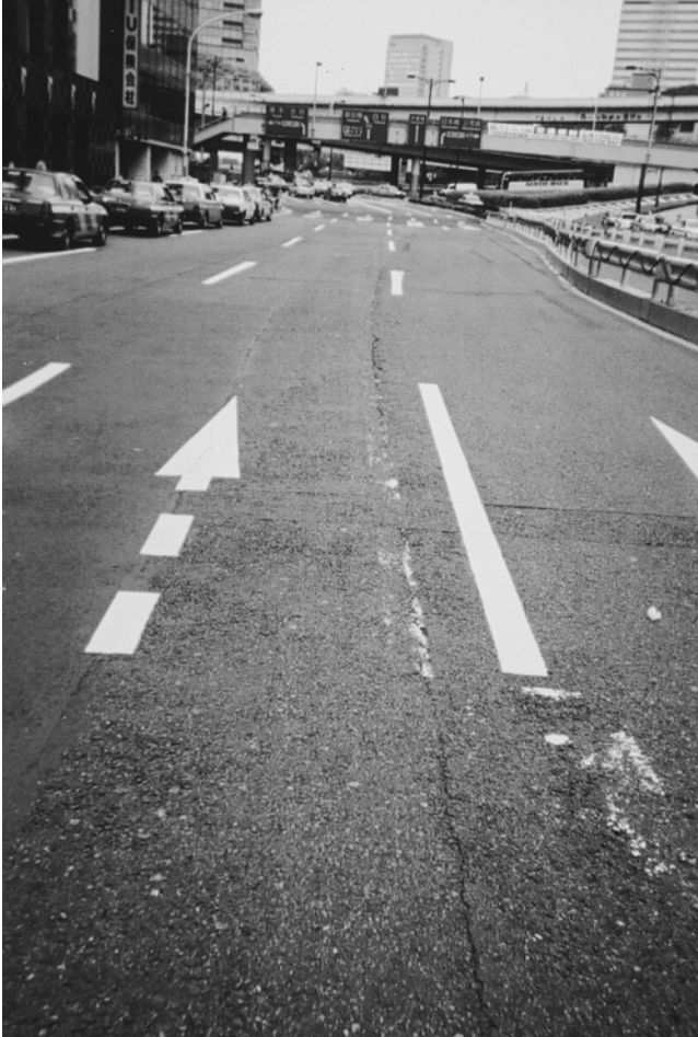
Plate 8.15 Longitudinal cracking.
