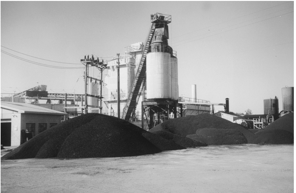
Plate 6.7 Large surge bin.
