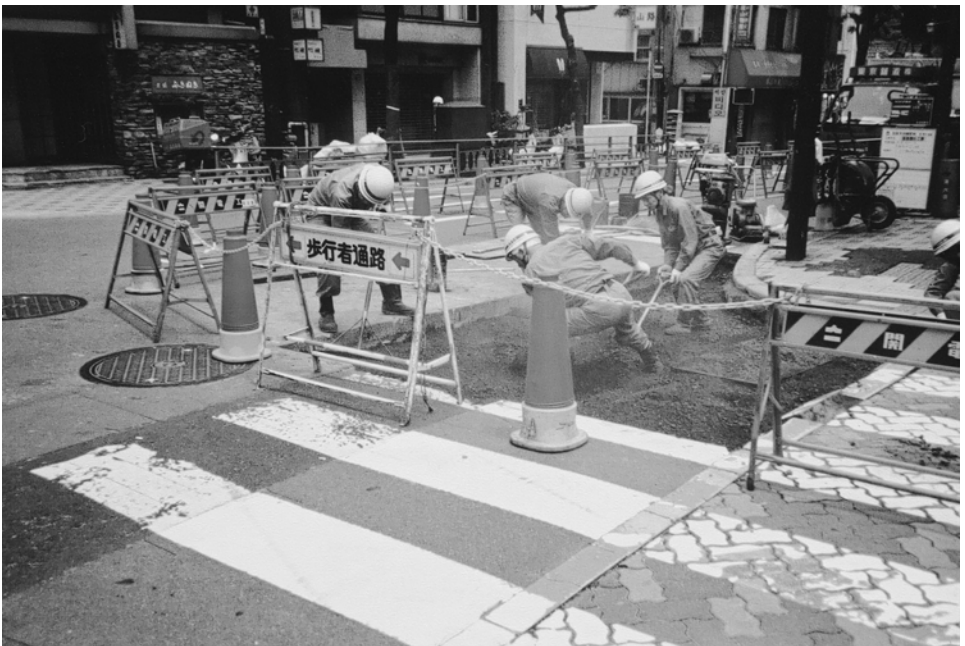
Plate 9.9 Spreading the mixture.
