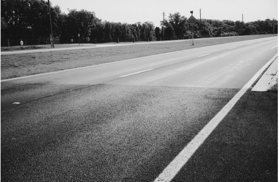
Plate 7.6 Transition between porous asphalt and a dense graded wearing course.
