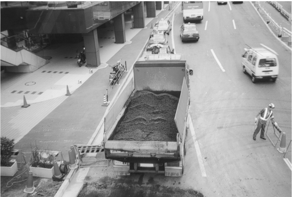
Plate 6.17 Separate batches in truck.
