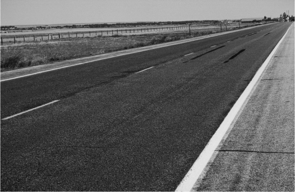
Plate 9.25 Chip seal or surface dressing.
