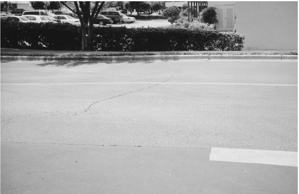
Plate 8.14 Transverse crack.
