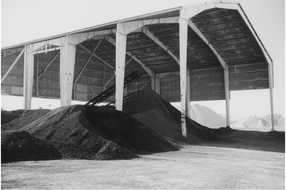
Plate 2.3 Large RAP stockpile.
