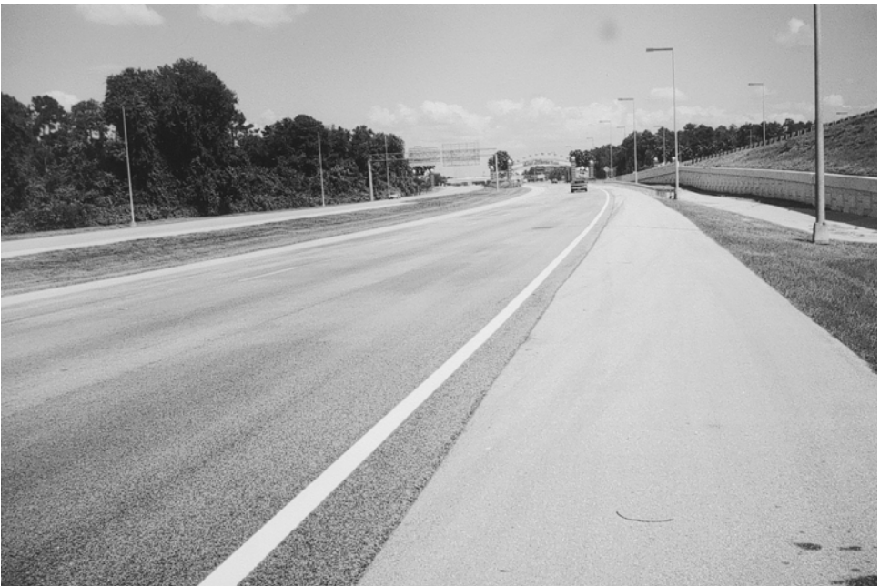
Plate 8.8 Moderate flushing.
