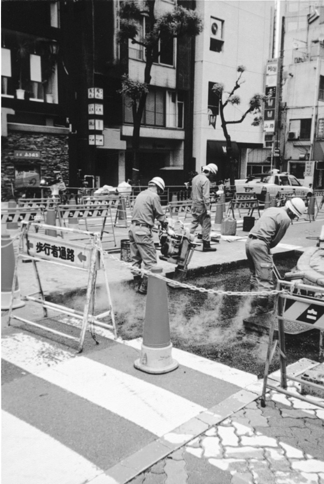
Plate 9.12 Tamping foot compactor.
