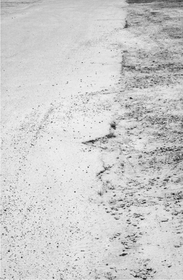
Plate 8.19 Edge failure.
