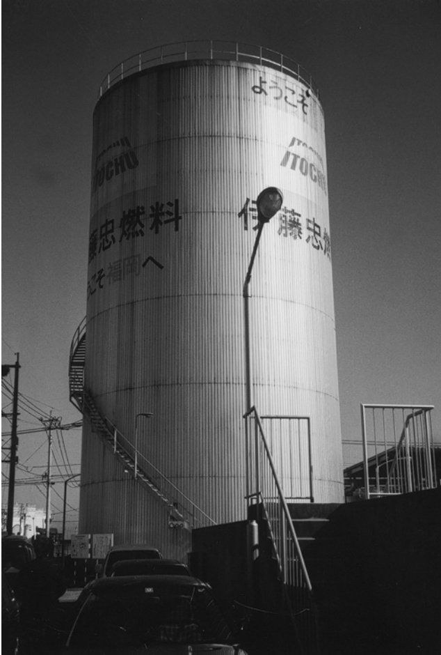
Plate 1.2 Single tank asphalt terminal.
