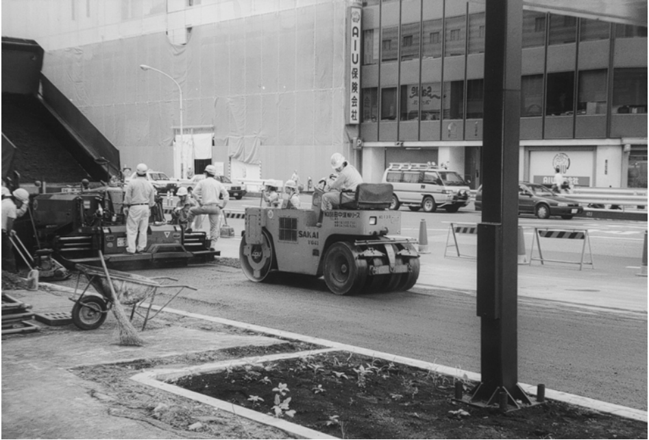
Plate 6.41 Combination roller approaching paver.
