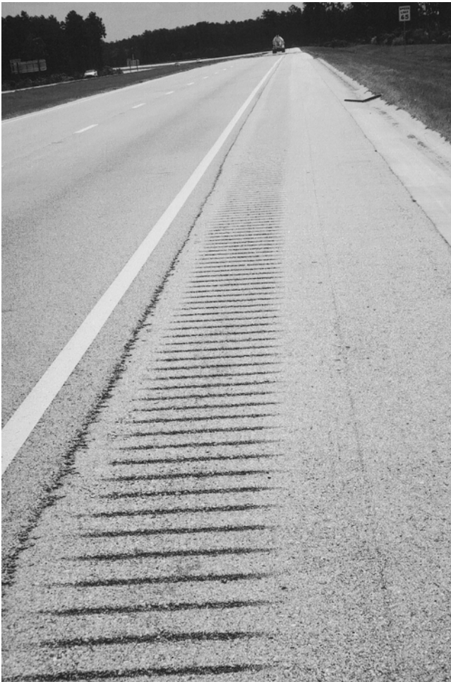
Plate 7.3 Porous asphalt wearing course with “daylighted” edges. Also note the rumble strip that is pressed into the shoulder.
