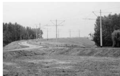
Figure 14. Embankment after completion of the construction.
