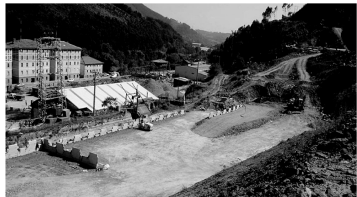
Figure 1. General view of the site.
