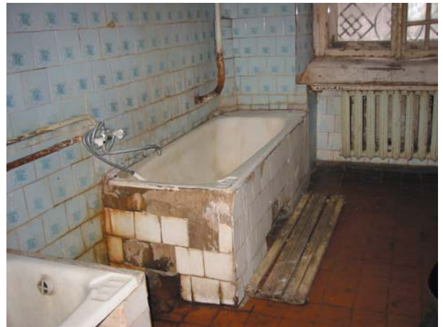
Plate 6 Bathroom on an old age psychiatry ward somewhere in the former USSR. Note (a) the obvious state of dilapidation; (b) more than one tub (in fact there were three) negates privacy; (c) baths are against the wall preventing nurses from being either side of a disabled patient; (d) such a bathroom is typical of thousands in the region.
