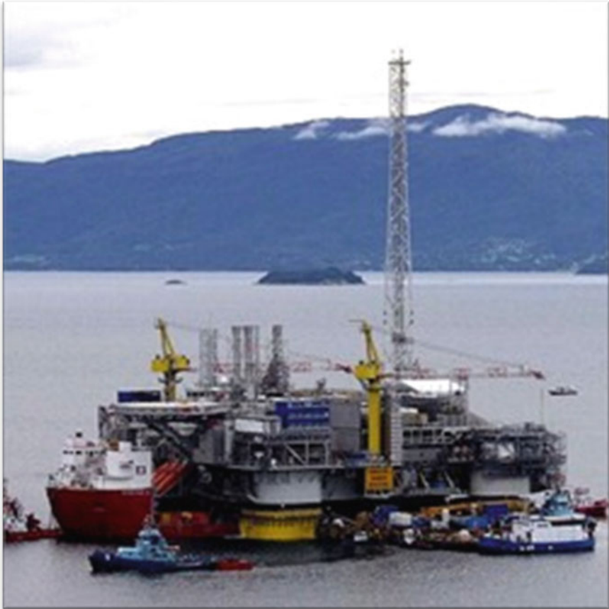
Fig. 2.39 Inshore deck floatover installation of semisubmersible platform Kristin (courtesy of Statoil)
