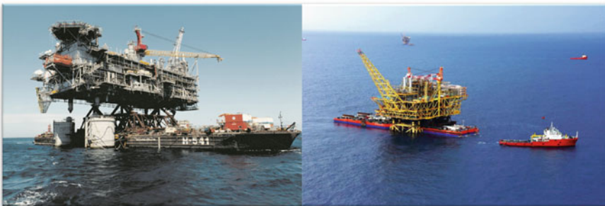
Fig. 4.12 Examples of floatover installation. On the left is the Shell's Malampaya platform with the weight of the topsides being 11,600 tons, installed in 2001. On the right is the Liwan 3-1 topsides with the weight of 32,000 tonnes installed in 2013 (Courtesy of Shell and CNOOC respectively) [16]
