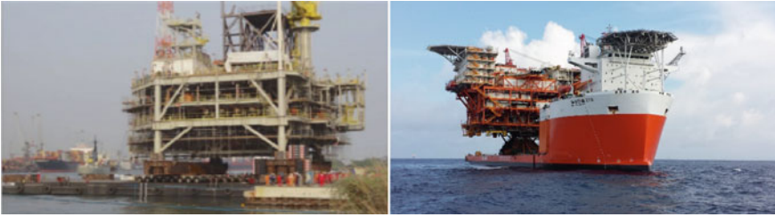
Fig. 1.27 Differences in the structure design of topsides for transportation (Courtesy of Chevron and CNOOC)
