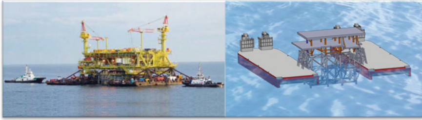
Fig. 6.20 Catamaran floatover mating operation. On the left is Kikeh spar floatover; on the right shows catamaran floatover used for a fixed platform integration (photo Courtesy of Technip) [18]
