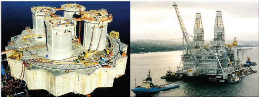
Fig. 2.36 Hibernia platform integration. The base structure of Hibernia is shown on the left and the right shows the topsides was transported by two giant barges to the integration site (courtesy of HMDC)
