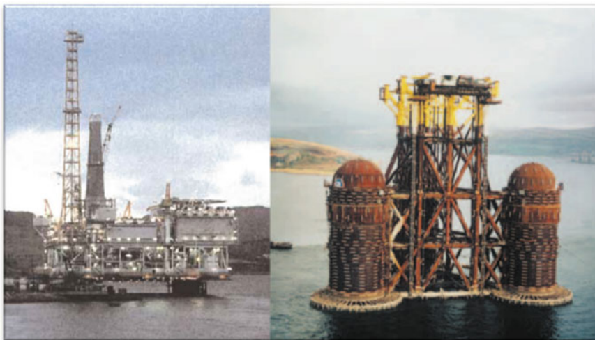
Fig. 4.5 The topsides of Maureen Alpha platform was built over water spanning between the quayside and a row of piled supports; It was carried by H-114 to the mating site ( left ). On the right is the Maureen TGS before the mating. It would be ballasted down at the mating site (Courtesy of Fagioli and ConocoPhillips respectively)
