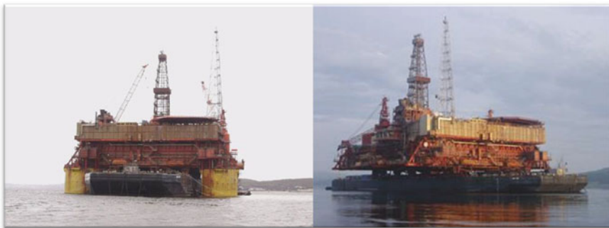
Fig. 4.10 The de-mating of Hutton topsides was carried out by Saipem barge S600 (Courtesy of ConocoPhillips)
