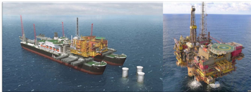
Fig. 10.15 Illustration of dismantling the topsides of Brent Delta (courtesy of Shell)
