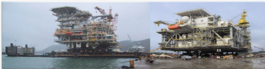
Fig. 1.18 The topsides fabrications: On the left , it shows the loadout of Lay Tay topside and on the right is the completion of the topsides of Blind Faith (Credit to the BP Lan Tay and Chevron Blind Faith projects)
