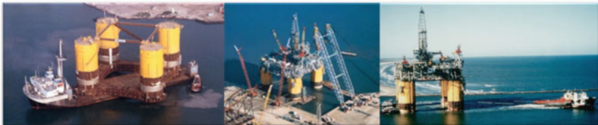
Fig. 2.29 Shell TLP Mars integration. The left photo shows the Mars' hull being carried by Mighty Servant 2 of Dockwise; the center shows the installation of modules; on the right , the integrated platform was wet-towed to the field (courtesy of Shell)
