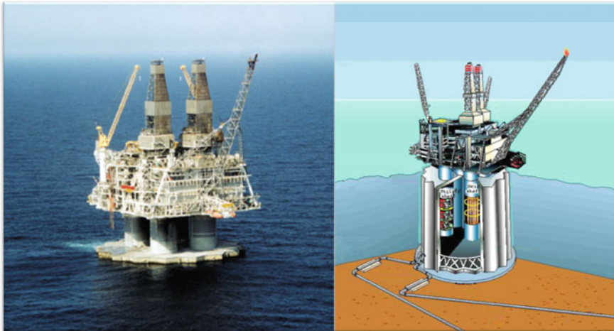
Fig. 6.2 The Hibernia GBS platform after integration [courtesy of Hibernia Management and Development Company Ltd. (HMDC)]
