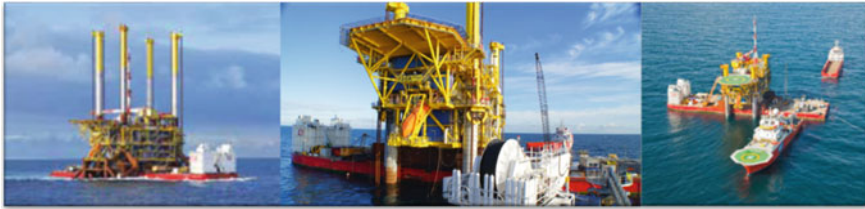
Fig. 2.16 Stationing operation at site. The center is a photo showing the BB35 with the F3-FA platform aboard during operation. The left illustrates the operation of the leg lowering; the right illustrates the completion of the F3-FA platform and BB35 being sailing away (courtesy of SPT Offshore)
