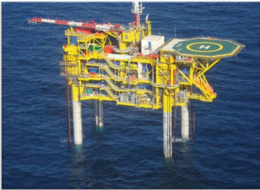
Fig. 2.17 The F3-FA platform after the topsides & legs locked. The strain jacks can still be seen (courtesy of SPT Offshore)
