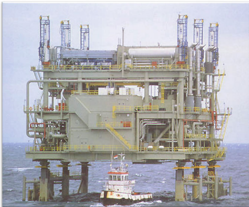
Fig. 5.12 The EKPE gas compression platform after the completion of floatover operation using ETPM's SMARTLEG technology. The vessel preparation took three days, but the floatover operation only last three hours (courtesy of ETPM)
