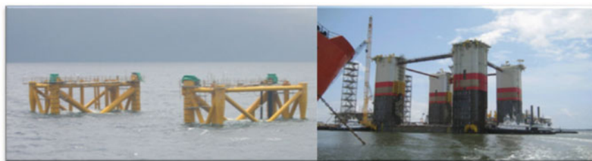
Fig. 1.19 The mating sites for Lay Tay platform and DDS Blind Faith (Credit to the BP Lan Tay and Chevron Blind Faith projects)
