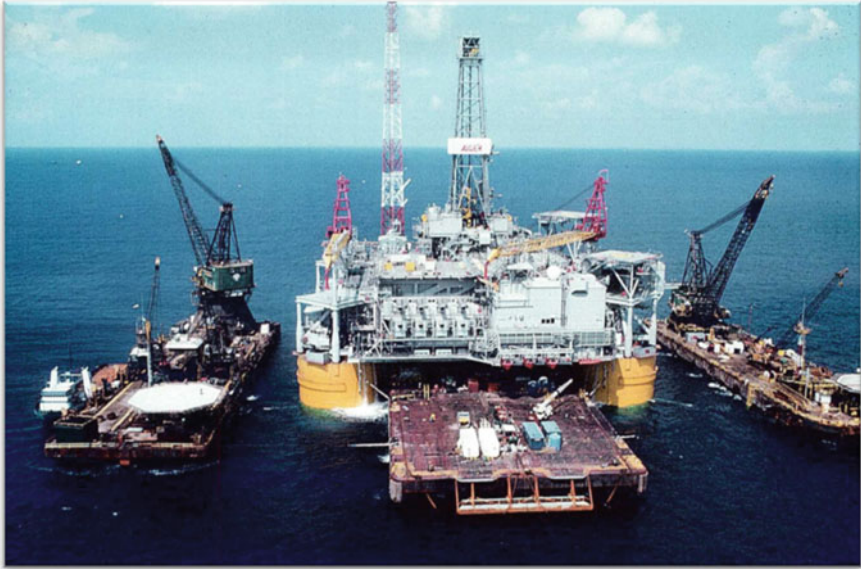
Fig. 2.57 The hull and topsides mating operation for Shell Auger TLP. McDermott's Intermac 650 carried the topsides weighing 24,000-tons. The top of the TLP column was 7 m (23 ft) above the water surface. The two derrick barges were not only standing by, but also assisting the mating operation (courtesy of Shell and McDermott)
