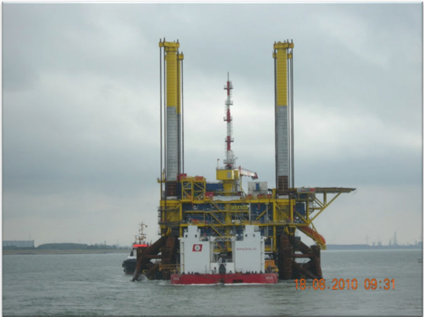
Fig. 2.15 SIP II platform being transported to the field. The limited transportation weather window is H_s = 4.0 m (courtesy of BOA Group)
