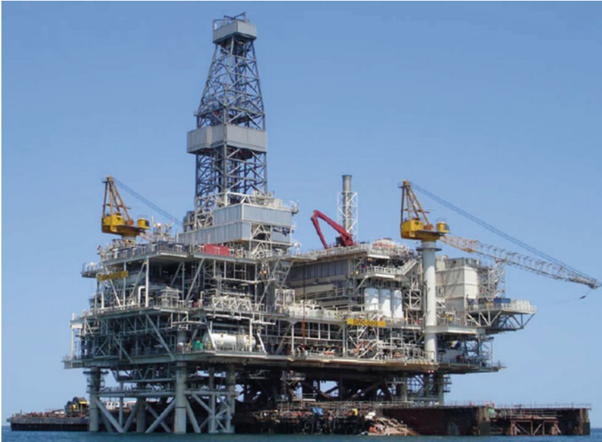
Fig. 4.13 ACG Topsides Floatover Installation in Caspian Sea [17]
