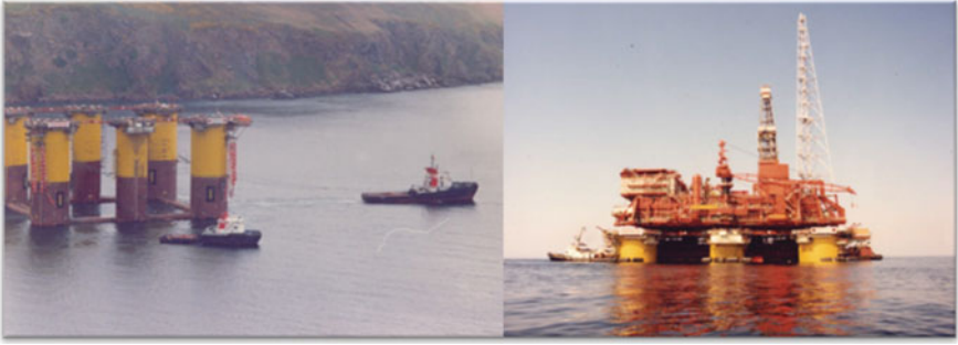
Fig. 2.38 The Conoco’s Hutton production TLP was integrated using floatover method (courtesy of Conoco)
