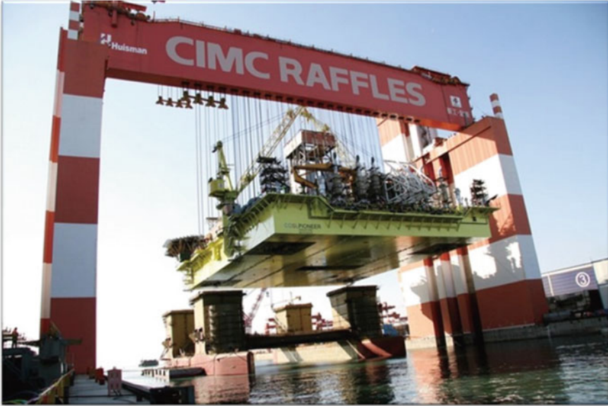
Fig. 2.40 The 14,000 tonne integrated topsides of the COSL Pioneer drilling semisubmersible had been lifted and the hull was moving in underneath (courtesy of CIMC Raffles)
