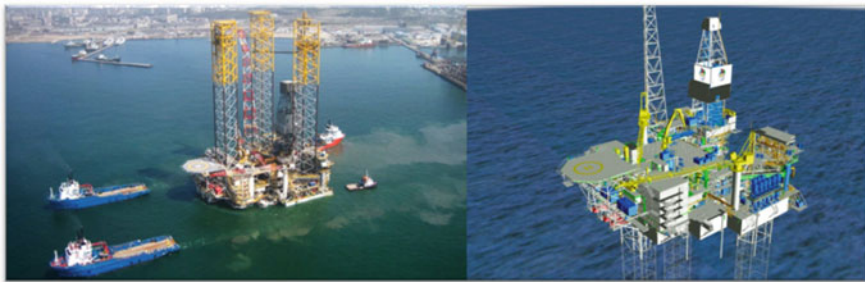
Fig. 2.1 BP Shah Deniz TPG500 production platform which is a Jack-up with 3 legs (courtesy of BP and Keppel Group respectively)
