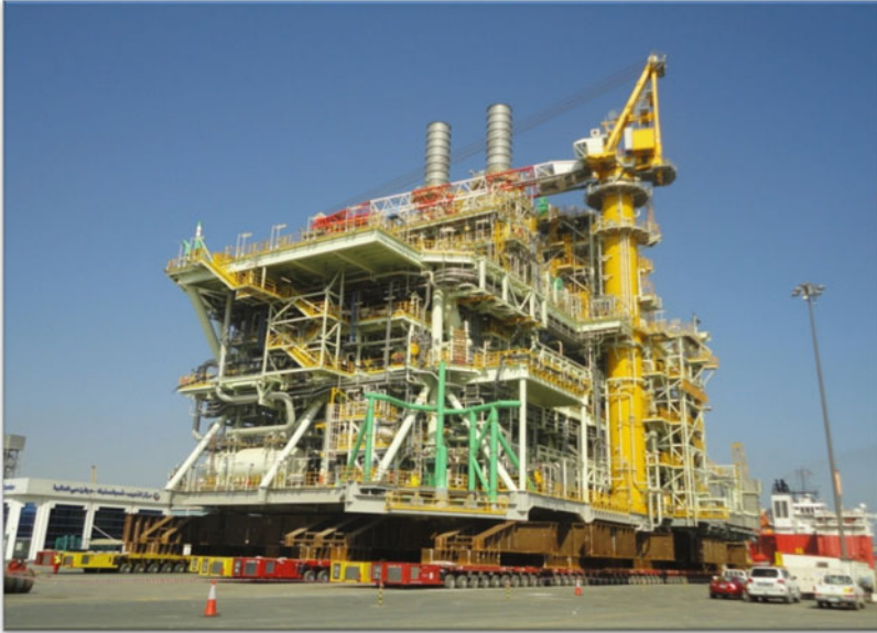
Fig. 1.4 A completed topsides is ready for loadout (Courtesy of Nexen Petroleum U.K. [5])
