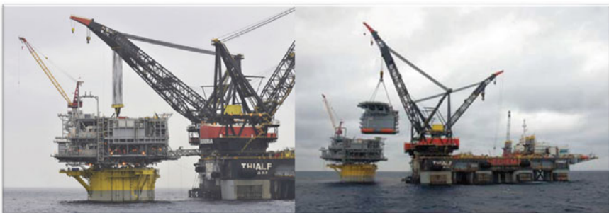
Fig. 1.14 On the left the lightweight single lift topsides is installed to the Perdido hull by HMC's Thialf with one single lift and then the living quarter module was put atop the topsides three days later (Courtesy of Shell)
