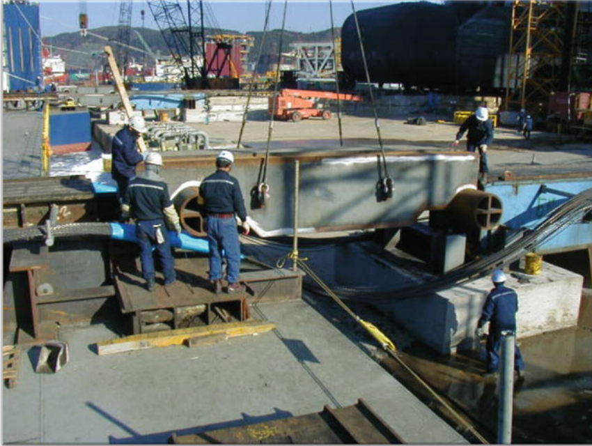
Fig. 9.9 Installing the link-beam (Photo credit to Bayu Undan project)
