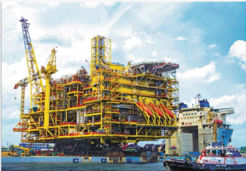
Fig. 1.10 An integrated topsides for floatover installation in Malaysia (KBB project) (Courtesy of KPOC)
