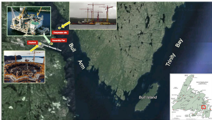
Fig. 6.3 Construction of Hibernia topsides and GBS (based on public information of Hibernia project from website)
