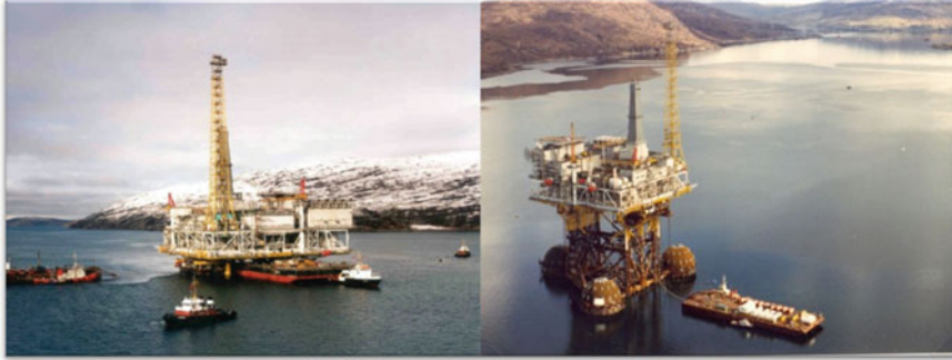
Fig. 4.6 On the left , it shows the platform integration operation inshore, the Maureen TGS was ballasted down leaving about 8 m (26.2 ft) of the jacket top emerging above the water. It can be seen on the right , after the H-114 withdrawing, the Maureen Alpha platform further deballast and ready for towing off (Courtesy of Oilrig.Hunterston.eu)
