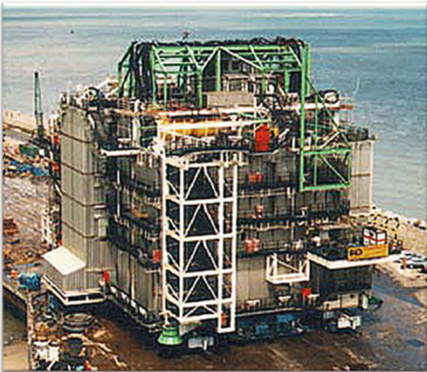
Fig. 1.9 Living quarter of Miller platform (Courtesy of BP)
