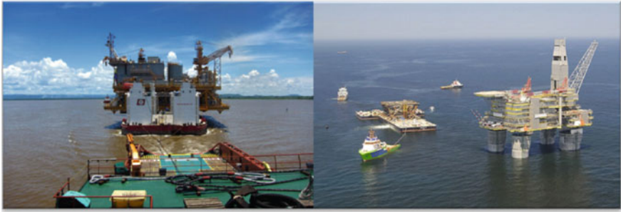
Fig. 3.10 Floatover method can be used in very shallow water with high mating load as shown on the left for the COCOCORO project—the water depth is 5 m and the mating load was 7400 tonnes. On the right is the Sakhalin LUN-A platform, the topsides weighed 21,800 tonnes (courtesy of conoco and shell respectively)
