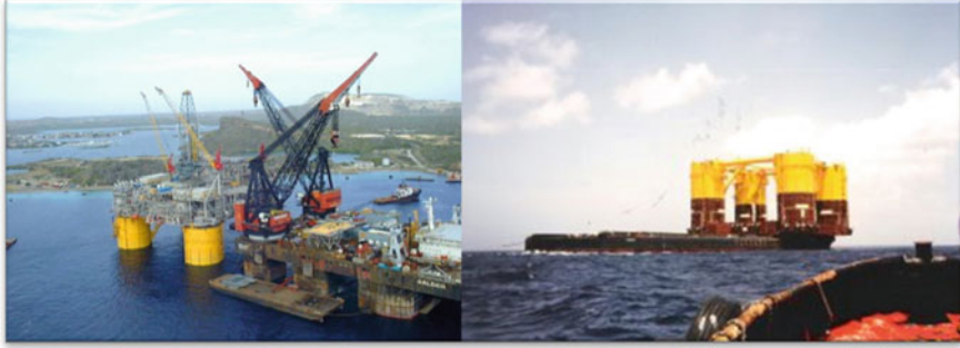
Fig. 2.30 The left photo shows the Ursa hull being transported from Italy to the integration site offshore Venezuela on barge H-851. On the right , the HMS's SSCV was lifting modules during the installation. The sheltered waters were calm (courtesy of HMC)
