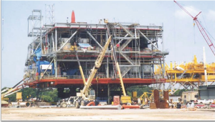
Fig. 1.8 The North Module is half of the whole Petronius topsides weighing 7500 t (Courtesy of Chevron)
