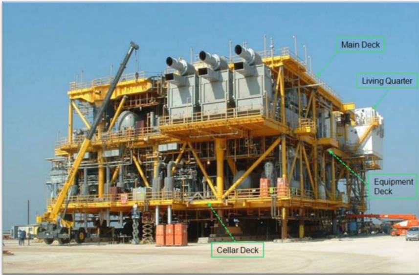
Fig. 1.2 A topsides shows multi-level decks populated with modules (Courtesy of Anadarko Petroleum Corporation [3])
