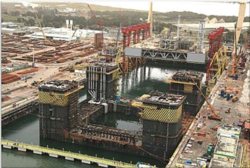
Fig. 2.41 P-55 platform integration in the drydock of Rio Grande yard (courtesy of Petrobras)
