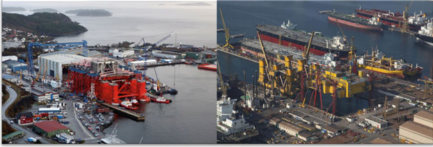
Fig. 2.46 Both the drydocks are open to the sea. On the left , it can be seen that three (3) tugs are used to push the hull to move in underneath the elevated topsides (courtesy of Aerophoto.no and Drydocks World separately)
