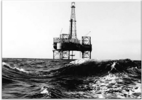
Fig. 2.3 The first jack-up scorpion is designed and fabricated by R. G. LeTourneau, Inc. The hull size is 186 \times 150 \times 24 ft and the steel legs (spuds) are 140 ft long. The platform weighed 4000-ton (courtesy of Rowan)
