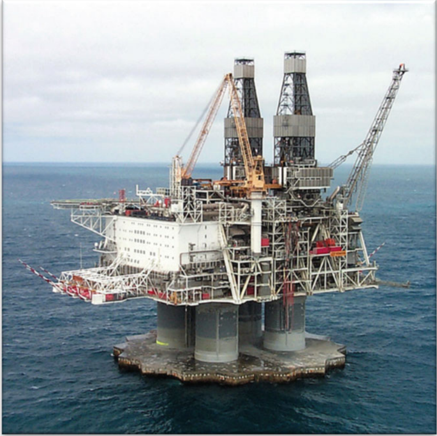
Fig. 2.35 Hibernia platform (courtesy of HMDC)
