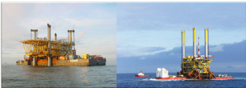
Fig. 2.8 SIP II concept platforms: on the left is Calder SIP II platform in 30 m water depth in Irish Sea, UKCS; on the right is F3-FA SIP II platform in 40 m water depth near Dogger Bank in the North Sea (courtesy of SPT Offshore)
