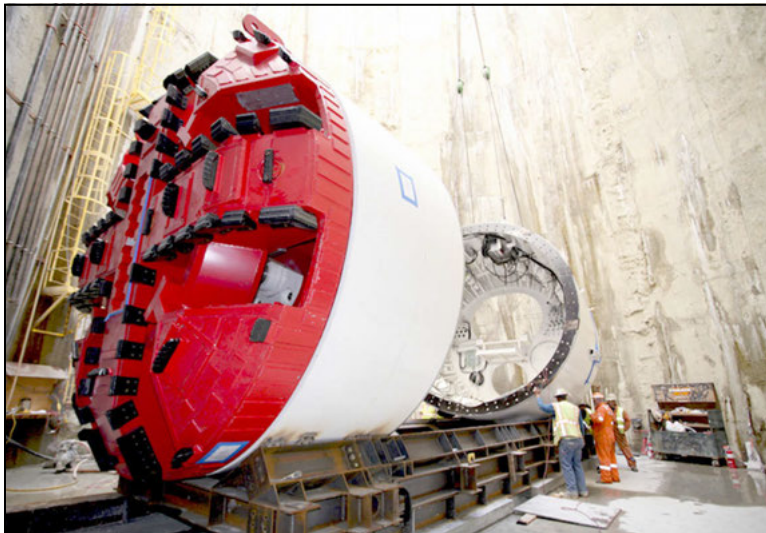
Figure 5. Assembly of the earth pressure balance machine
