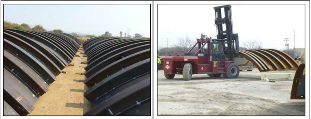
Figure 11. Quarter sections of 10m (33 ft) diameter liner
