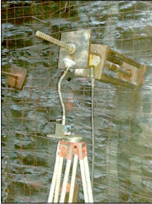
Figure 3. Rock bolt testing setup
