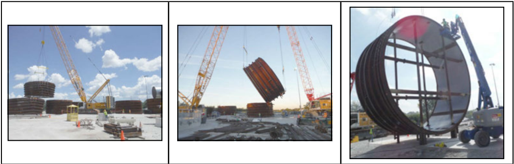
Figure 20. Bifurcation and bull nose assembly
