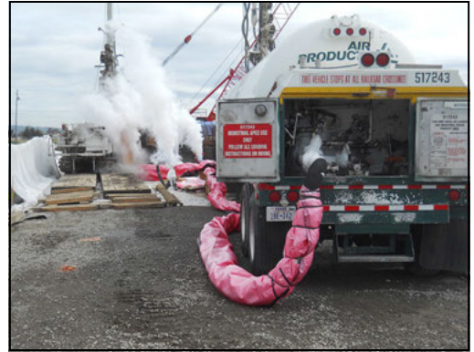
Figure 20. LN vapor escaping from vertical freeze pipes
