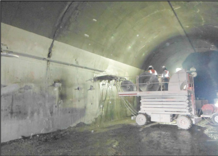
Figure 4. Diamond saw cutting of existing liner
