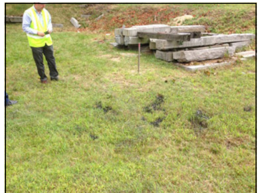
Figure 7. Slurry break out
