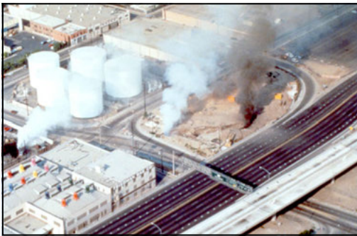
Photo 4. A130 tunnel fire and collapse segment (Courtesy of F. Gularte)
