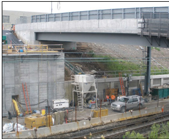
Figure 11. Shotcrete plant at ground surface
