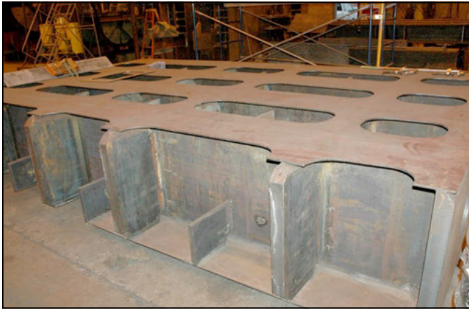
Figure 8. Gate fabrication in progress
