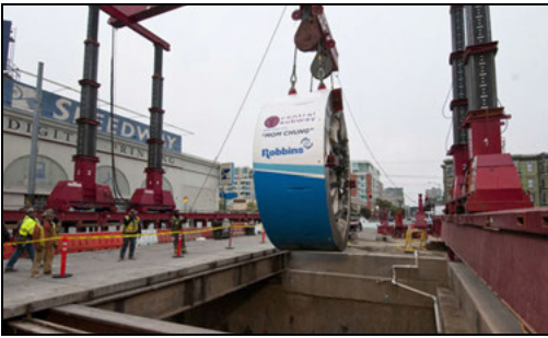
Figure 7. Lowering a section of machine shield (Image credit: SFMTA)
