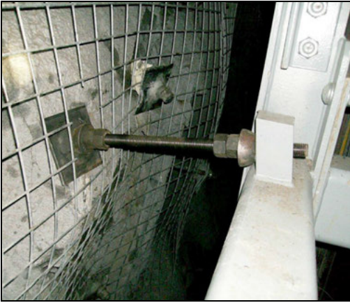
Figure 6. Set steel blocking installation
