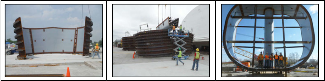
Figure 19. Bifurcation and bull nose assembly
