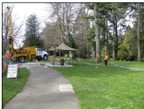
Figure 5. MPBX fiberglass rod protective tubing
