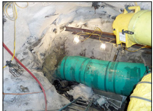
Figure 16. Completed water line section in frozen cave
