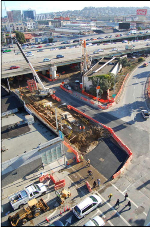
Figure 6. Small jobsite passes under Interstate highway 80 (Image credit: SFMTA)
