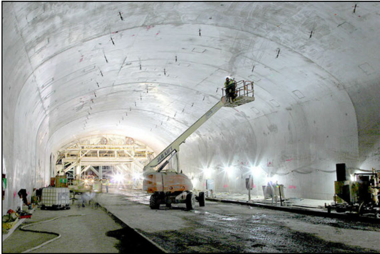
Figure 8. Tunnel concrete liner with grout packers installed
