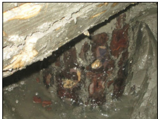
Figure 10. Exposed timber pile and cap
