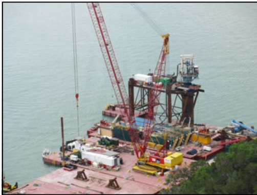
Figure 6. Intake drilling operations
