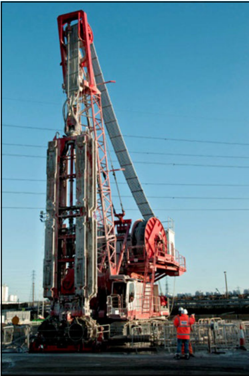
Figure 5. Hydrofraise unit for diaphragm wall construction
