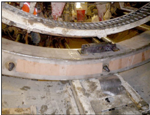
Figure 4. Stainless-steel ring beam
