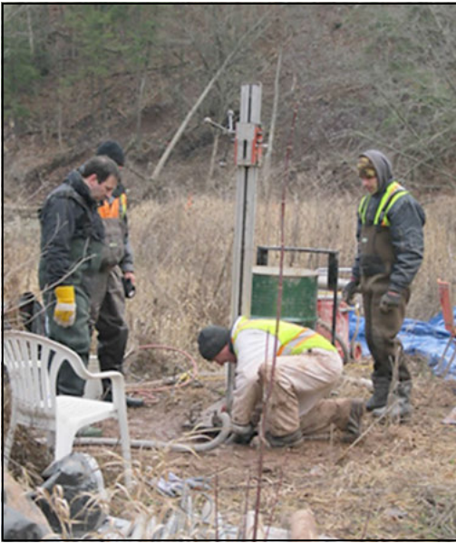
Figure 10. Rock core sampling in the valley floor
