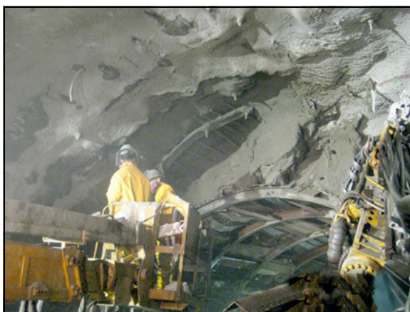
Figure 10. Sequential excavation using pre-support spiling in shear zone
