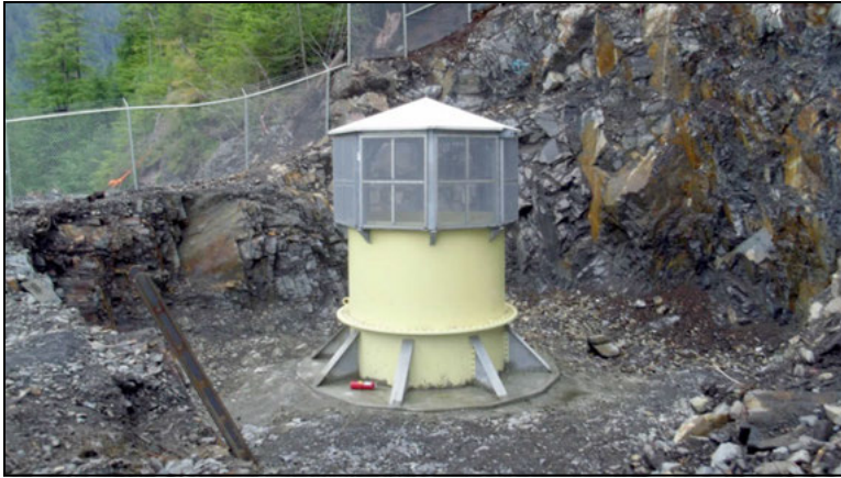
Figure 7. Completed surge shaft breakthrough steel structure
