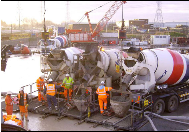
Figure 4. Three concrete trucks at a diaphragm wall primary lining pour
