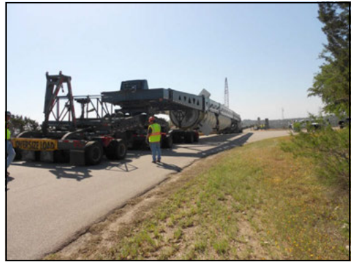
Figure 13. Crew at riser pipe
