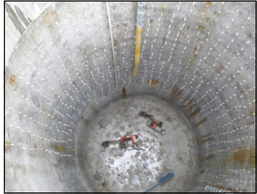
Figure 6. Main gate shaft at final depth
