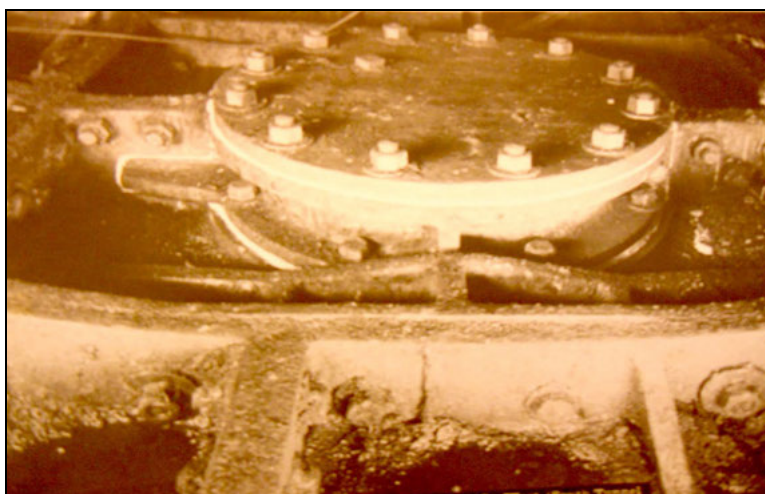
Figure 6. “Bore segment” with cover after decision was made not to install screw piles (Forgie personal papers, Smithsonian Institution)
