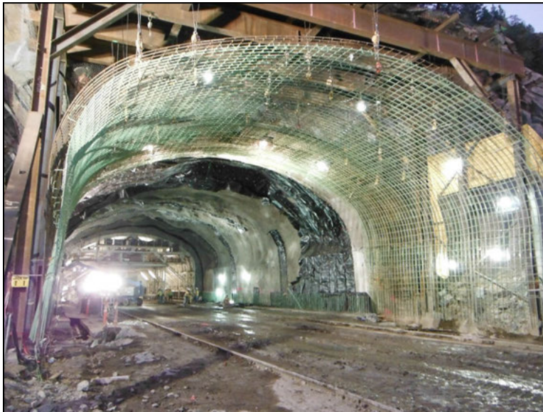
Figure 6. Rebar cage waiting to be lowered onto form
