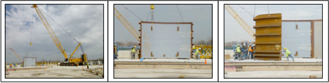
Figure 13. Assembly of sections
