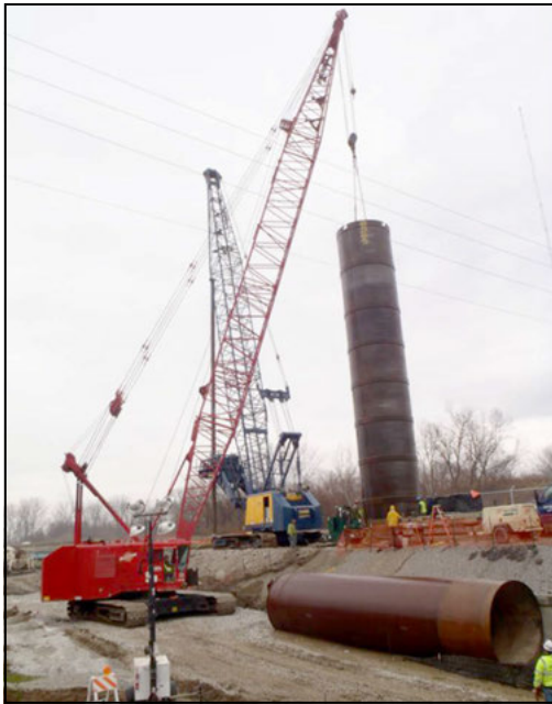
Figure 4. Case foundation placing permanent casing into excavation at Utility Shaft #3
