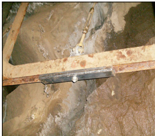
Figure 3. Shaft turnbuckle temporary support
