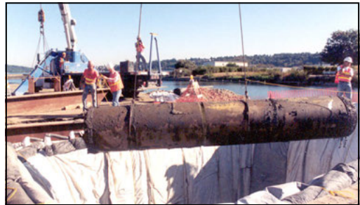
Figure 7. Removal of MTBM from shaft with no dewatering
