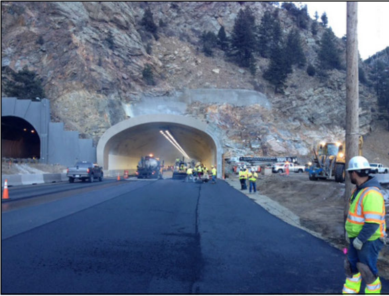
Figure 9. Final paving and tunnel entrance
