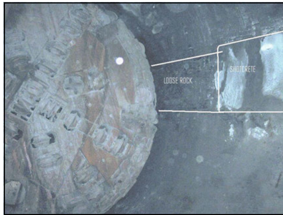
Figure 5. SELI TBM with location of poor quality rock at springline identified
