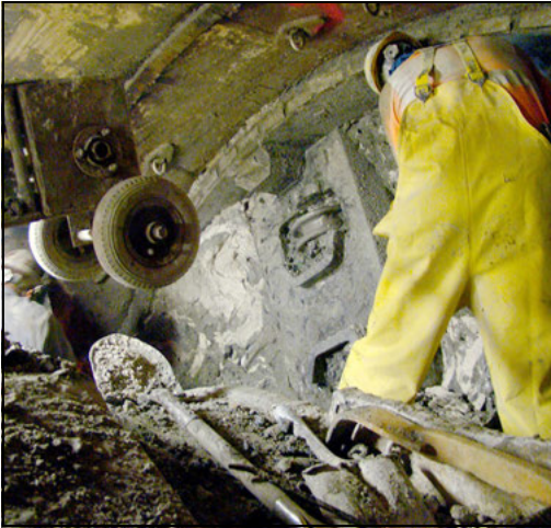
Figure 11. Removing cutter head near frozen soil
