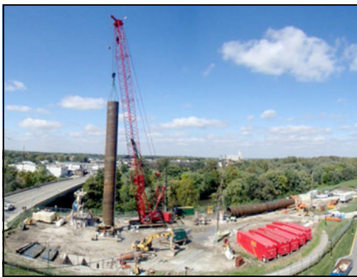
Figure 15. Typical shaft installation
