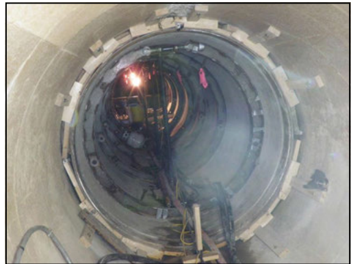
Figure 12. Temporary steel ribs used to stiffen steel pipes during grout placement
