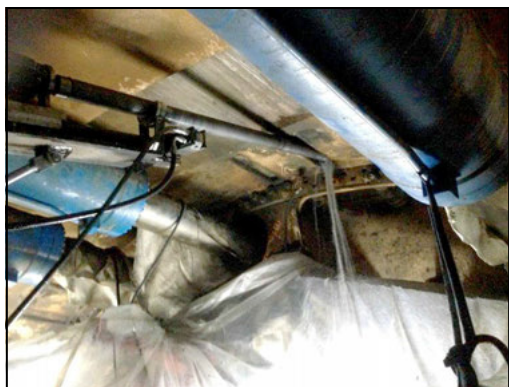
Figure 5. Canopy tube drilling
