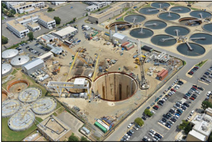
Figure 4. Blue Plains dewatering and screening shaft site
