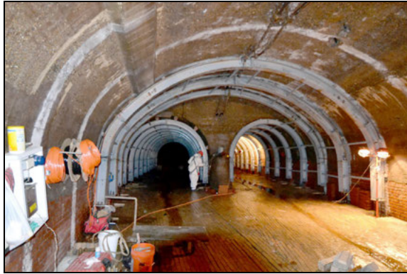
Figure 9. Steel ribs being installed in the Tiber Creek sewer
