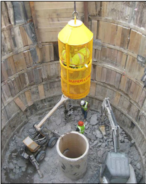
Figure 10. 25th Street shaft demolition
