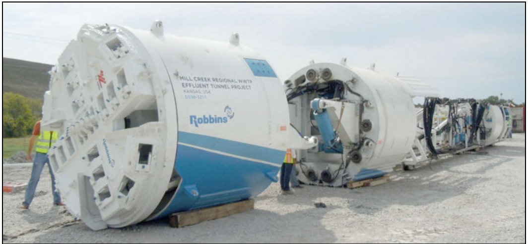
Figure 9. TBM above ground during pre-assembly at down shaft site
