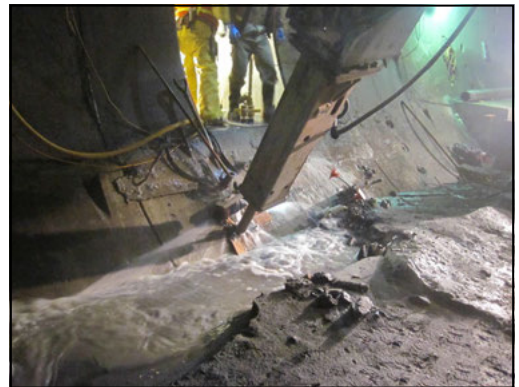
Figure 7. Groundwater inflow encountered during well abandonment
