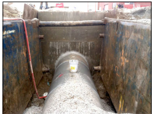
Figure 9. 1372 mm (54 in) diameter connection to WR06-DV-1
