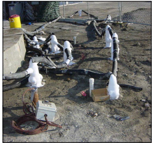
Figure 3. Extra freeze pipes in operation
