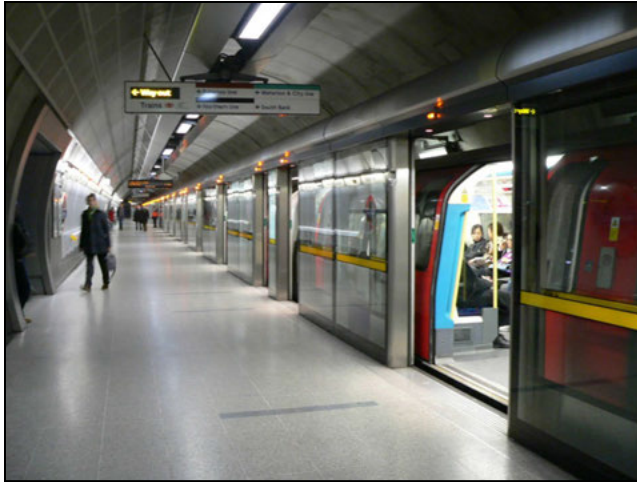
Figure 2. Platform edge doors in underground station
