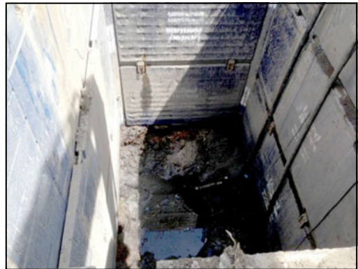
Figure 9. Excavation support system
