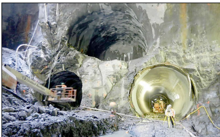
Figure 9. Excavation and geometry—CIR adit and TBM tunnels at South Open Cut
