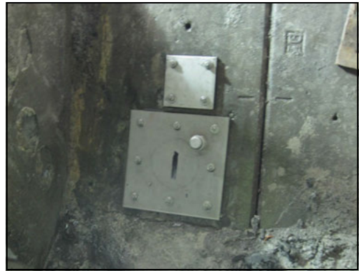
Figure 9. Well point 1 with final stainless-steel plates
