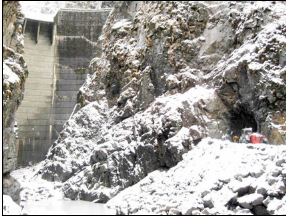
Figure 2. Drainage tunnel portal location
