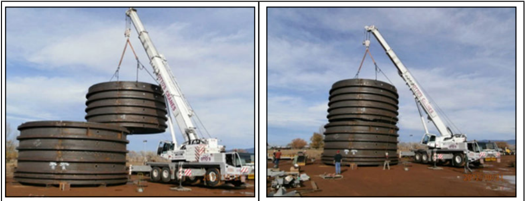
Figure 12. Preassembly of sections
