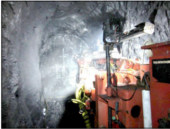
Figure 3. Drilling in intake tunnel
