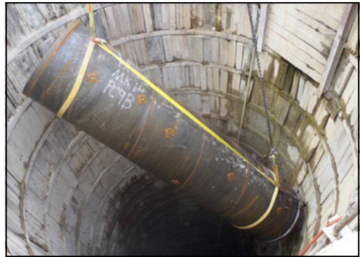
Figure 11. Lowering steel pipe into 25th Street shaft
