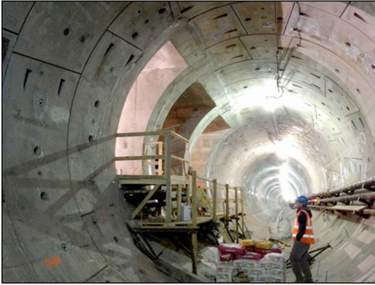
Figure 14. Finished cross passages—View from the TBM tunnel
