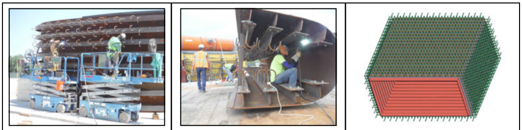
Figure 18. "J" anchor welding and anchor layout
