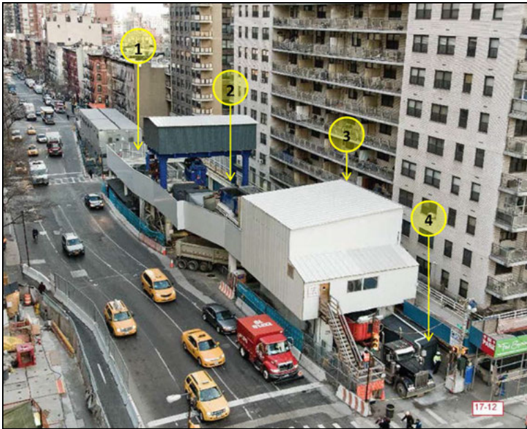
Figure 5. 86th Street station mucking system
