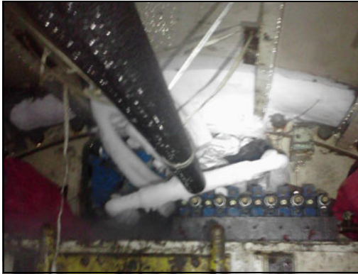
Figure 19. LN lines freeing ceiling of TBM
