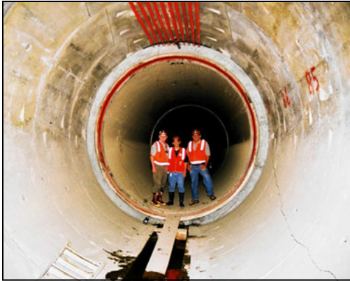
Photo 7: Initial gasketed bolted precast segmental liner and final carrier pipe liner. East Central Interceptor portion of North Outfall Sewer. (Courtesy of J. Critchfield)
