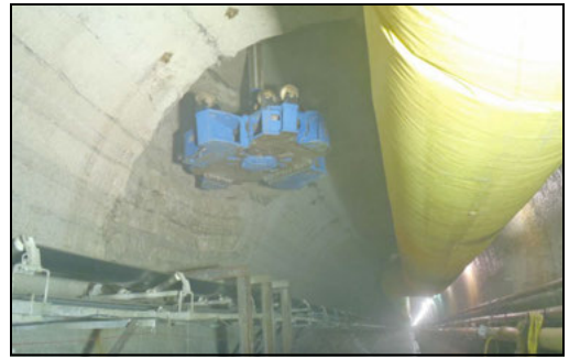
Figure 5. Raise bore reamer, as seen in the tunnel
