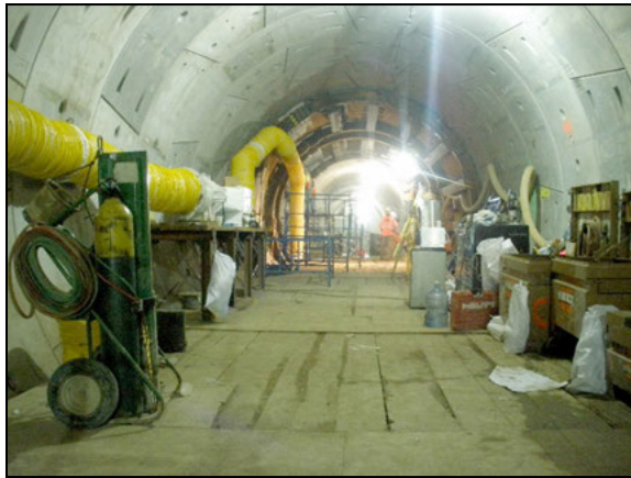
Figure 8. Temporary working deck at the cross-passage location
