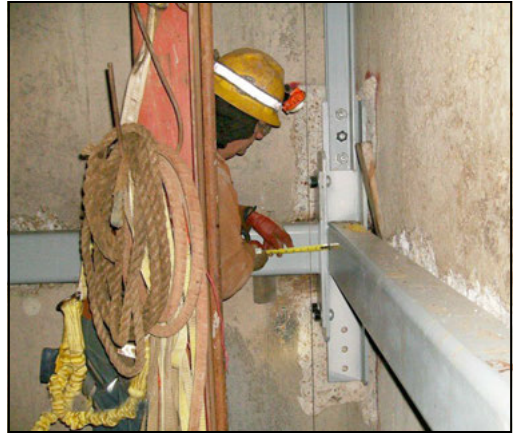
Figure 7. Shaft alignment measurements
