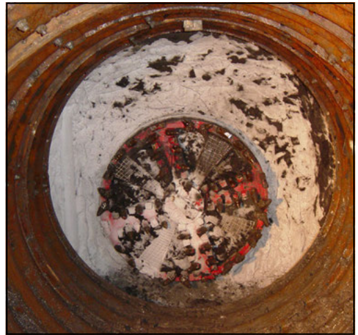
Figure 4. MTBM face encased in frozen soil
