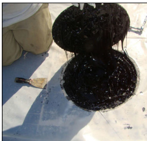
Figure 4. Top of monitoring well—asphalt filled
