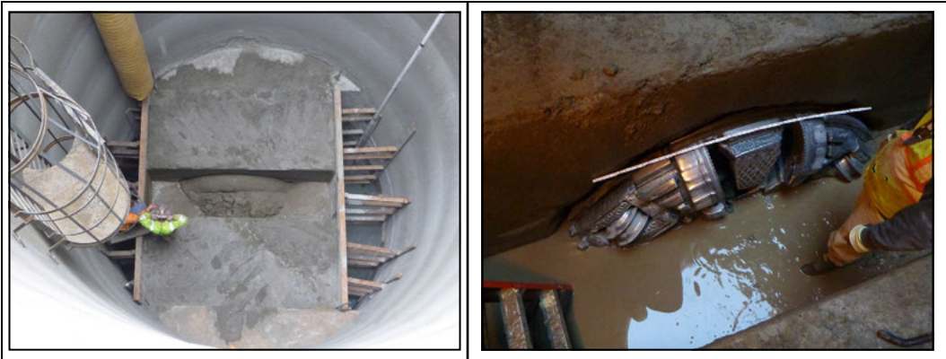
Figure 1. SARI “push-thru” intermediate shaft for MTBM inspection
