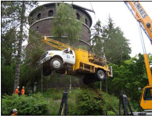
Figure 6. Crane lifting drill rig into place
