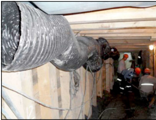
Figure 3. Bypass tunnel excavation
