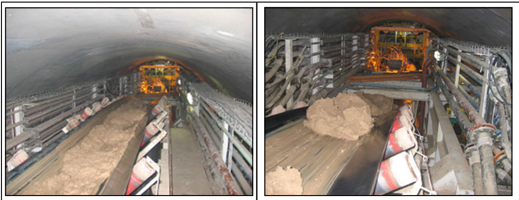
Figure 3. Silty clay prior to and following GC treatment (Photo courtesy of Condat)
