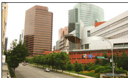
Figure 4. Existing buildings, north of NE 4th Street
