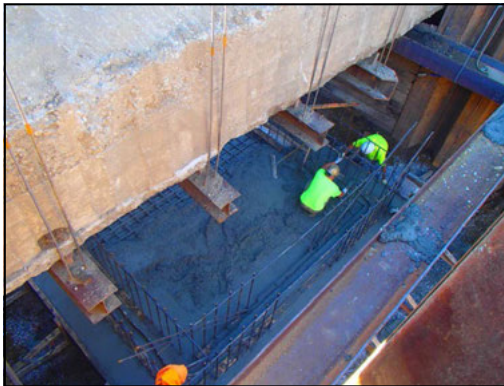
Figure 6. Typical large diversion structure base slab
