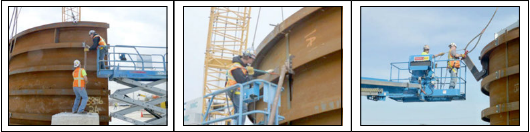
Figure 14. Rigging and connections
