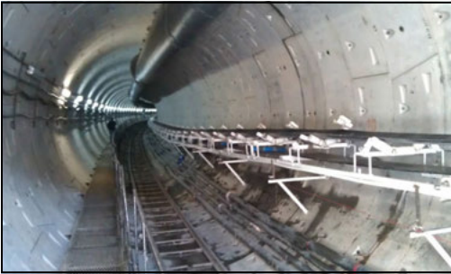
Figure 8. Horizontal conveyors going around a curve
