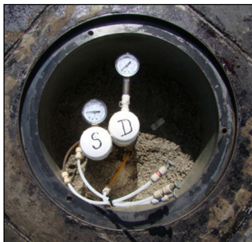
Figure 5. Cleaned-up monitoring well
