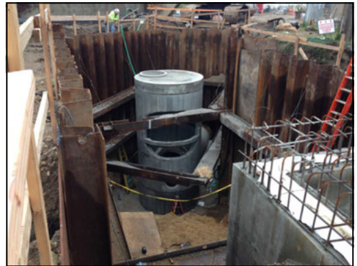
Figure 8. Typical large diameter manhole installation
