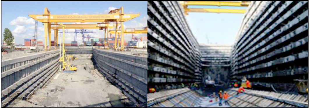
Figure 6. Asia transition box—TBM launch shaft
