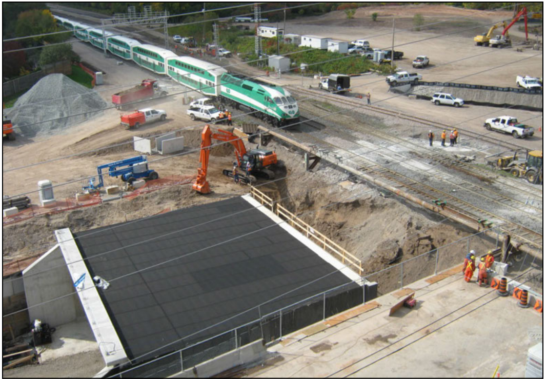
Figure 4. Underpass structure completed prior to the jacking operation
