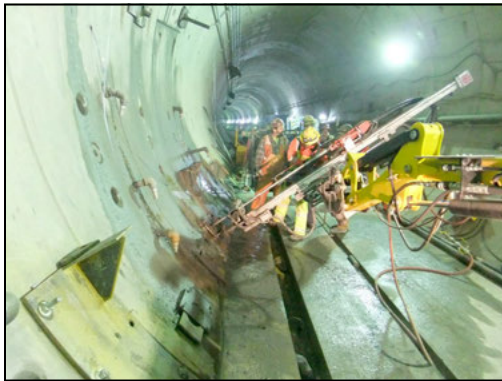
Figure 3. Drilling and installation of drain pipes at cross passage
