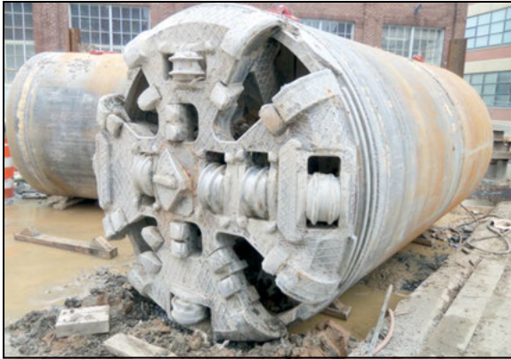
Figure 6. “Go Yard” after completing the Tingey Street Diversion Sewer tunnel drive
