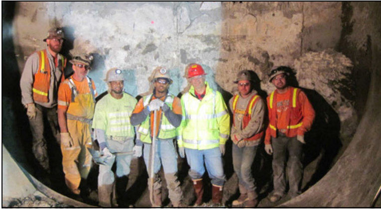
Figure 6. Completion of excavation and initial ground support for Cross Passage 17
