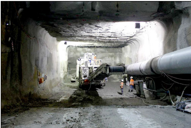
Figure 4. View into the Forecourt Tunnel during full-face roadheader excavation
