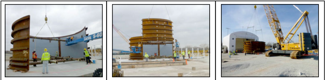
Figure 15. Bracing subassembly and shelter
