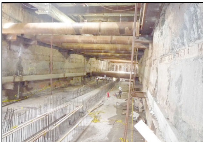
Figure 6. North end of station
