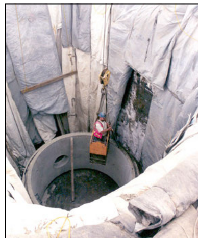
Figure 8. Installing concrete manhole inside frozen shoring
