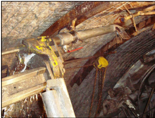
Figure 8. Drilling through stand pipe at Parbati
