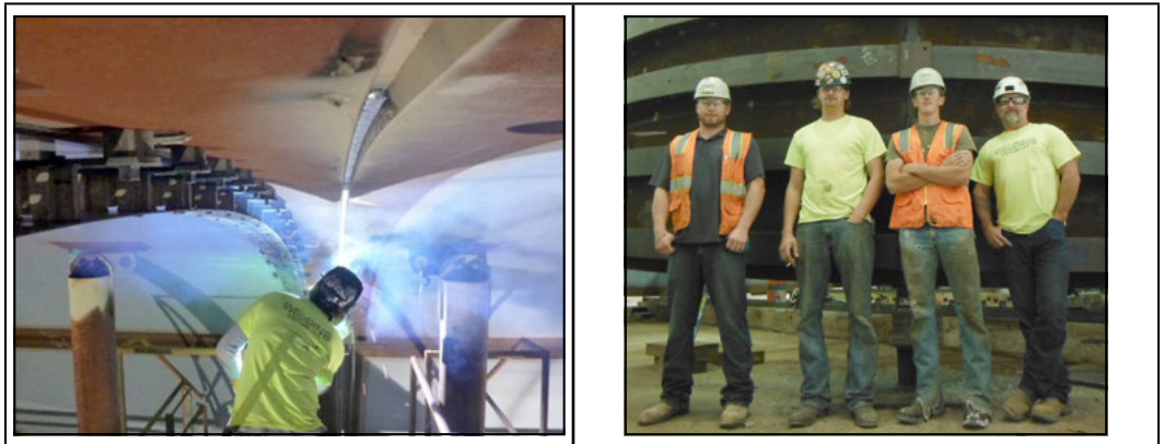
Figure 24. Circumferential seam welding and technical welding team
