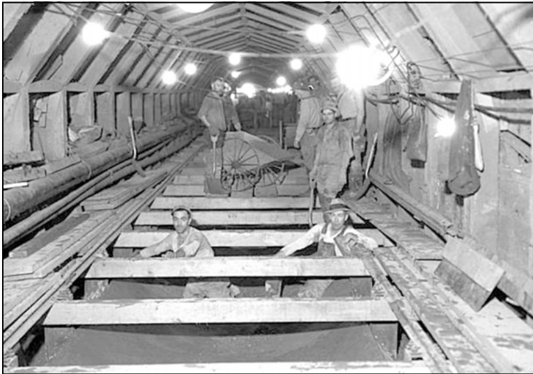
Figure 2. Existing Irvington Tunnel
