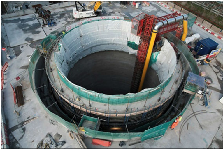
Figure 7. Slipformed construction of secondary lining
