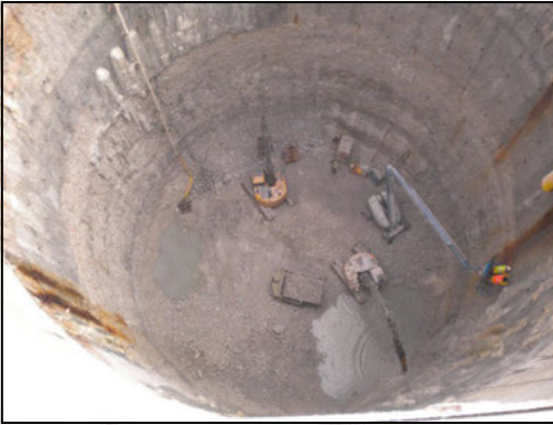
Figure 5. Main gate shaft during excavation
