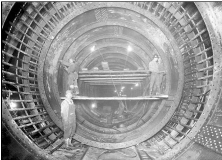
Figure 3. Steel-concrete interliner used in RWBT Roseton and Wawarsing areas
