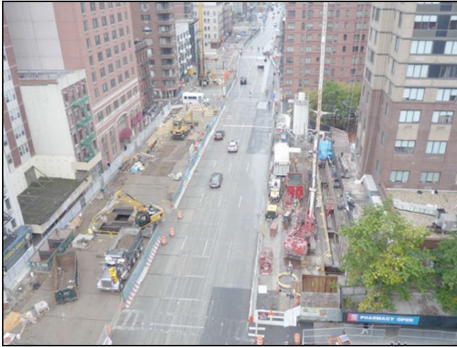
Figure 8. Street view of work zone and travel lanes
