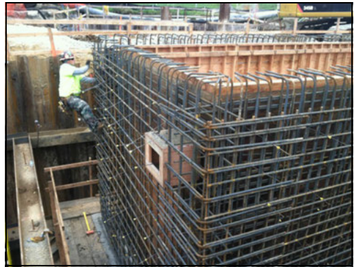
Figure 12. Typical screen and gate structure
