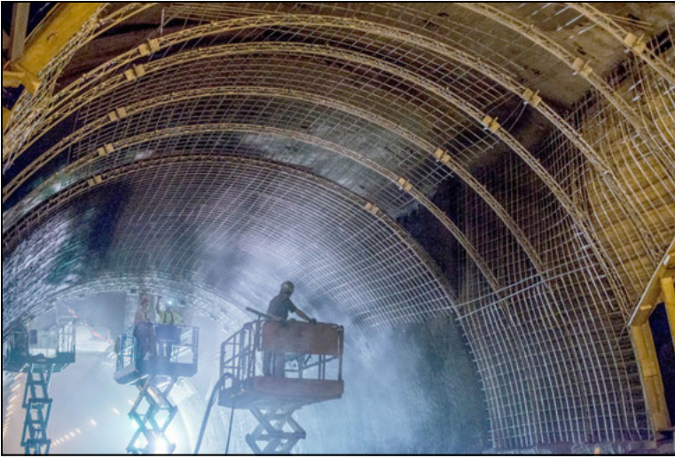
Figure 9. Construction sequence Step 5—preparation of center arch section
