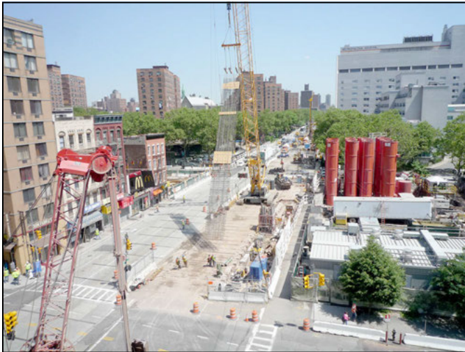
Figure 9. Installation of slurry wall reinforcing cage
