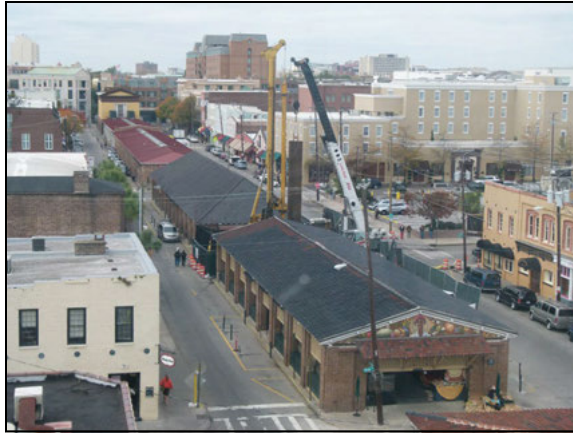
Figure 5. Drop shaft installation along Market Street
