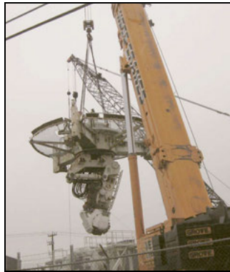
Figure 6. Lowering the vertical shaft machine into the shaft liner
