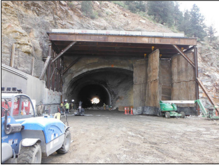
Figure 5. Structural steel framed canopy with blast mats attached
