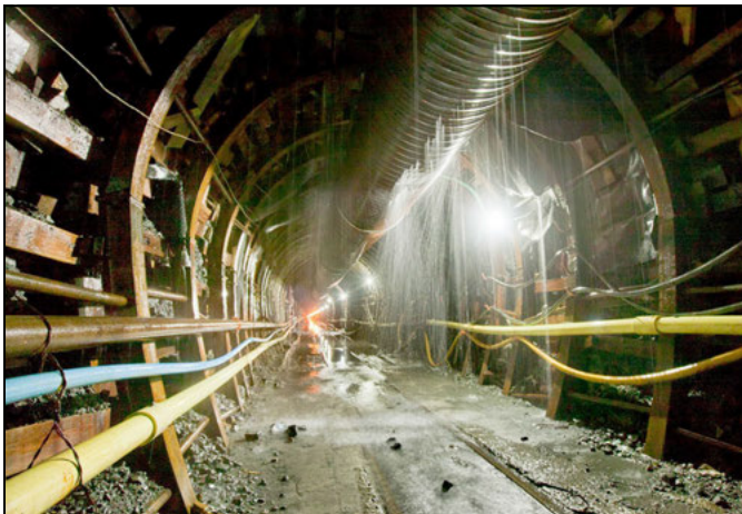
Figure 7. Tunnel heading in zone of high water inflow
