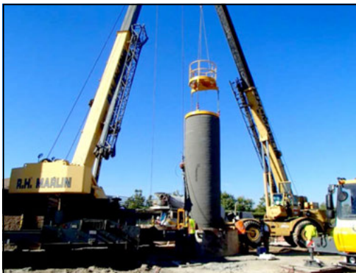
Figure 7. Typical drop shaft final liner
