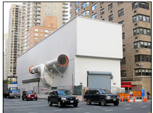
Figure 12. Operational Muck House at 72nd Street site. Ventilation and electrical systems are also enclosed.
