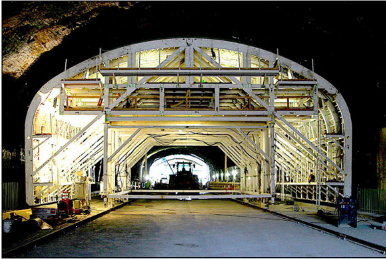
Figure 7. Concrete form in tunnel
