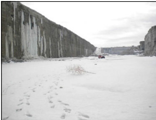
Figure 3. McCook Reservoir and limestone quarry
