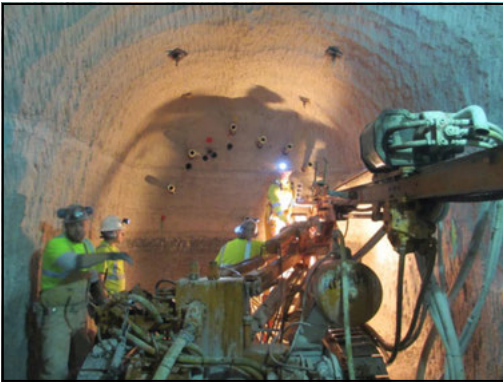
Figure 11. Probing operations
