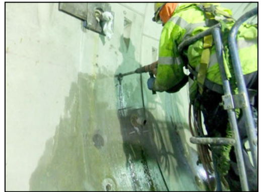
Figure 4. Installation of piezometer with electric rotary hammer drill
