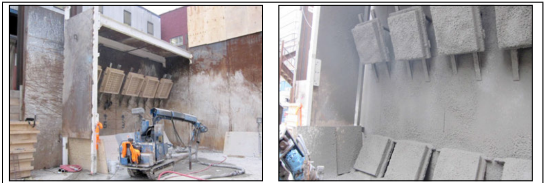
Figure 2. Test panels before and after shotcrete application
