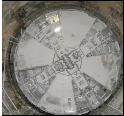
Figure 12. BT4 successfully mined inside BT3
