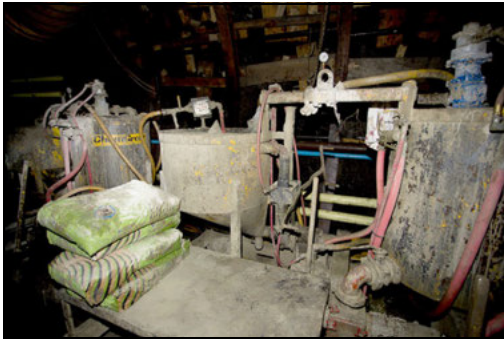
Figure 8. Pre-excitation grout plant in heading
