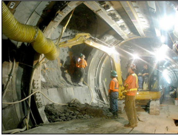
Figure 7. Tunnel liner bracing and start-up of excavation for drift 1
