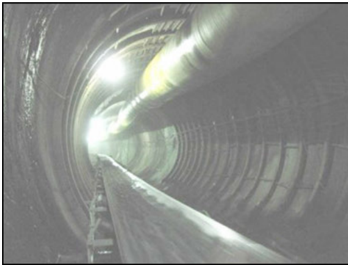
Figure 3. Full circumference ring sets to be removed for TBM back-up
