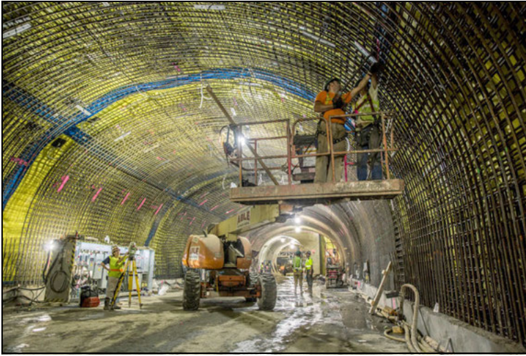
Figure 9. Photograph of welded mat reinforcement installed in the G4/S2 turnout cavern
