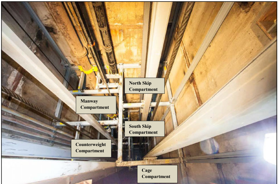
Figure 5. Typical sets installation looking down the shaft (photo by Steve Babbit)
