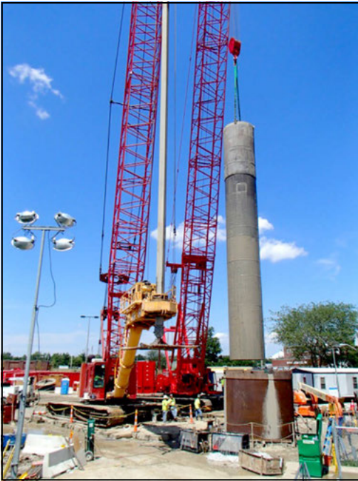
Figure 23. Float can installation
