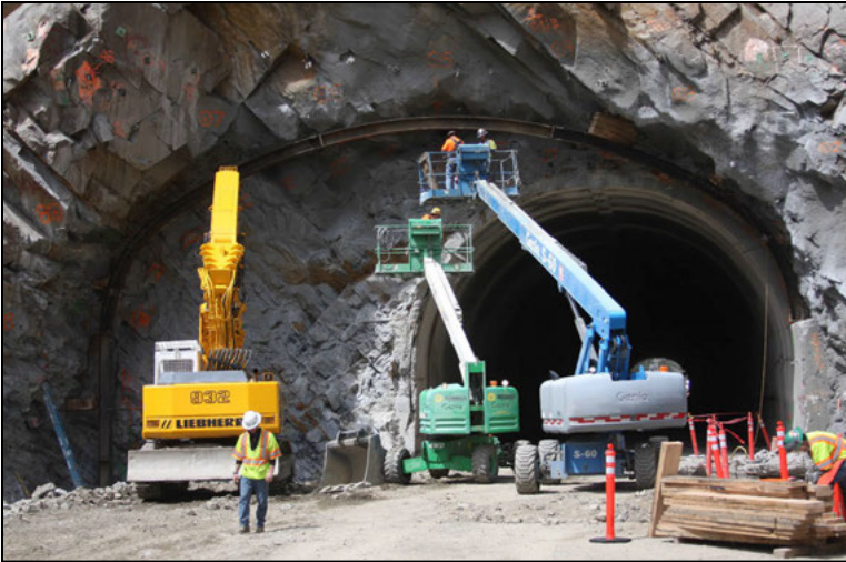
Figure 3. Portal development on east side
