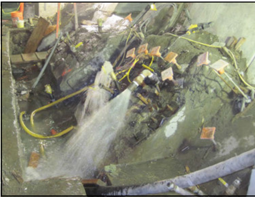
Figure 8. View of bolted shotcrete and grout ports
