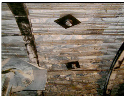
Figure 8. Loose rock held in place by McNally system
