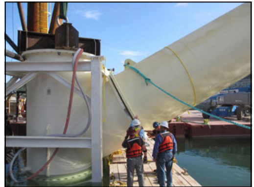
Figure 8. Assembly of intake piping
