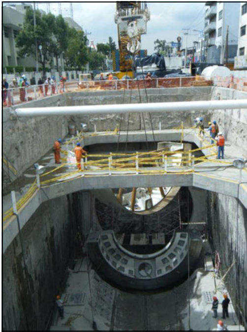
Figure 1. Lowering of machine shield sections, MX12 Line, Mexico City, Mexico
