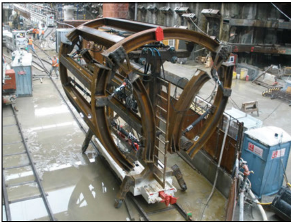
Figure 6. Foldable frame for bracing of the tunnel segmental lining
