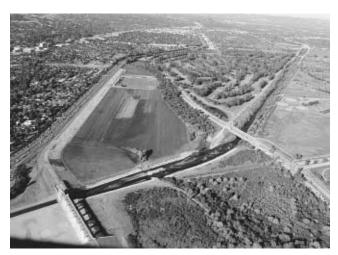
Sepulveda Dam and Flood Control Basin, San Fernando Valley, County of Los Angeles. Too much water can also be a problem. Heavy winter rains cause catastrophic flash flooding. The 710-foot high Sepulveda Dam (left foreground) was completed in 1941 to protect downstream cities in L.A. County. It permits the 1,335-acre basin to be flooded during sustained downpours. Photograph by Michael J. Dear.
