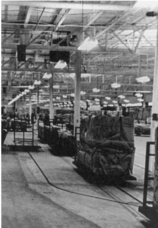
Figure 14 In-floor Tow-Line Conveyor.
