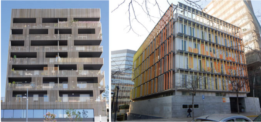
Fig. 8.3 Images of shadings in residential buildings, whose design and use is very common and appreciated in the Mediterranean Region. Montpellier (France) and Barcelona (Spain)
