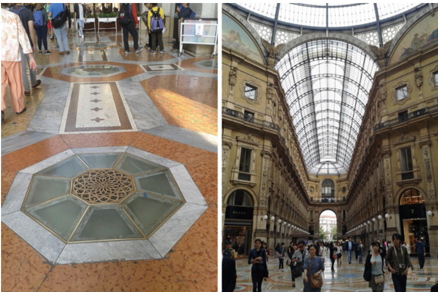
Fig. 7.20 Conditioning of semi-exterior spaces. Vents introduce cool air from the basement. Galleria Vittorio Emanuele II. Milan (Italy)
