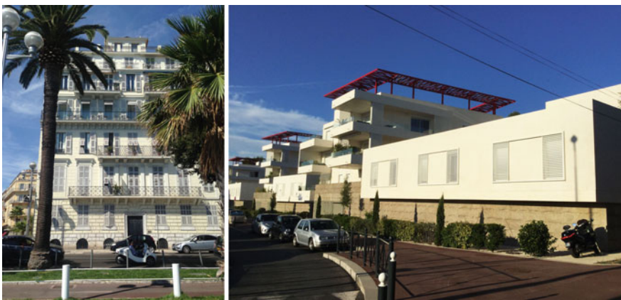
Fig. 3.12 Illustrative images of Southern European buildings with passive strategies. Nice and Montpellier (France)
