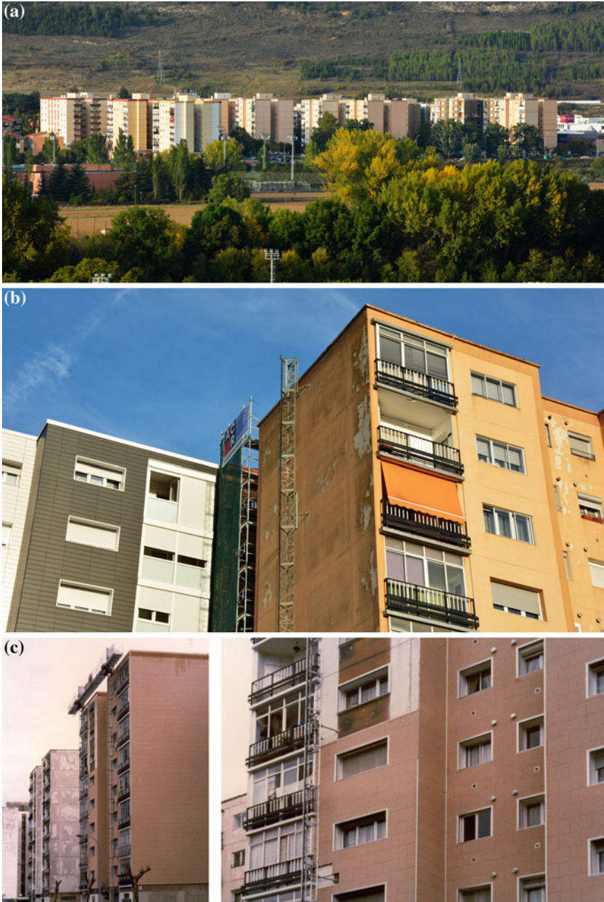
Fig. 5.9 Photographs of ORVINA group in Chantrea, a panoramic view, b building renovation example and c ORVINA case study
