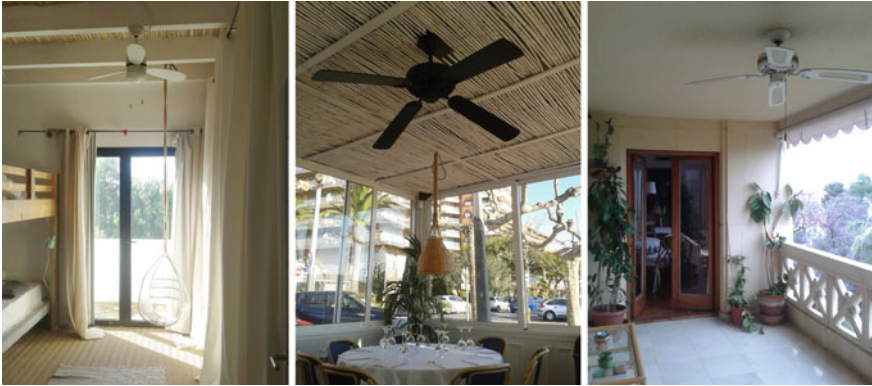
Fig. 3.9 The use of fans in the ceiling to condition indoor spaces and even semi-exterior (porch and terrace) is a well-established and valued measure in the Mediterranean
