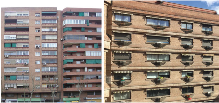
Fig. 3.13 Installation of air conditioning systems anywhere on the façade and integrated. Examples in Barcelona and Madrid (Spain)
