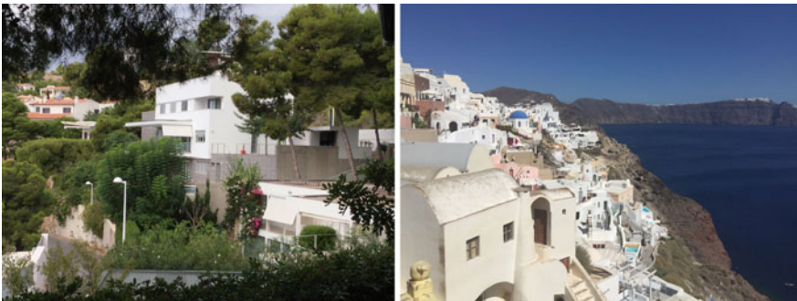
Fig. 1.3 Examples of new and traditional passive architecture in Southern Europe. Oropesa del Mar (Spain) and Santorini (Greece)
