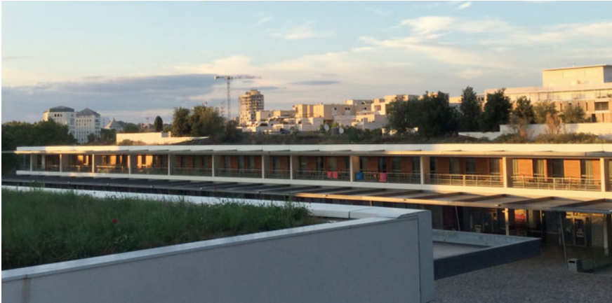
Fig. 7.23 Illustrative images of passive measures in the Mediterranean area: green roofs, canopies, movable shading, etc. Montpellier (France)
