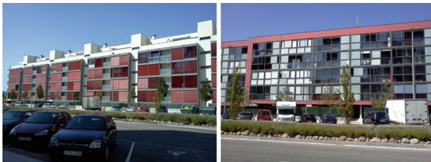
Fig. 7.11 Images of bioclimatic buildings with sunspaces in Sarriguren Ecocity near Pamplona (Spain), with and without shading devices in the buildings
