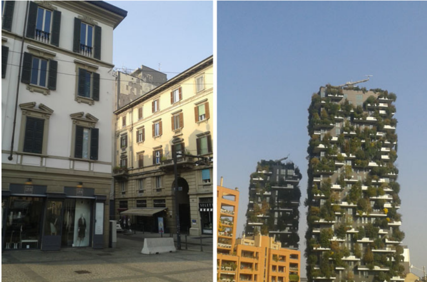
Fig. 8.25 Example of passive energy strategies Milan (Italy) Movable shading and green facades in high rise buildings
