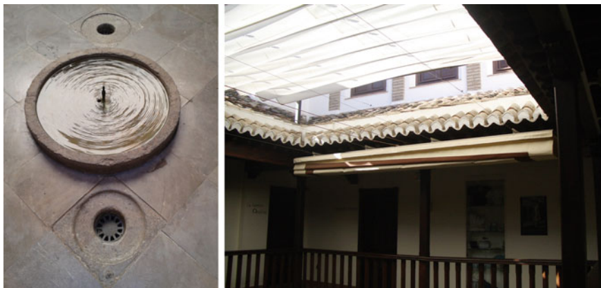
Fig. 7.16 Examples of traditional Andalusian patio. Shading and evaporative cooling in Granada (Spain)
