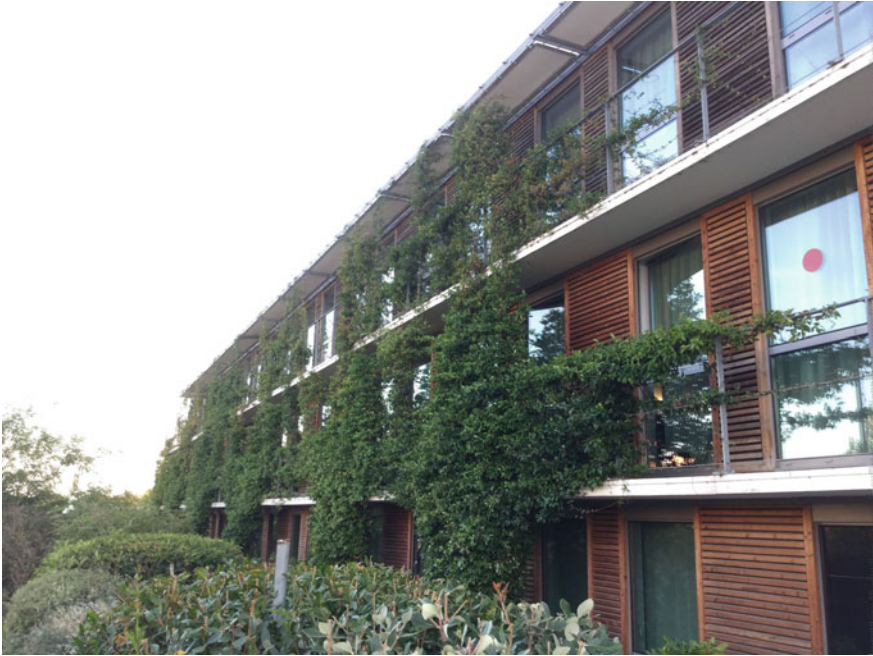
Fig. 7.21 Illustrative images of different types of shading: vegetation, overhangs, shutters, etc. Montpellier (France)
