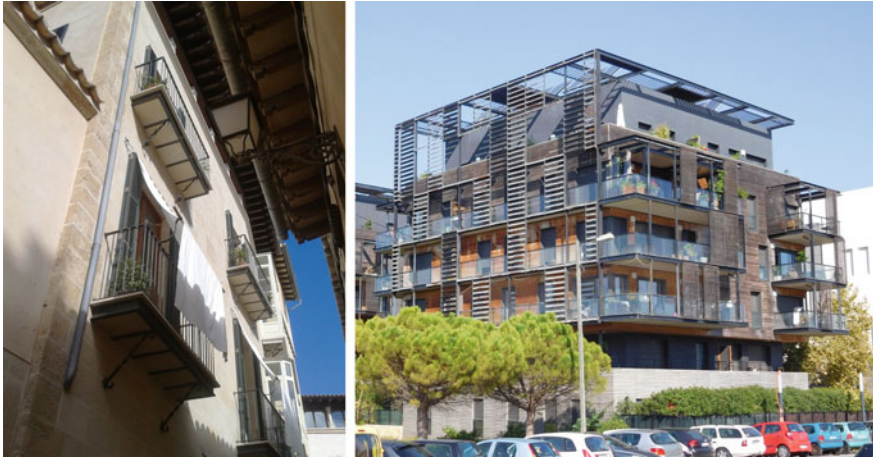
Fig. 8.11 Examples of shading in the Mediterranean from traditional (Palma, Spain) to new designs (Montpellier, France)
