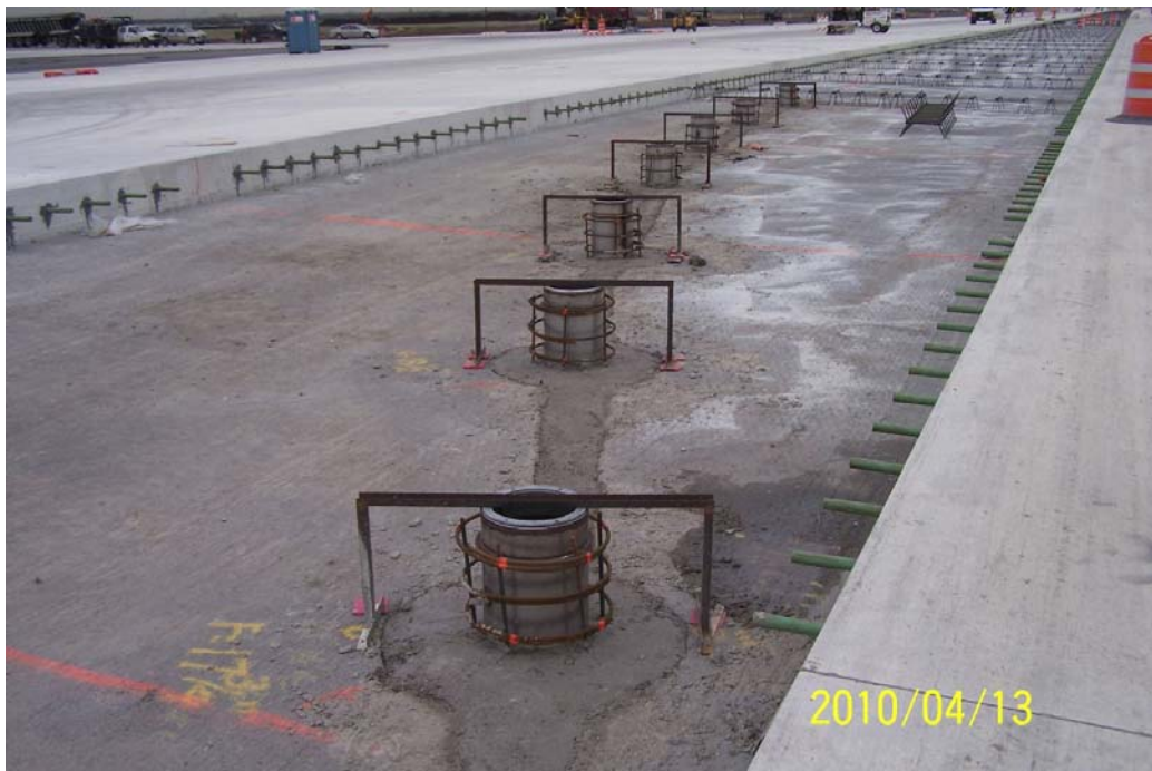
Figure 3- Reinforcing Cage around Light Can
