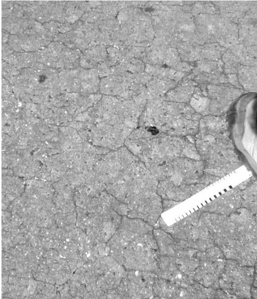
Figure 1. Map cracking in a concrete pavement
