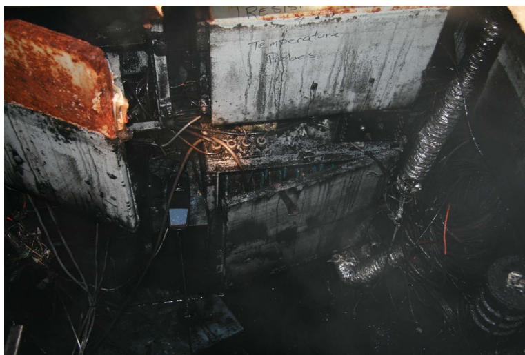
Figure 4. Condition of FAA Instrumentation Vault at DIA
