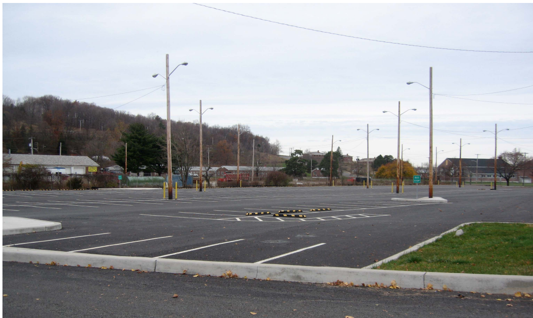
Figure 3: Permeable Asphalt at the Stewart International Airport, Orange County, New York
