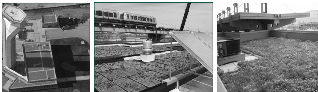
Figure 2: ORD North Airport Traffic Control Tower, ORD Aircraft Rescue and Firefighting Facility #3, and the MDW Electrical Vault Vegetated Roofs (pictured left to right)
