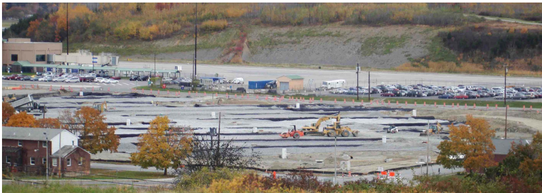
Figure 5: Construction of the Terraces and Berms. The dark lines are the berms covered with geotextile fabric.
