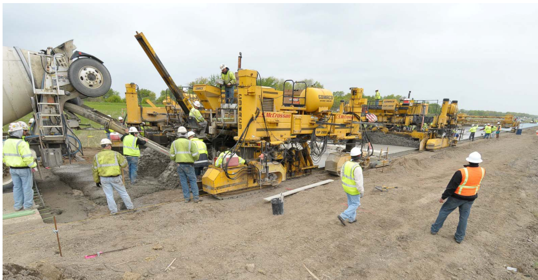
Figure 3. 2010 Composite Pavement Construction, Wet on Wet Concrete
