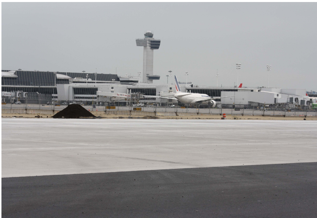
Figure 2: Concrete Pavement on Runway 13R-31L John F. Kennedy International Airport
