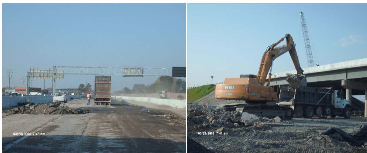
Figure 1(a). During JRCP Pavement breaking (b) JRCP Pavement removing
