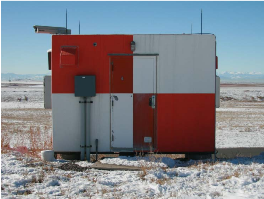
Figure 2. FAA Instrumentation Shelter with Video Camera at DIA
