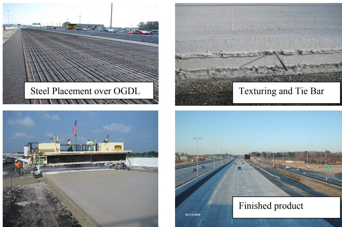
Figure 2. I-64 Battlefield Blvd Project construction
