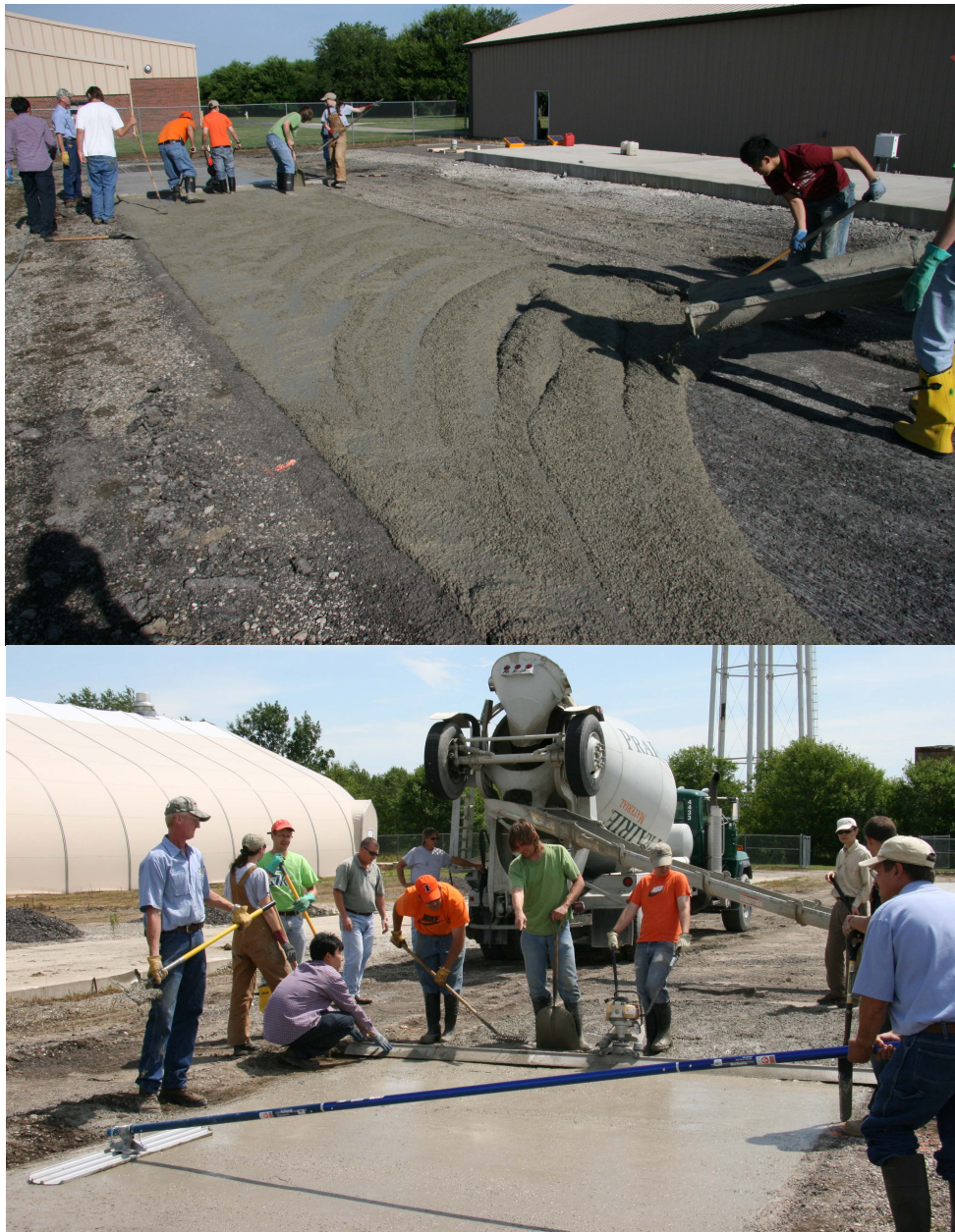
Figure 3. Photographs from construction of the FFC inlay.
