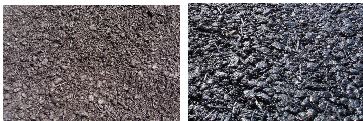
Figure 2. Close-up of the fiber-reinforced HMA
