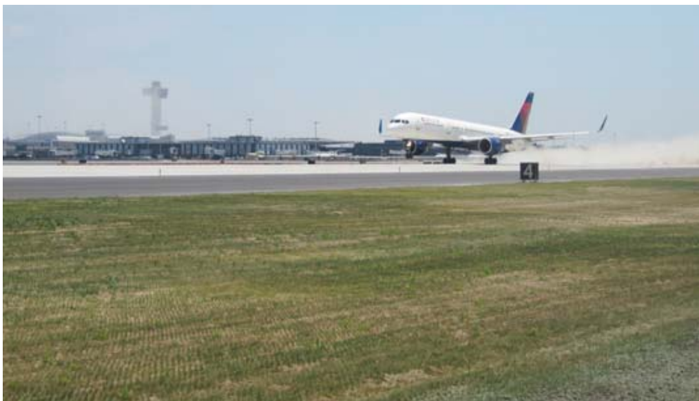
Figure 4- Stage I Completed and Runway Reopened
