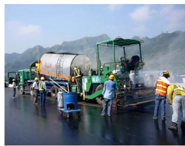
Figure 14. Application of Guss mix.
