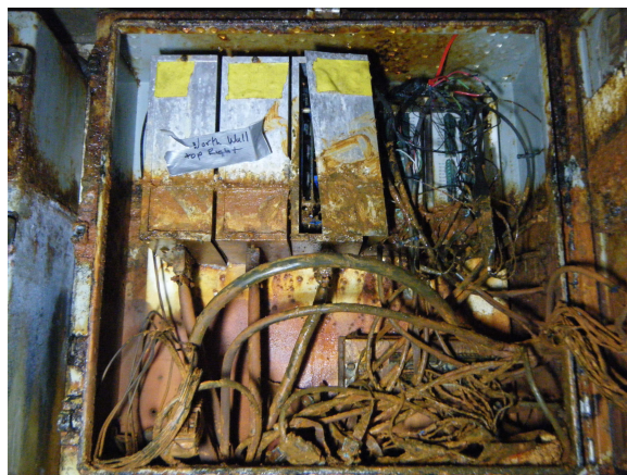
Figure 5. Condition of Data Acquisition System at DIA
