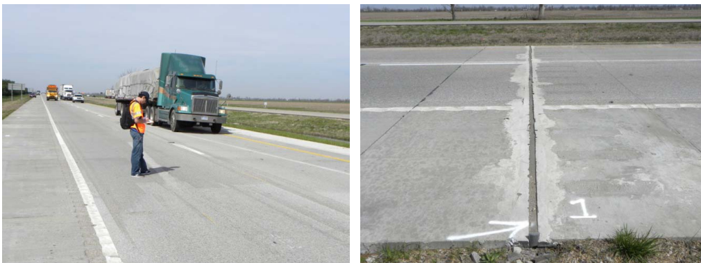
Figure 4: I-57 PPCP views (right photo shows reconstructed expansion joint)
