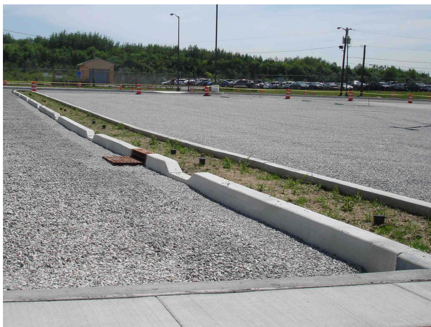
Figure 2: Parking Lot Islands, Stone Sub-base with Choker Course, Prior to Placement of Open-Graded Asphalt Concrete Top Course
