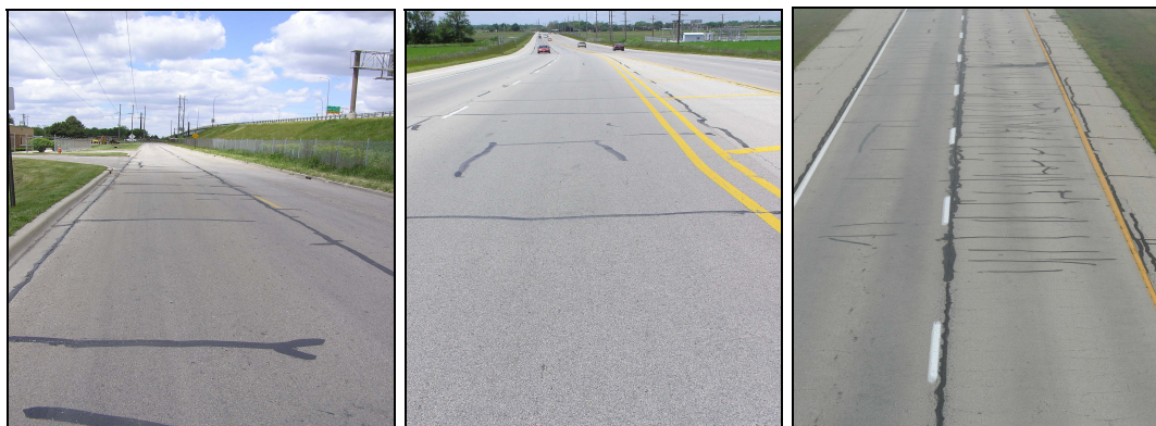
Figure 1. Thermal cracking in asphalt concrete pavements.
