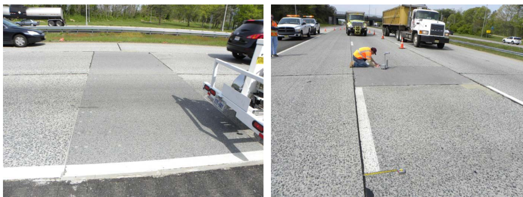
Figure 7: Views of the I-295 precast panels
