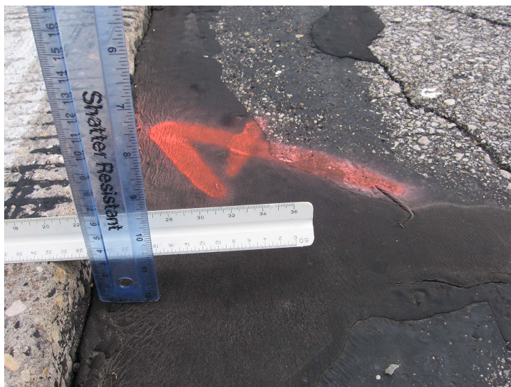
Figure 4. Lane to shoulder drop off in test section of RCA/5 (I-35 in Hamilton county mile post 131.40 to 131.45).
