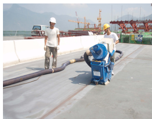
(a) shot blasting
