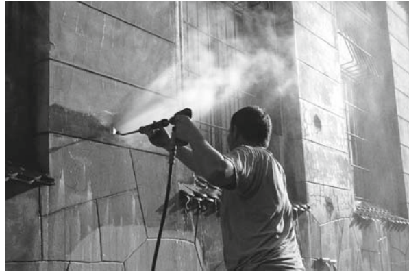
Fig. 14.11 Stripping existing modern masonry paint with the use of superheated water
