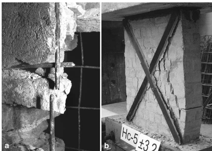
Fig. 17.5 Strengthening of brick-masonry walls by coating: a tensile rupture of reinforcing bar indicates the flexural failure mechanism of the strengthened wall and b delamination of diagonally placed CFRP laminate strips at shear failure
